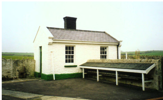
Fig. 11 Workshop at Nash Point Lighthouse. Now an engine room.
