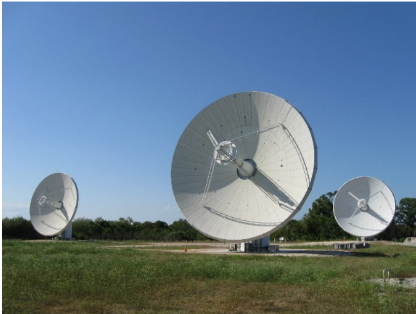
Fig. 2. Current array configuration of three 12m reflector antennas at the Kennedy Space Center
