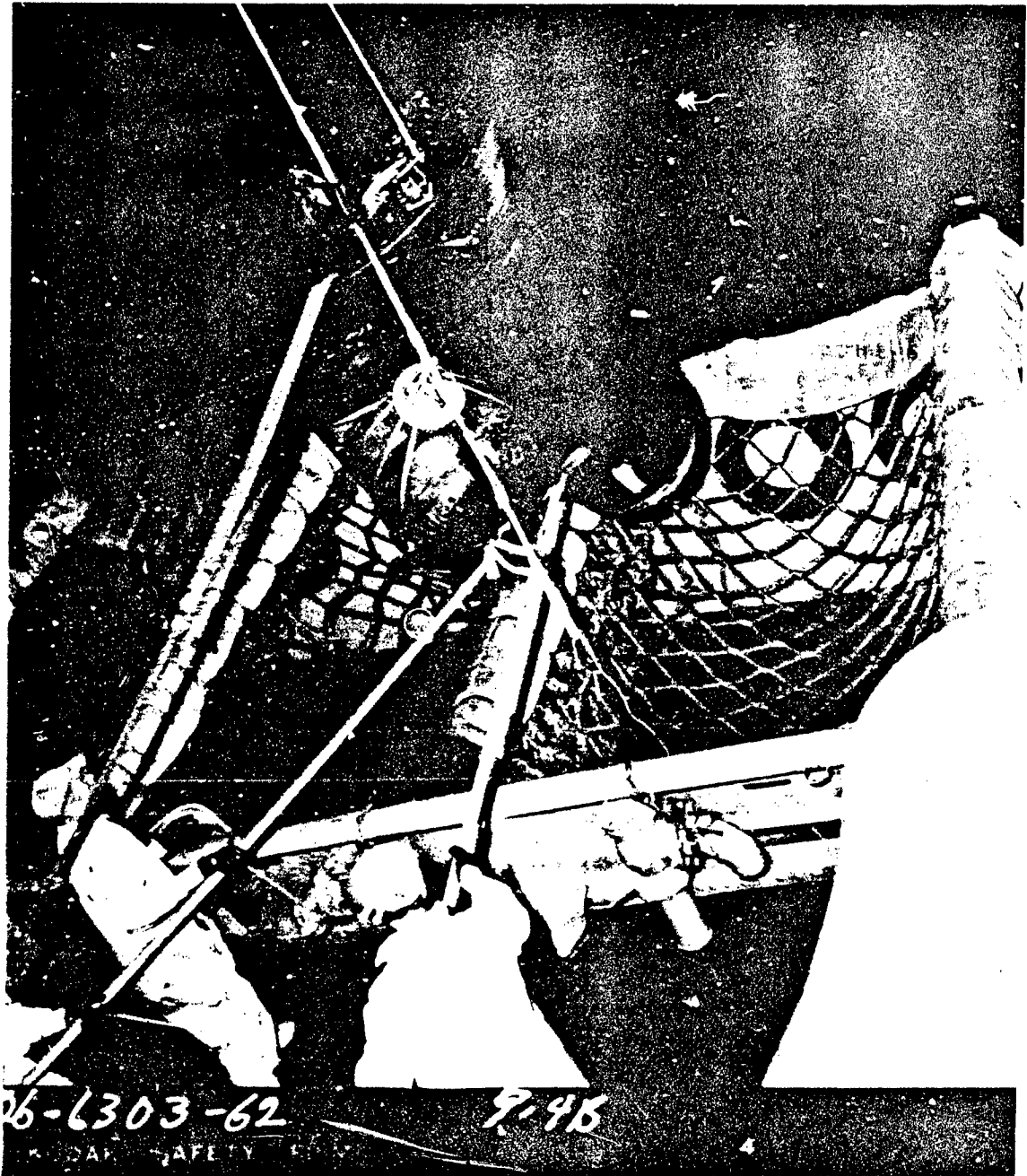
Figure 29. Radioactive pod with flotation bag still attached is guided into sling in M-boat following DOMINIC shot.
