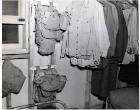
**Figure 7:** New metal bed frames with modifications to allow stacking (top), and simple devices for hanging field gear on walls (bottom).
