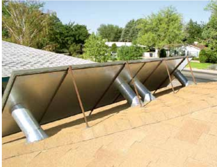
Figure 15. Roof-mounted solar collector.
