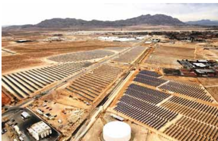
Figure 2. A 14-MWp PV system at Nellis AFB, NV.
