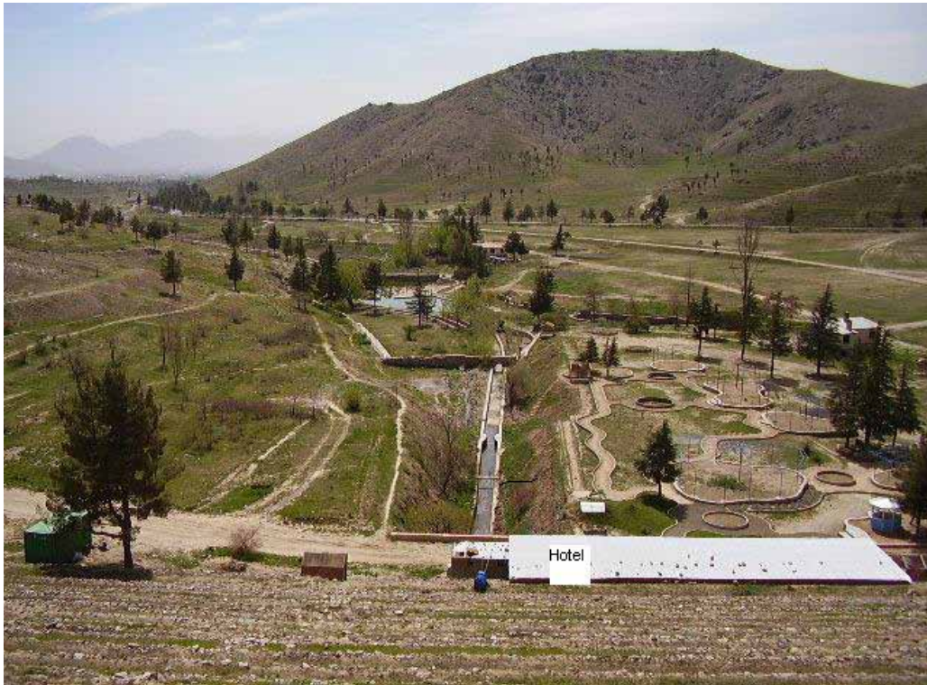
Figure B1. Terrain downstream of Qargha Dam.
