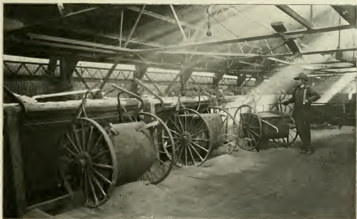
HOPPERS. Dumping roasted calcines into smelting furnace.
