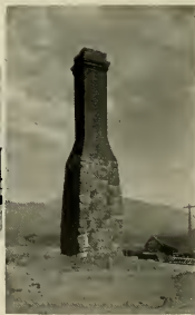
Stack of Centennial Smelter.
