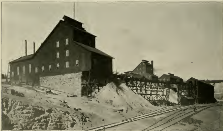
MOUNTAIN CONSOLIDATED. NO. 2.
