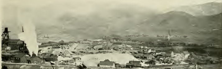
LOOKING EAST FROM MEADERVILLE. Showing extension of operations across valley toward Rockies.
