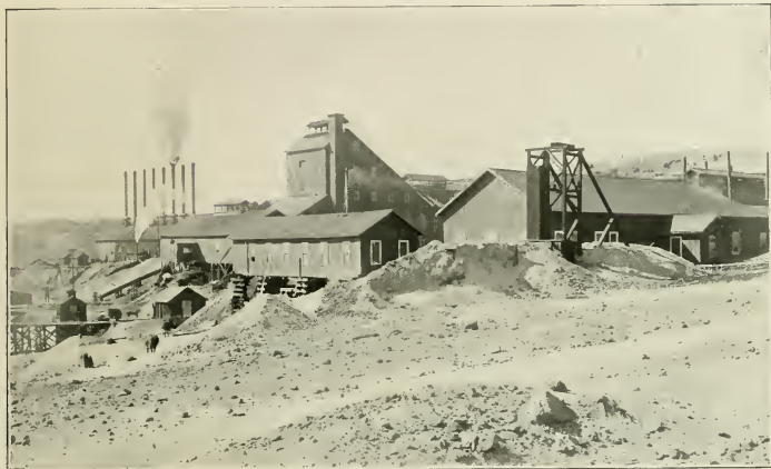
MOUNTAIN CONSOLIDATED, No. 1.
