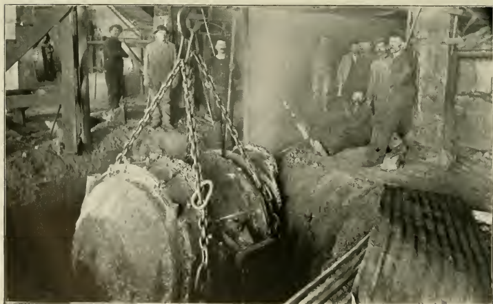
PREPARING TO FILL CONVERTER WITH CHARGE OF MATTE.
