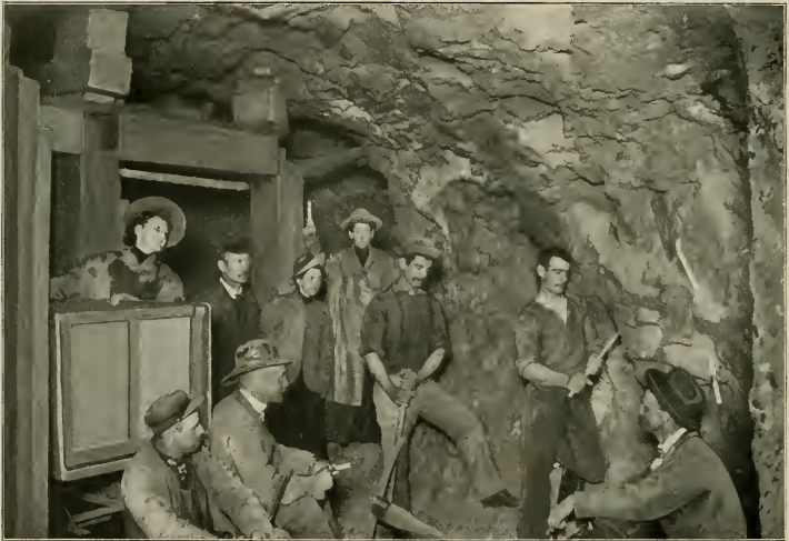
HAND DRILLING. 1,200-foot level, Parrot Mine.
