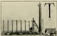
STEEL STACK 112 FEET HIGH.
