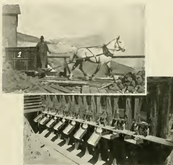
CARRYING ORE TO THE BIN.
