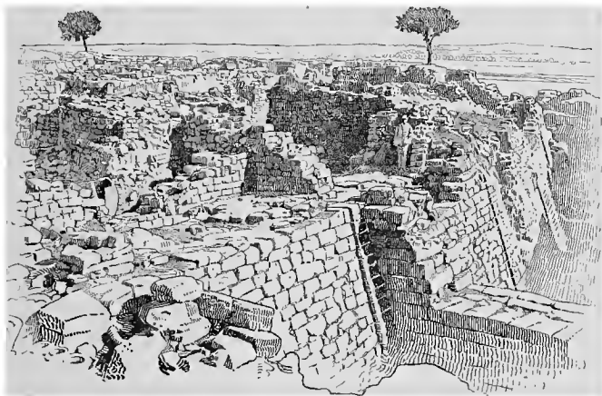
FIG. 151. THE WALLS OF HOMERIC TROY (BUILT ABOUT 1500 B.C.)
