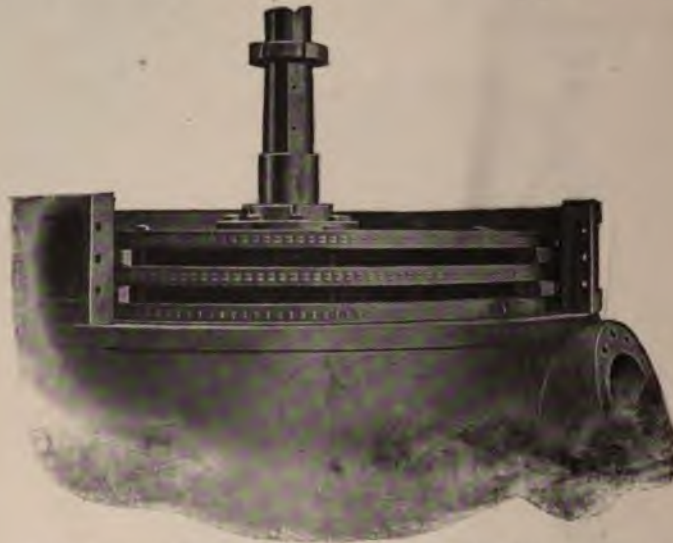
500 KW CURTIS' STEAM TURBINE IN COURSE OF CONSTRUCTION.
