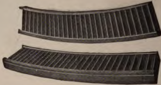
STATIONARY BUCKETS FOR CURTIS STEAM TURBINE.
