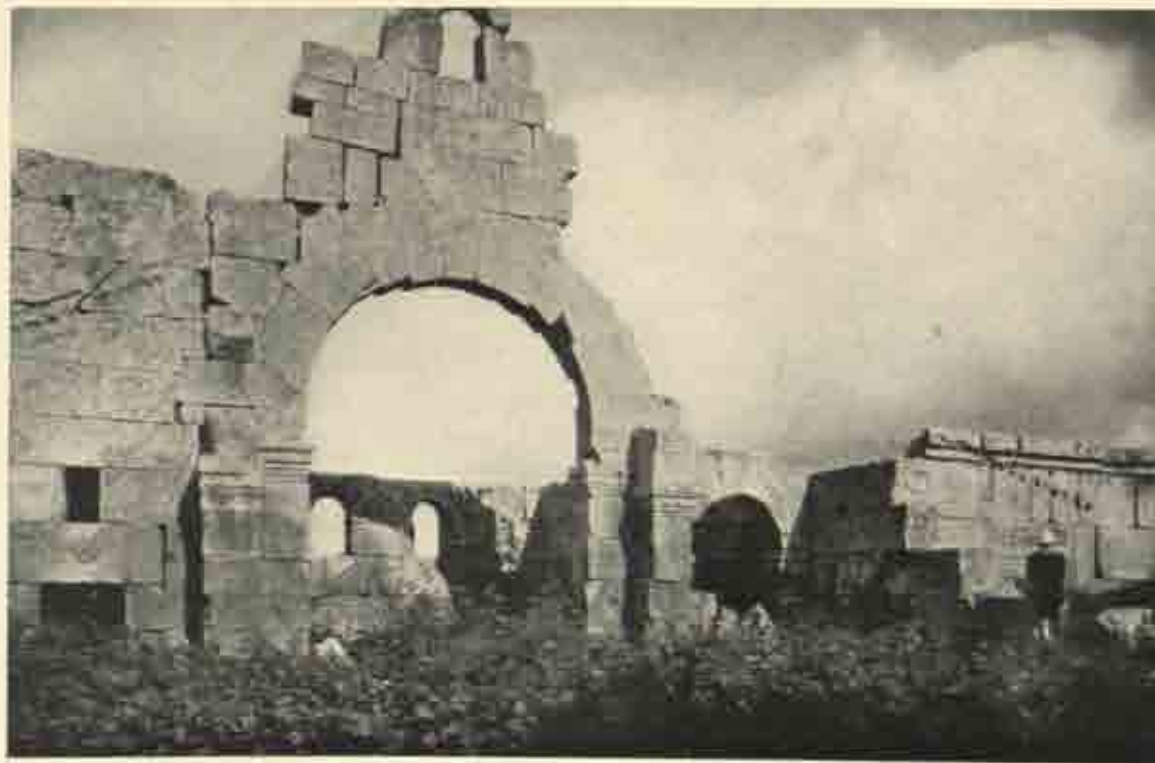
Interior of Church of St. Sergius, at Dār Kītā, looking southeast.
