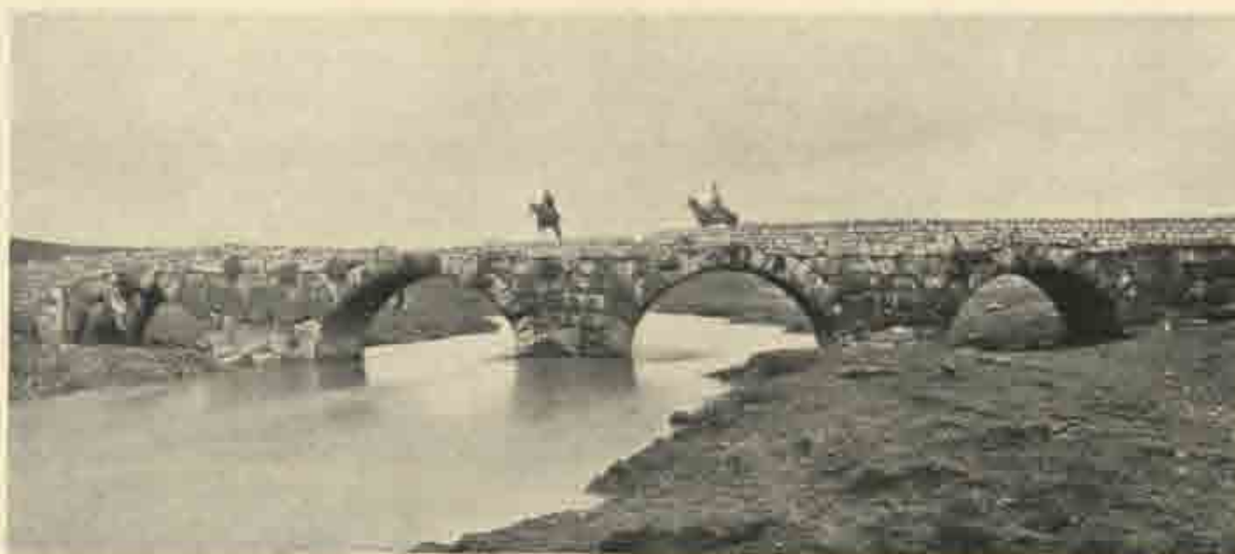
Djār il-Maḥḥal, ancient Roman bridge on the road between Hamā and Apamea, about two hours and a half north of the former. The arches are each about 6 m. broad, and the roadway is 5.60 m. wide.
