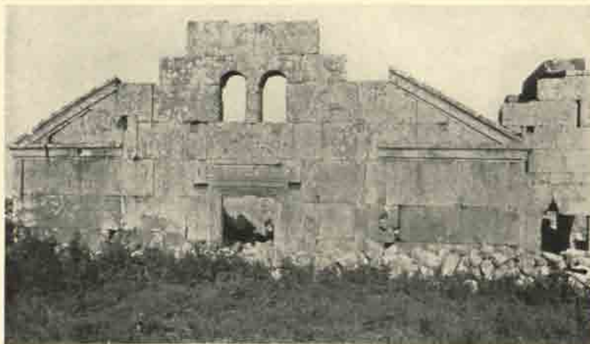
West façade of church at Serdjibeh.
