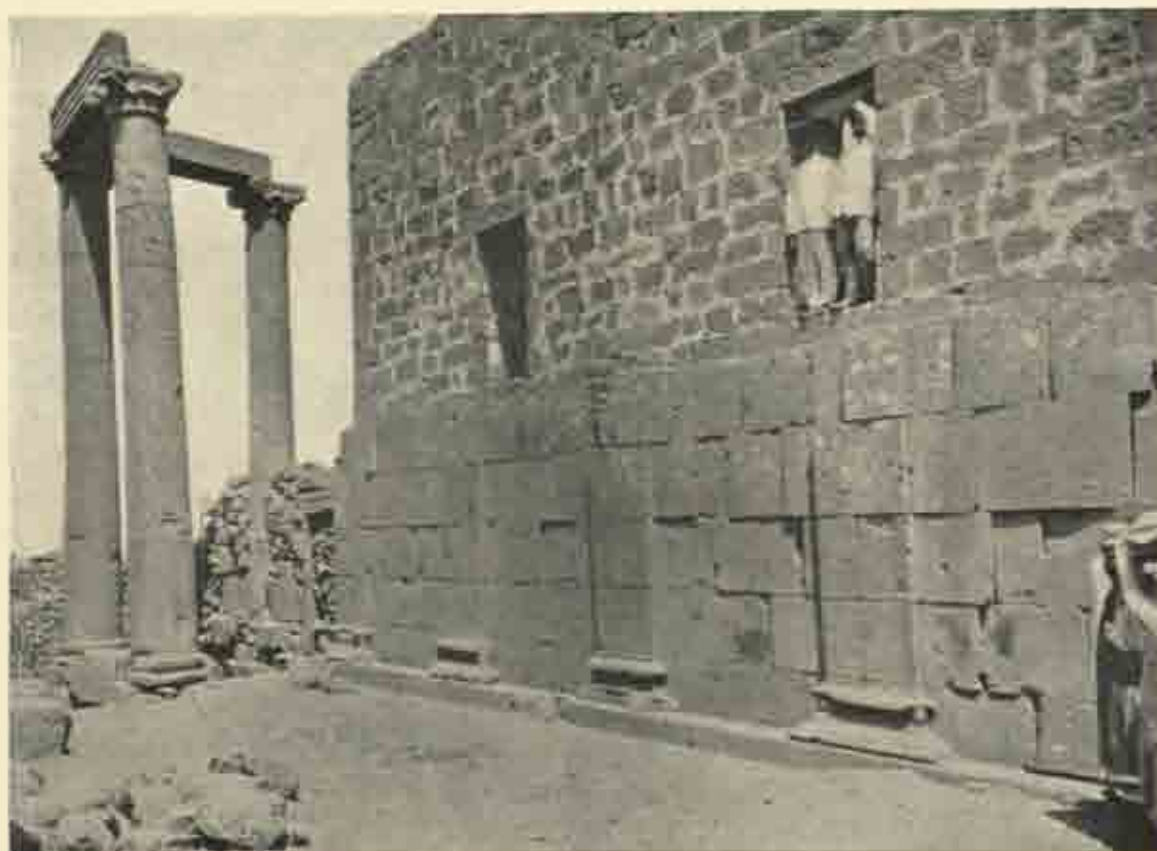
South wall of temple at Suwêda, from the southeast.
