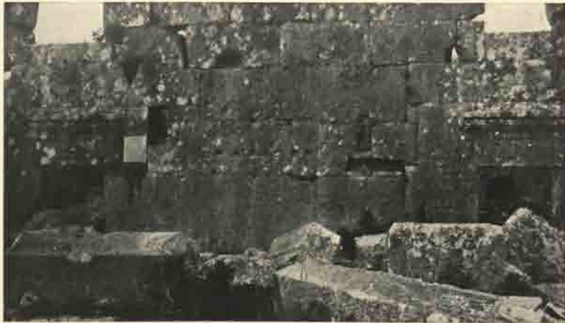
South wall of house at Dêr Sêtâ.
