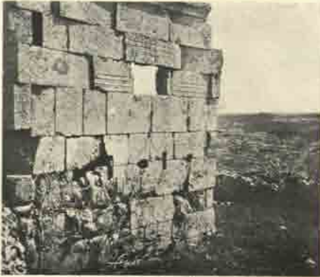
Window with incised moldings at Sakhrin.
