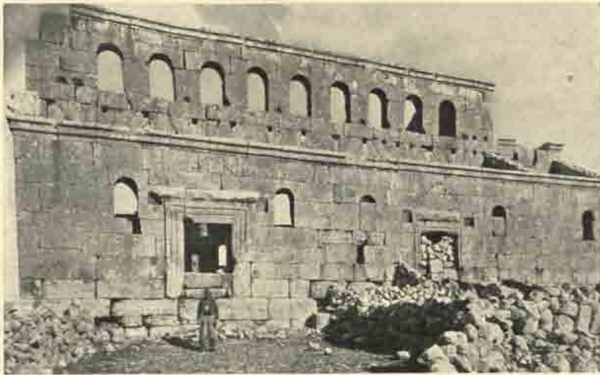
Church at Mshabbak, from the southwest, showing aisle wall and clearstory.
