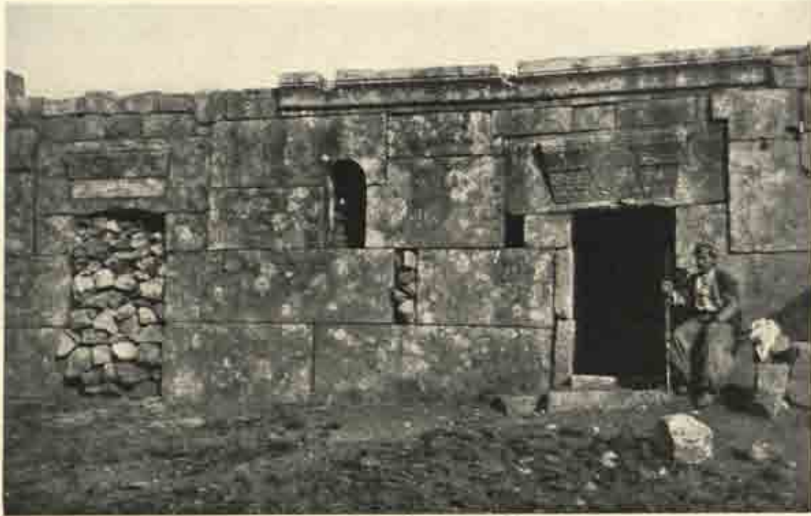
South wall of church at Khirbit Hasan.
