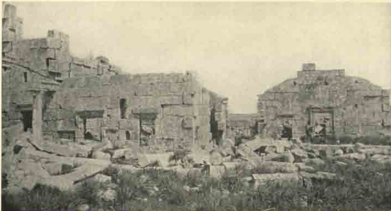
Ecclesiastical buildings adjoining south side of church at Khirbit Häss.
