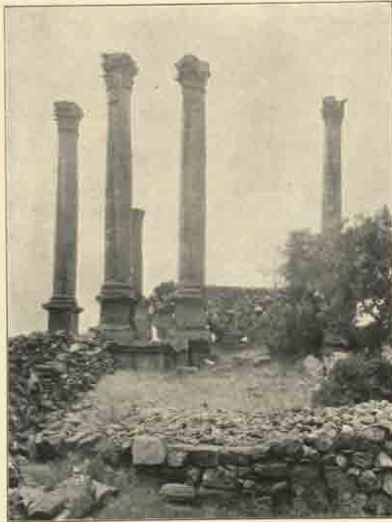
Peripteral temple at Kanawât, from the east.
