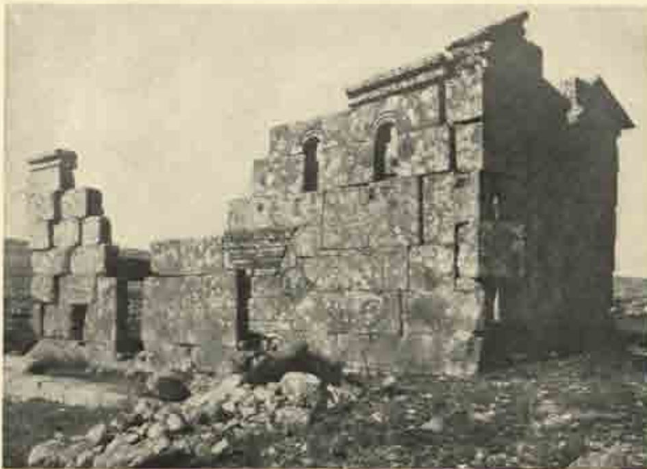
Public building at Bānakfūr, from the southeast.
