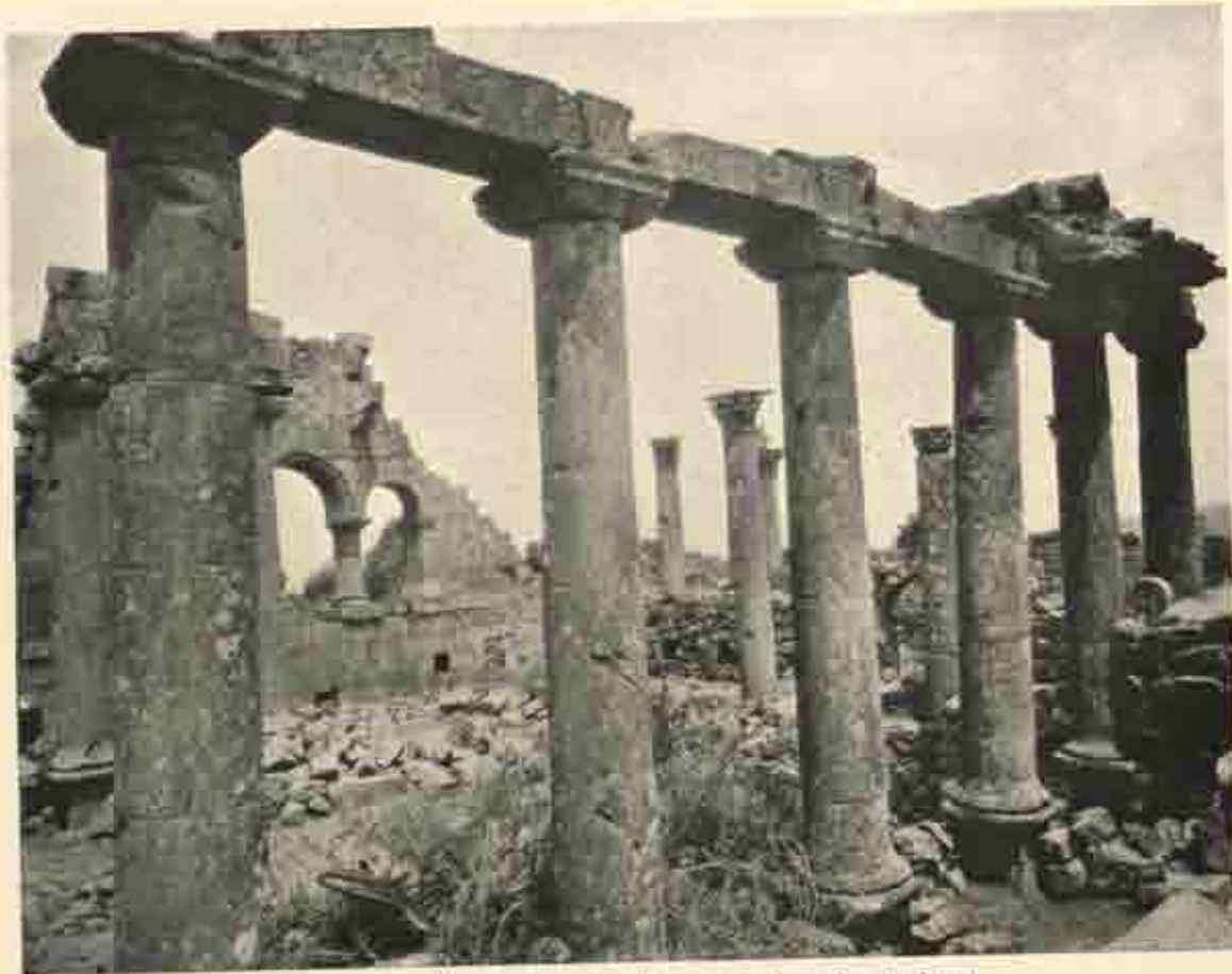
Atrium of basilica in Serâyâ at Kanawât, from the southeast.
