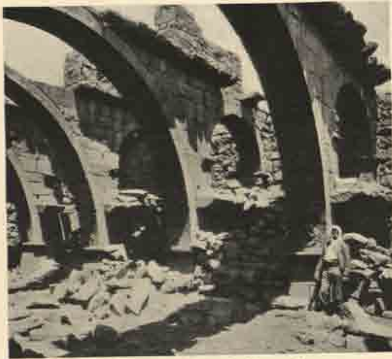
Interior of church at Tafhä, looking northwest.
