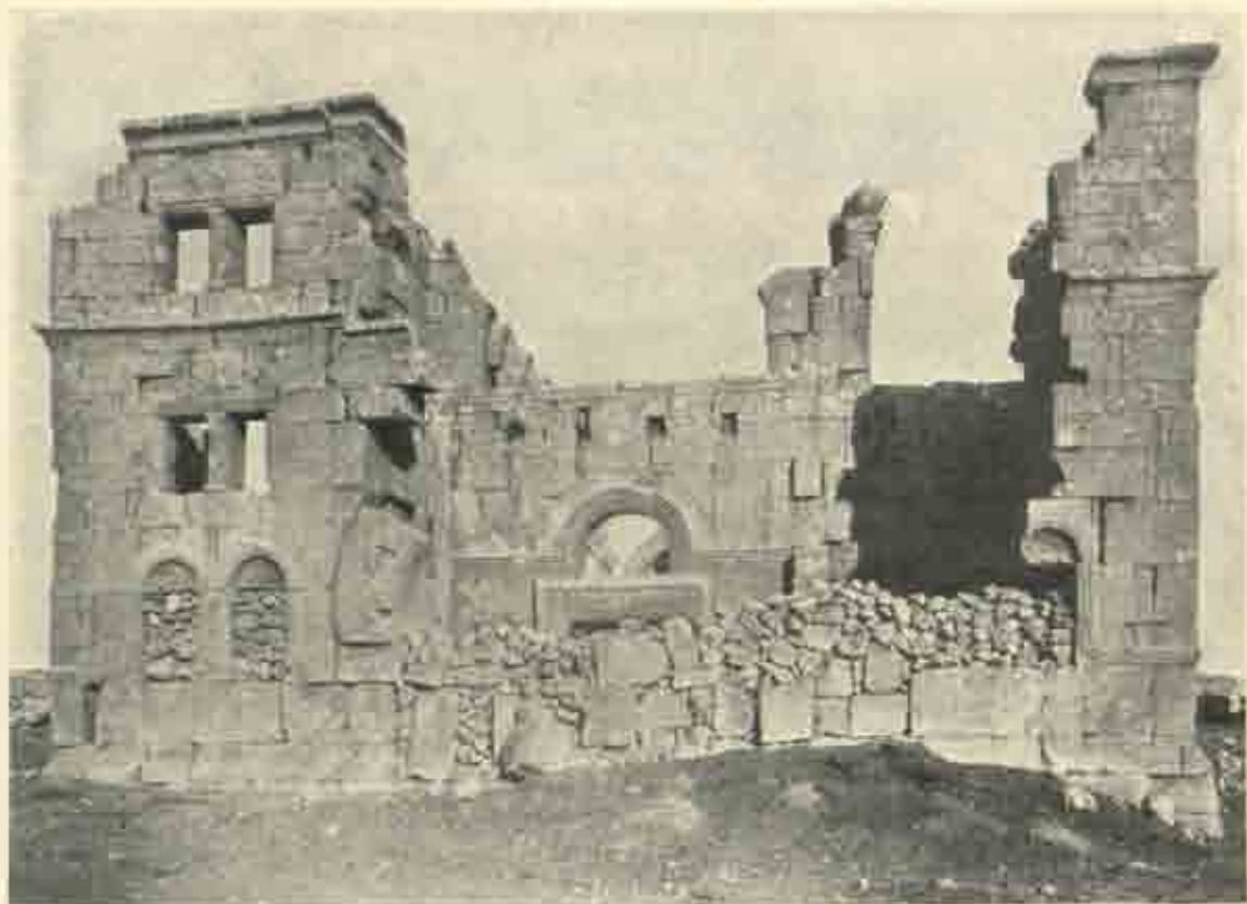
West façade of church at Kaly Lauzeh.
