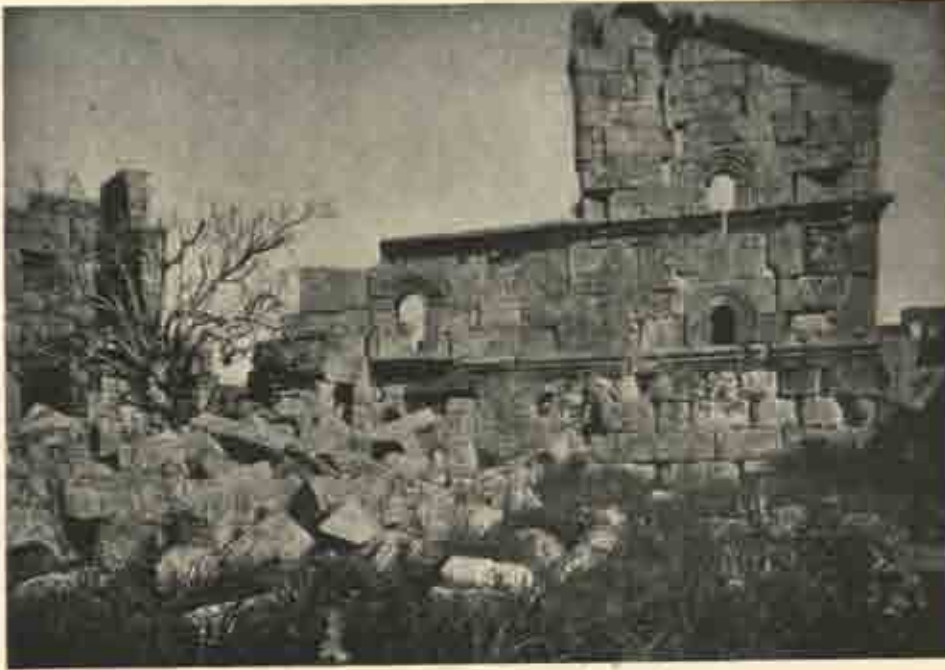
Chapel at Midjleyā, from the south.
