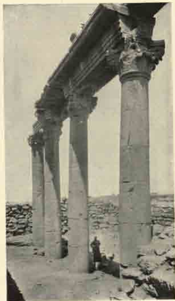
Inner face of north portico of temple at Suwêda.
