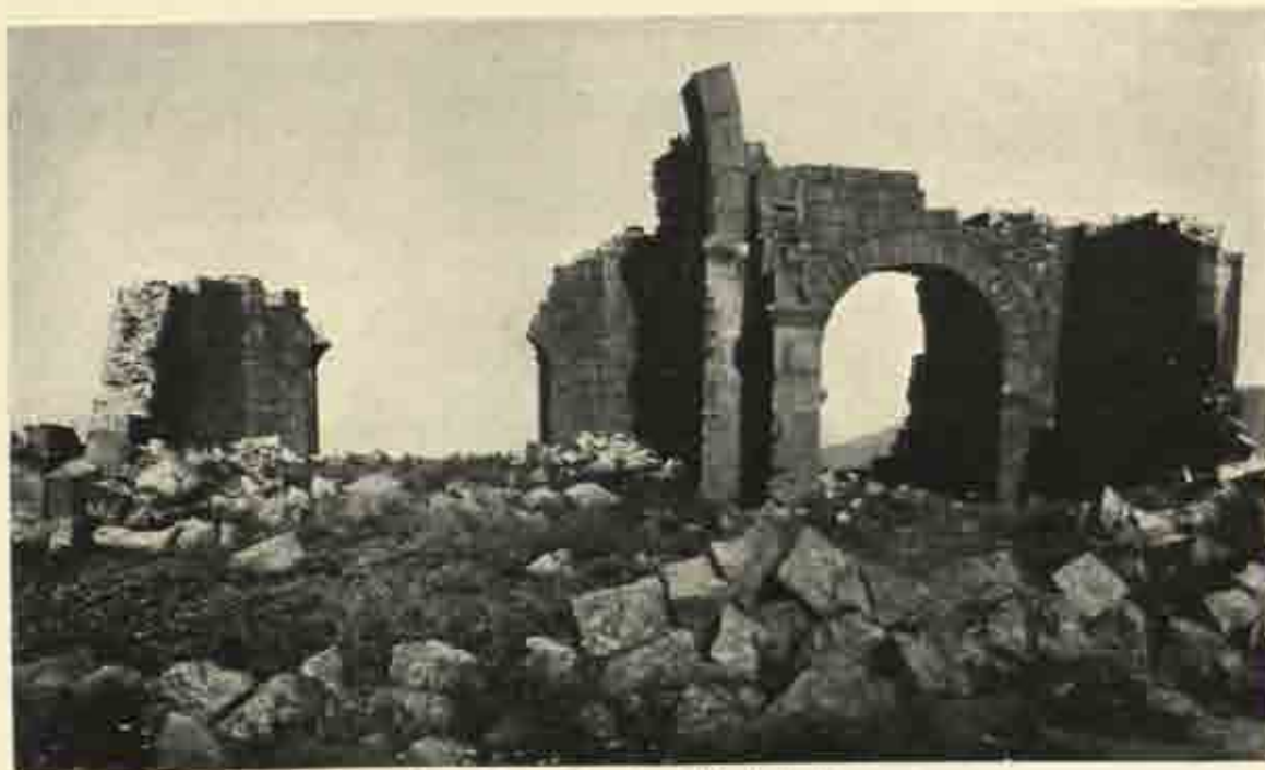
Interior of East Church at Zebed, looking east.
