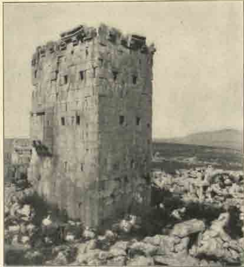
Five-story house at Serdjilich, from the southwest.
