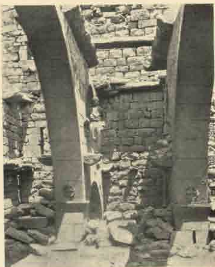
One bay of north aisle of church at Tafhā, showing a roofing slab in place.
