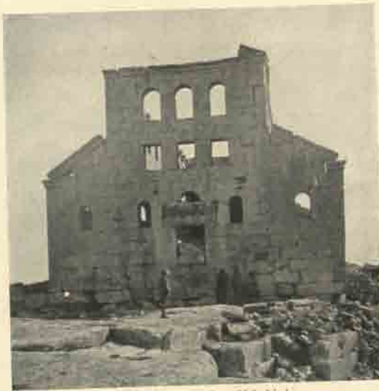
West façade of church at Mshabbak.
