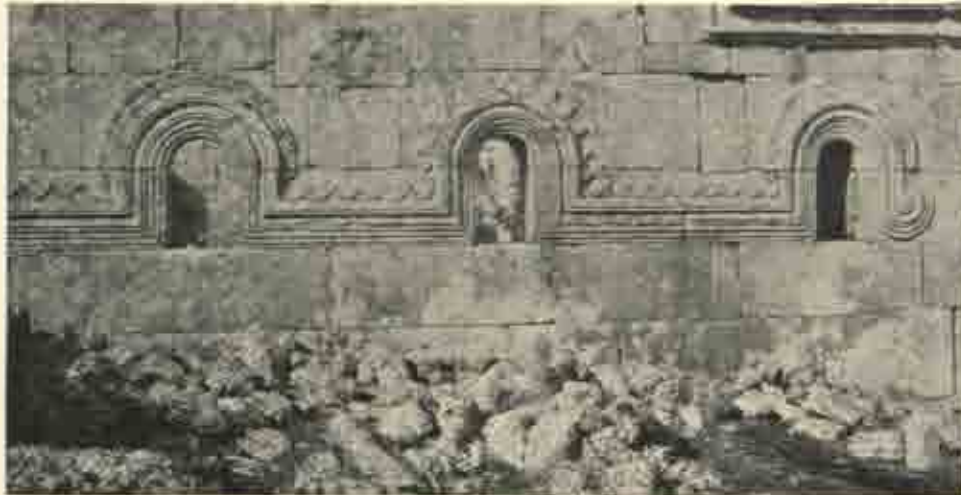
Windows in east wall of East Church at Bakirhâ.
