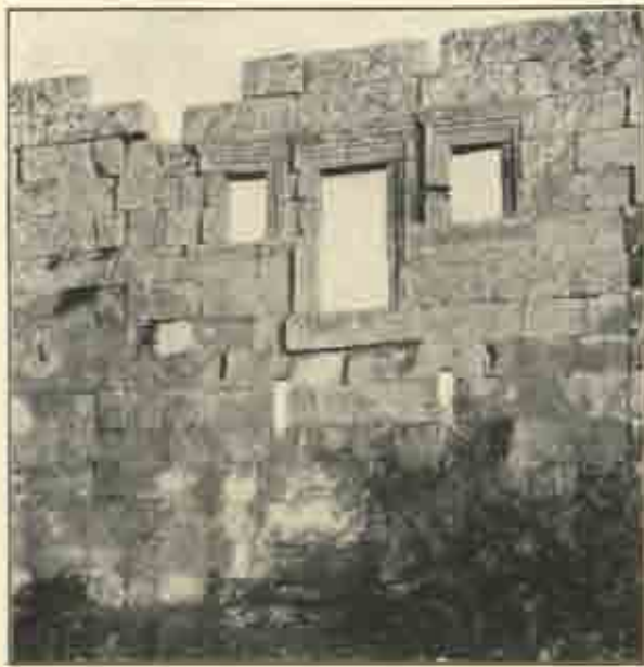
Doorway and windows in rear wall of house at il-Bārah.
