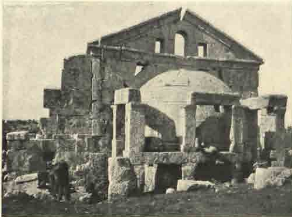
Exterior of apse, chapel at Klēr.
