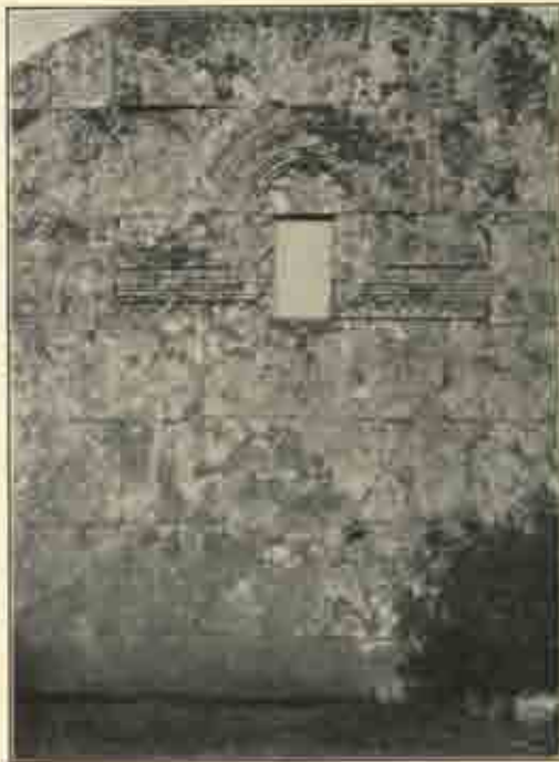
Window in house at Bāshakūh.
