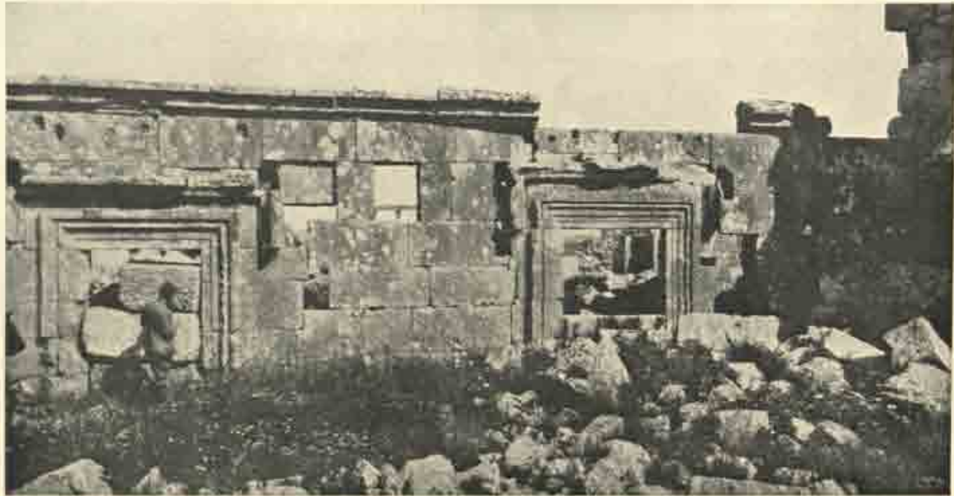
South wall of East Church at Ksédjbeh.
