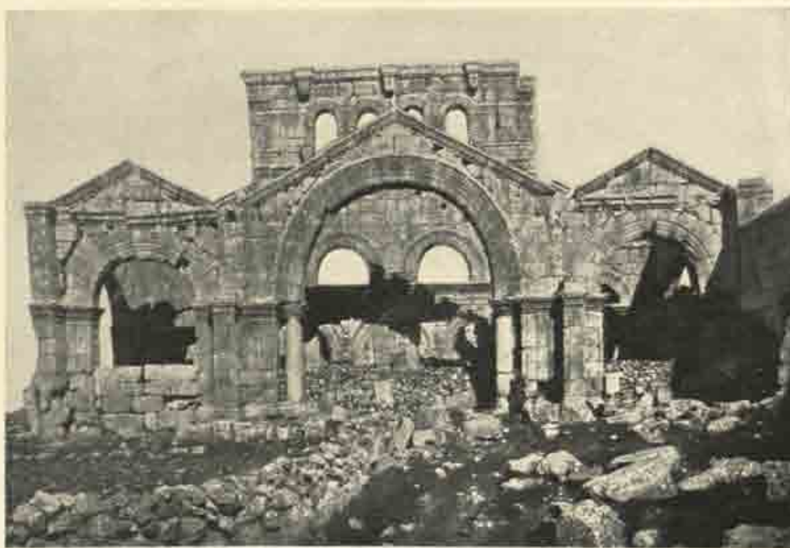
Façade of south wing of Church of St. Simeon Stylites, at Kal'at Sim'ân, the main entrance.
