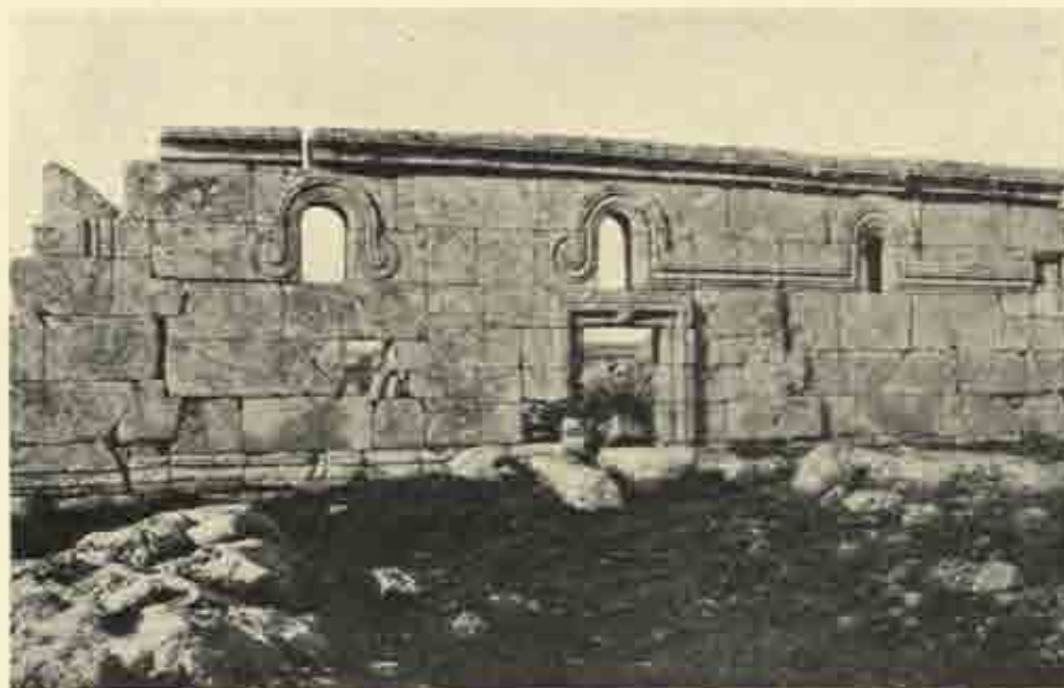
South wall of South Church at Dār Kitā.
