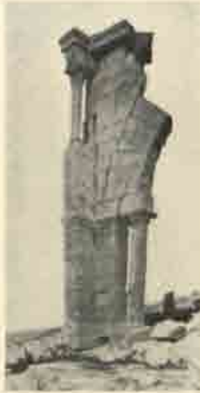
Pier of arch at Dér Sim'ân.
