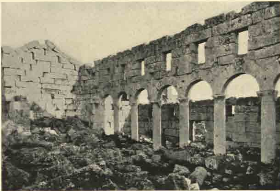
Interior of basilica at Ruwēhā, view from northwest angle.
