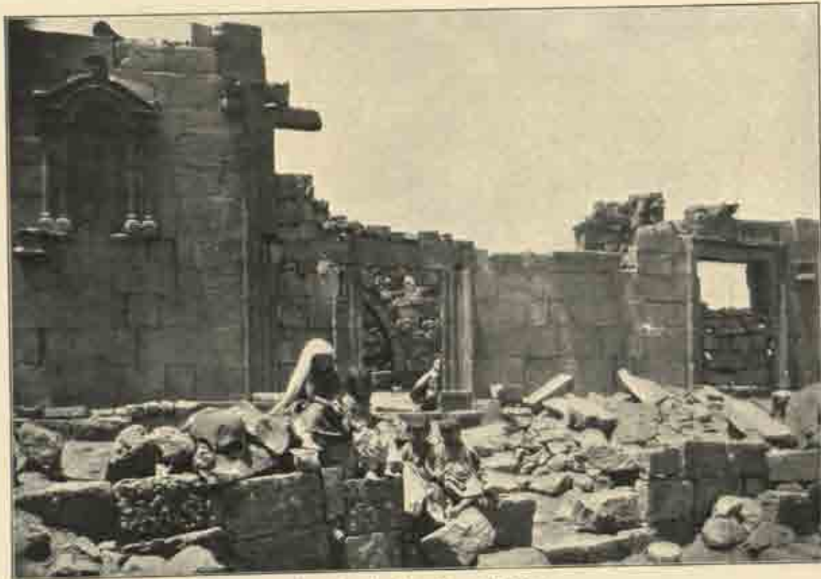
East façade of basilica at Shakkā.
