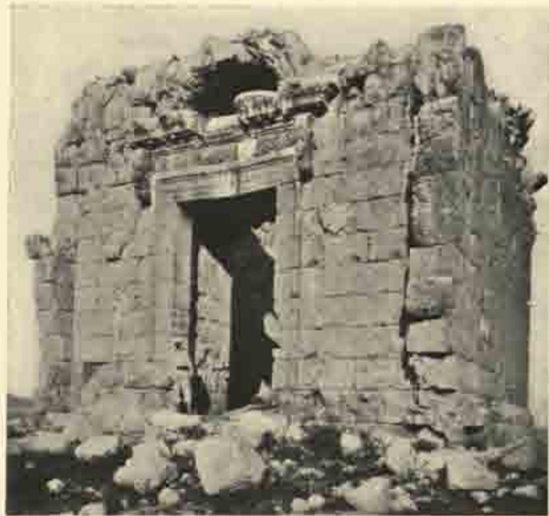
East façade of temple at Isriyeh.
