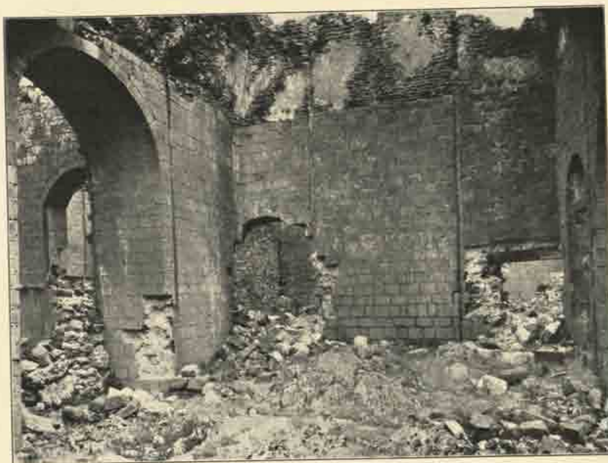
Interior of great-hall (A) of baths at Shehba, from the south.
