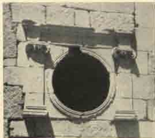
Oculus, originally above large window in palace at Shakkā.
