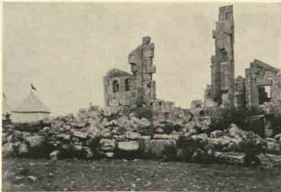
Ruin of large building at Bābiskā, from the southwest.
