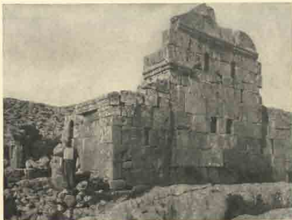
Chapel at Kebr Finsheh, from the southeast.
