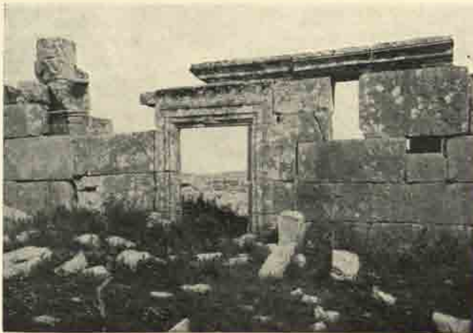
South wall of West Church at Ksēdjbeh.
