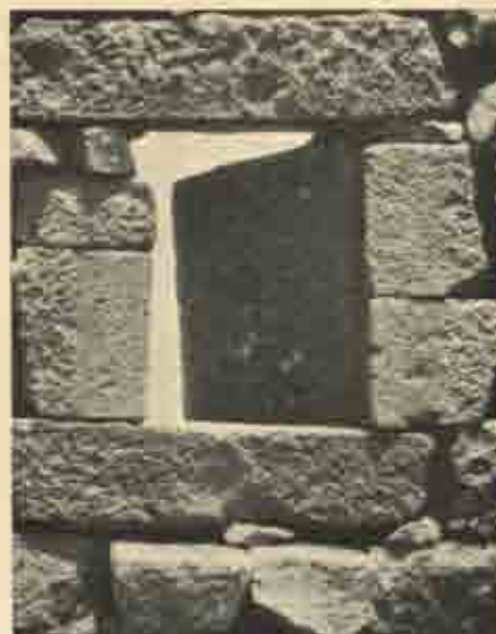
Window with stone shutter in tower of church at Tafhä.
