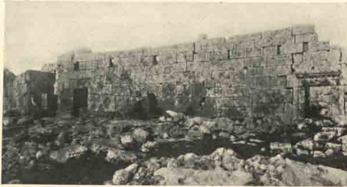
South wall of insula at Kırık Bēza.
