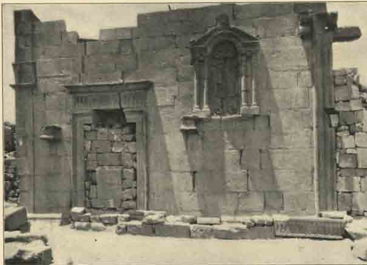
Southern half of east façade of basilica at Shukka.
