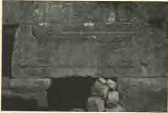
Lintel at Bshindelâyâ.
