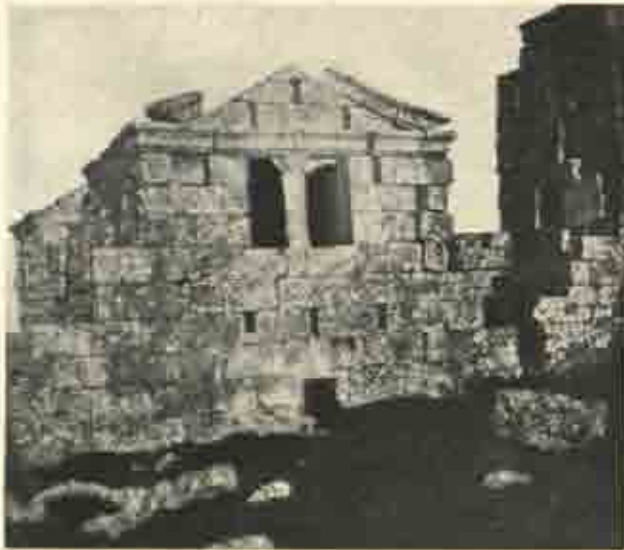
West end of clerical residences and tower adjoining church at Djerâdeh.
