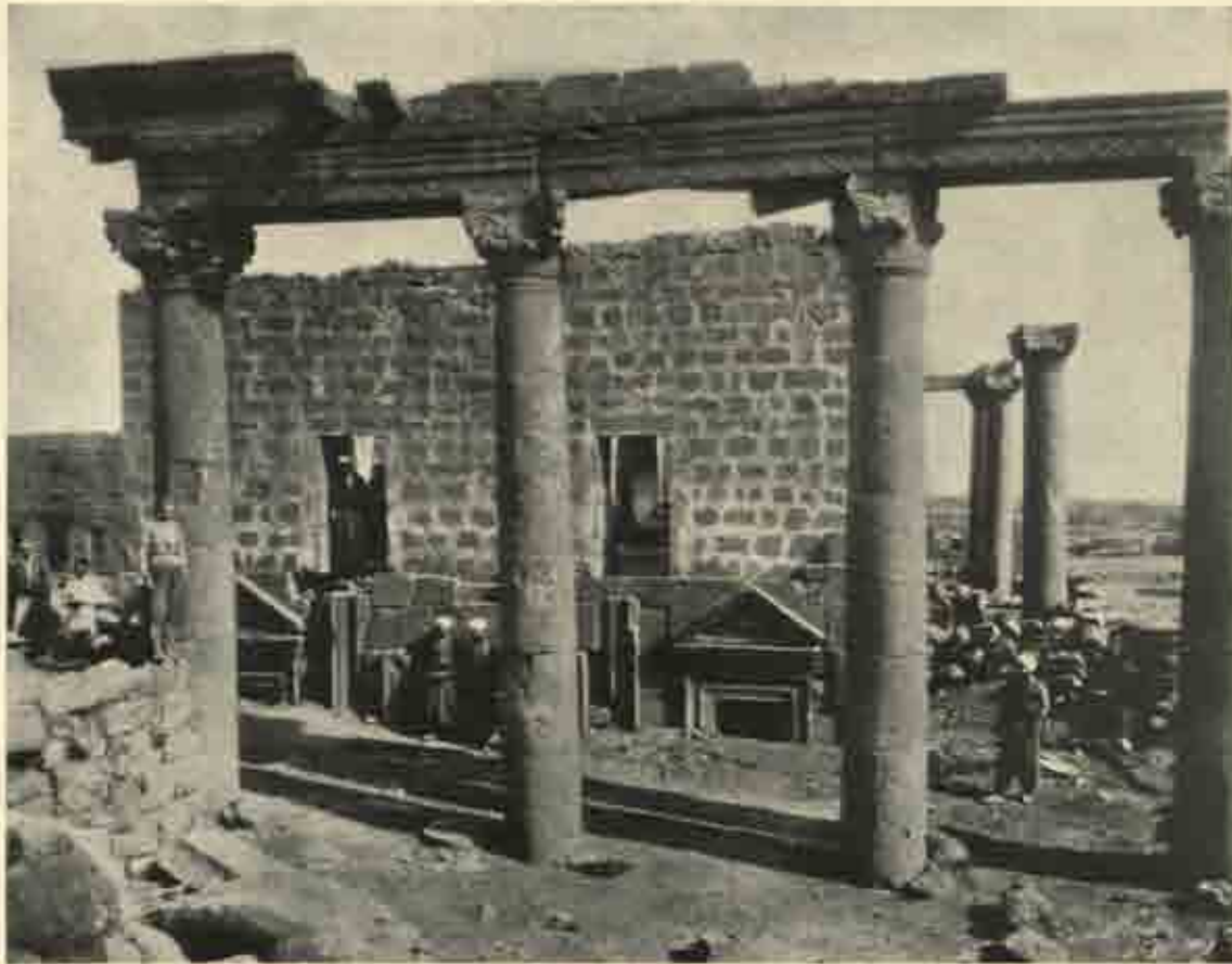
Columns and entablature of north façade of temple at Suwêda.
