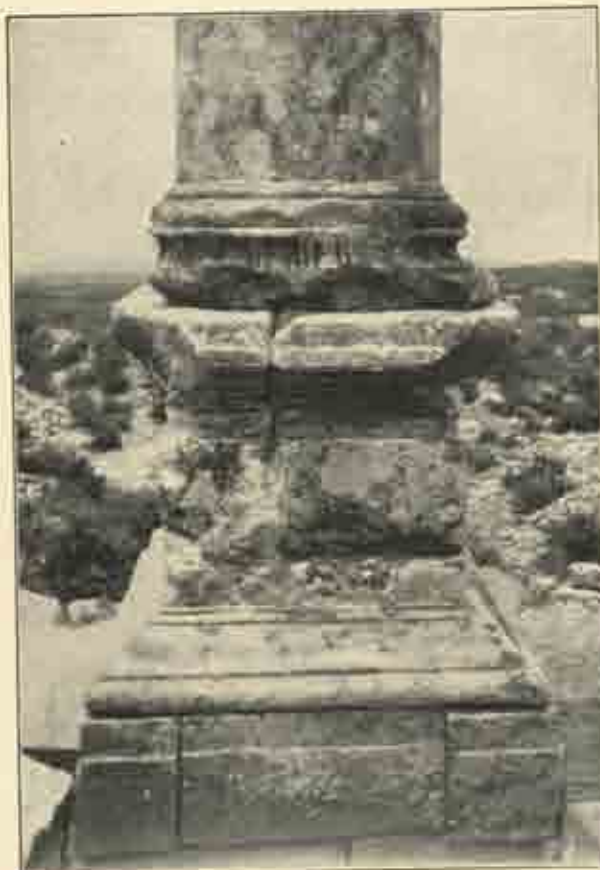
Pedestal and base of a column of the peripteral temple at Kanawât.
