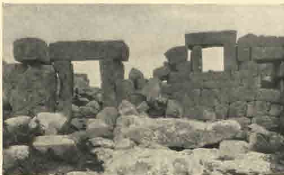
Front wall of house in polygonal style, at Bānkūsa.
