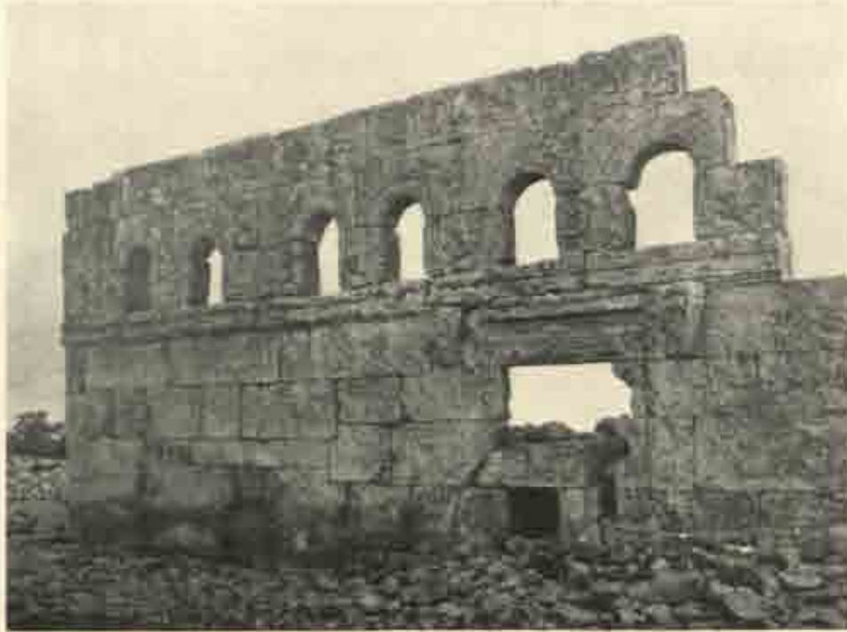
North wall of South Church at Kōkanāyā.
