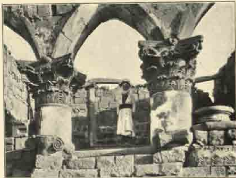
Capitals of hexastyle temple at Shehba, built into crude modern structure.
