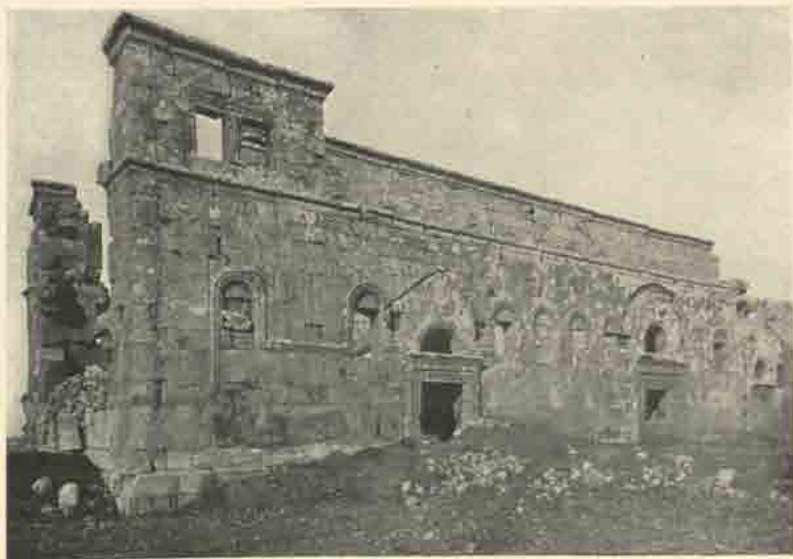
Church at Kaly Lauzeh, from the southwest.
