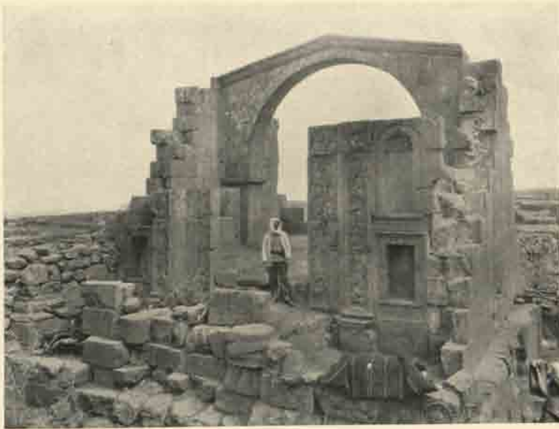
North temple at 'Atil, from the southeast.
