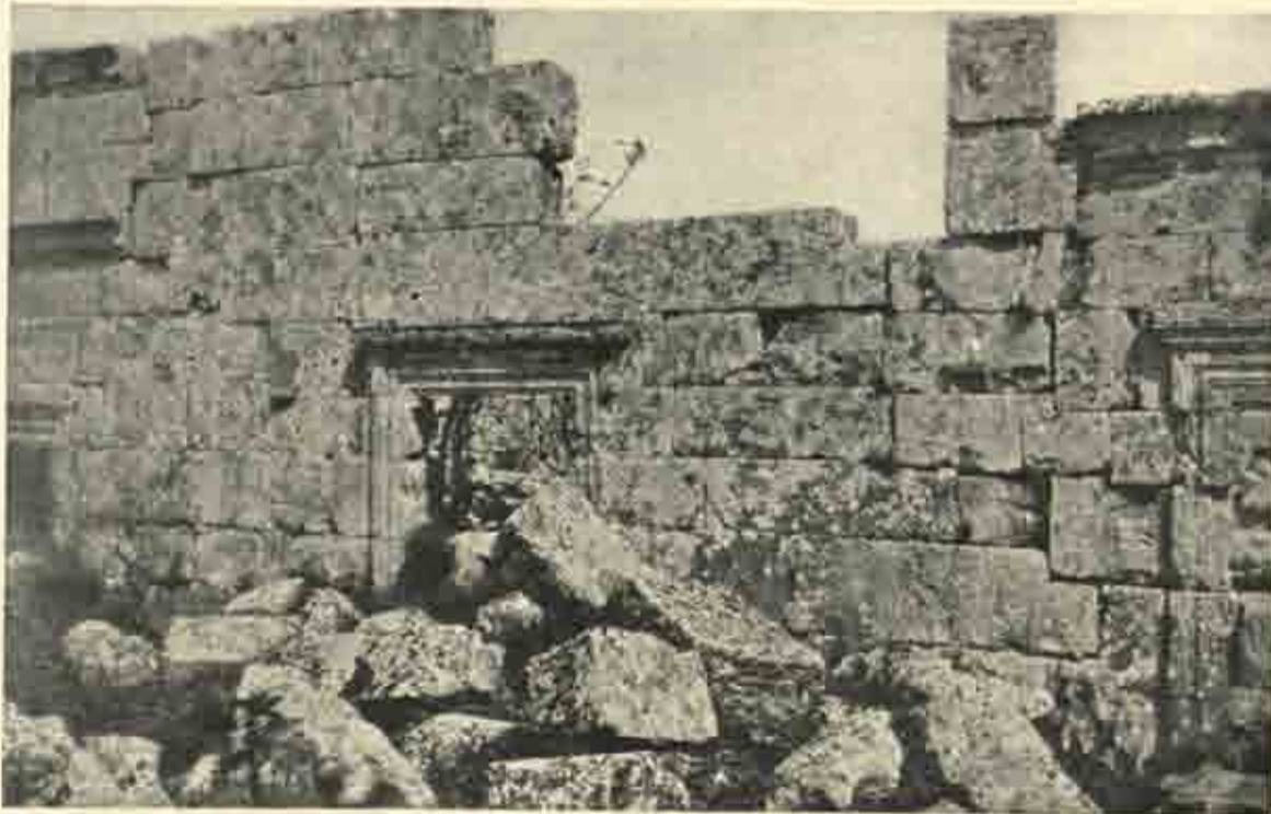
Church at Dêr Sambil, west front.
