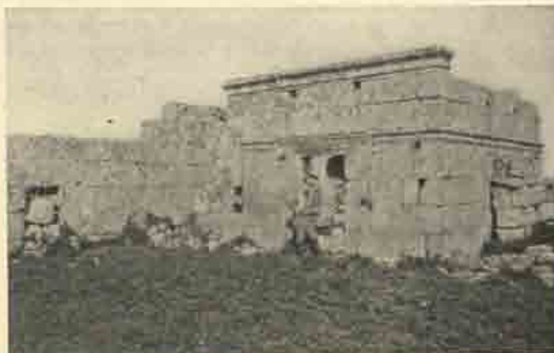
Baptistery at Rbê'ah, from the southwest.
