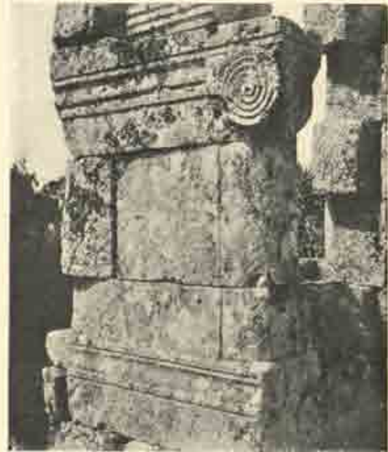
Engaged column of upper colonnade at Sakhrin.
