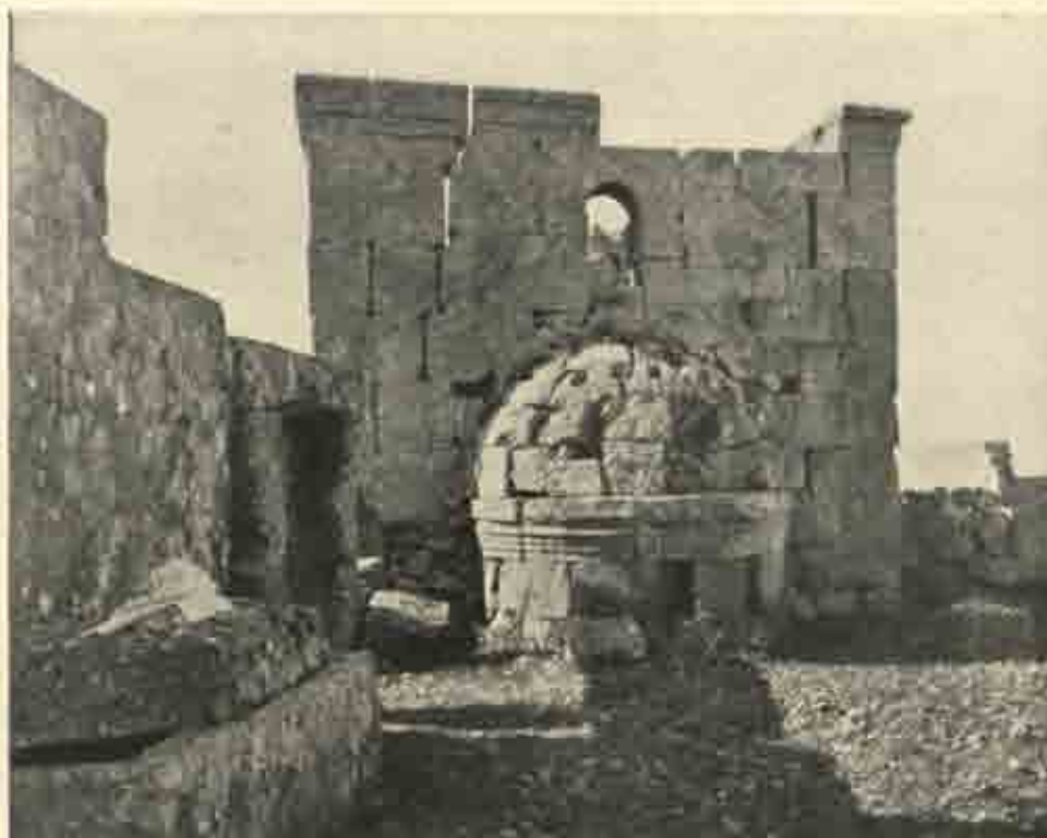
East wall of baptistery of church of Paul and Moses, at Dār Kītā, showing exterior of apse.
