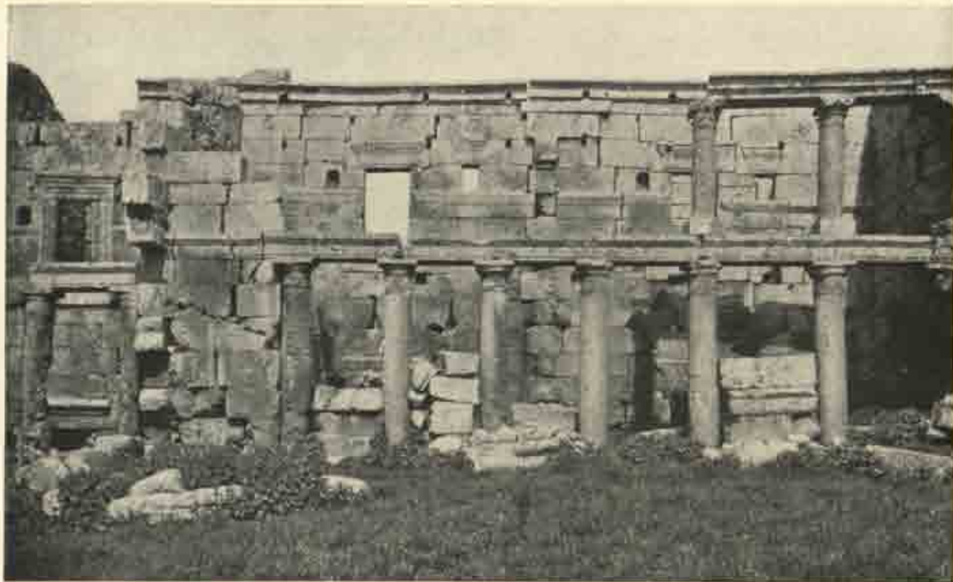
South wall and porticos of older part of villa at Serdjillā.
