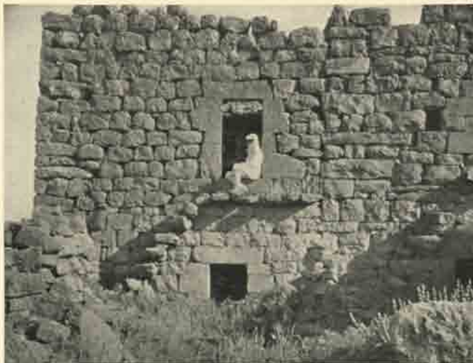
Wall of roughly squared blocks laid dry, at il-Malikiyeh.
