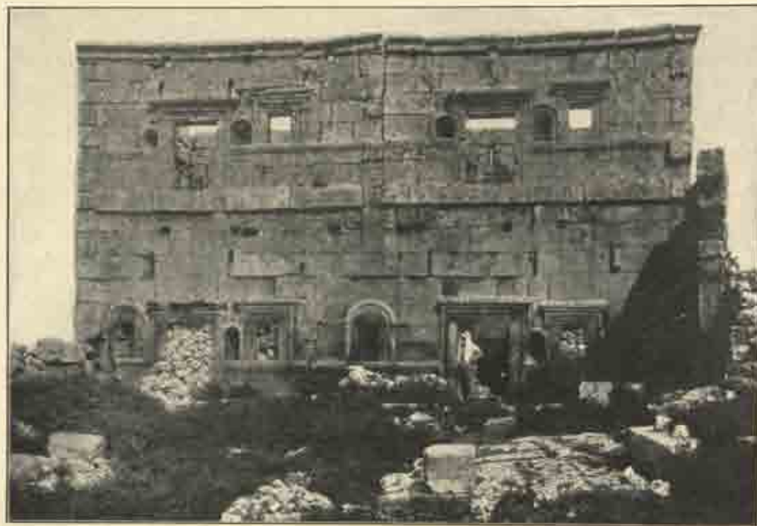
Front wall of house at Serdjilla.
