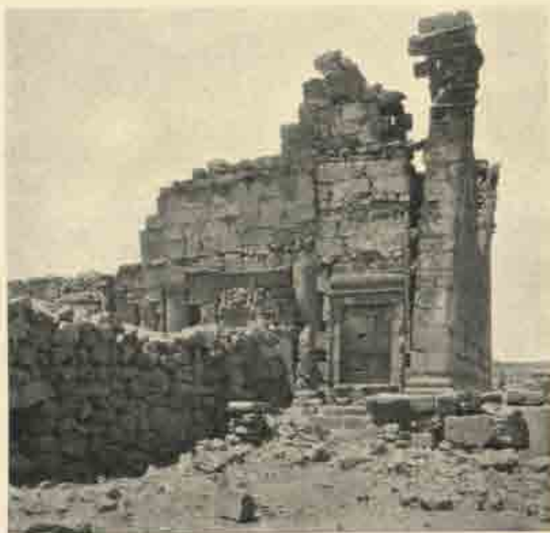
Modern wall of ancient fragments built between the antæ and columns of the temple at Mushennef.
