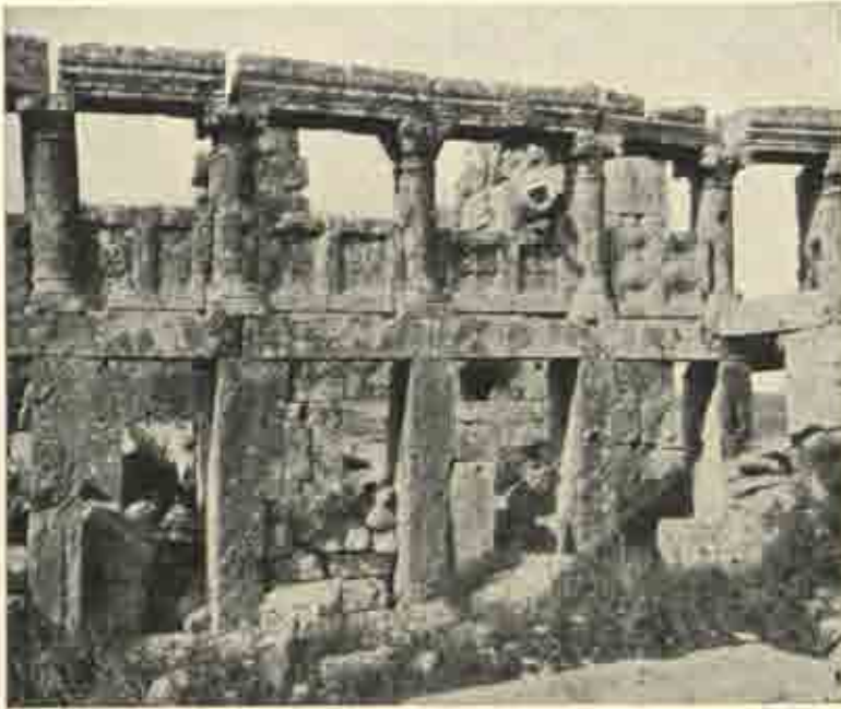
House II at Serdjibleh, facing south.
