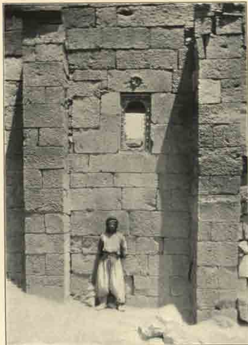
Buttresses and window in south wall of palace at Shakkā.
