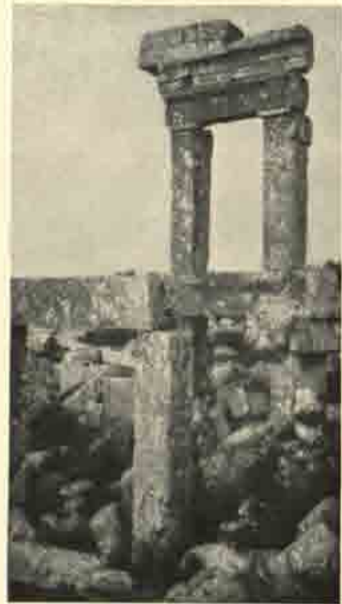
Superposed doorways of a house at Dêhes.
