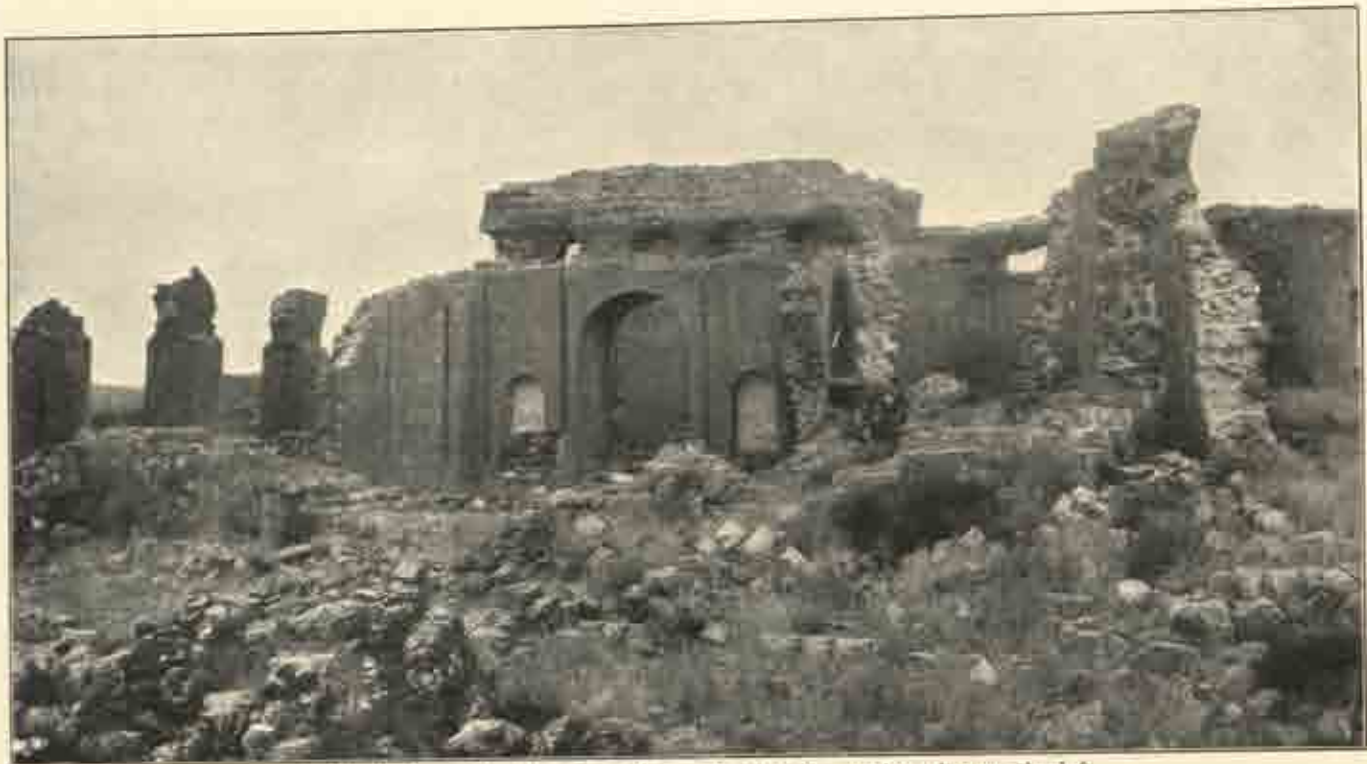
Public baths at Shehbā, from the northeast; piers of aqueduct at the left.
