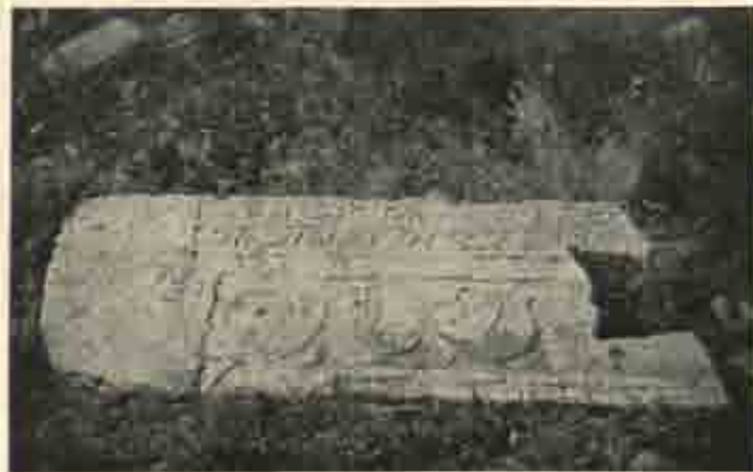
One half of two-piece lintel showing dovetail joint at Khanásir.
