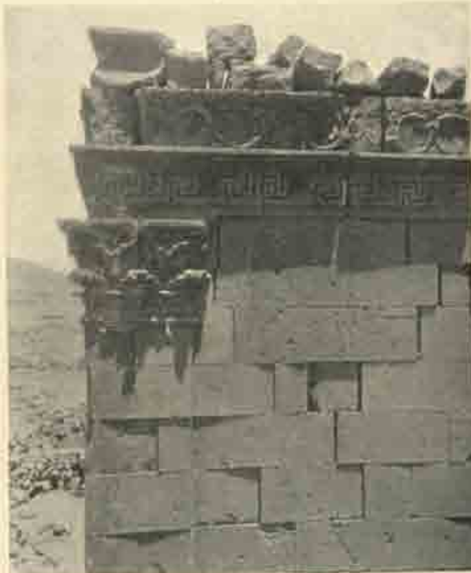
Pilaster-cap, architrave, and frieze; southwest angle of temple at Mushennef.
