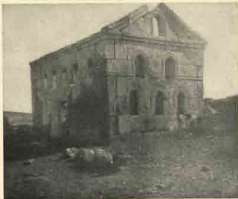
Chapel at Burdj id-Dērūnī, from northwest.
