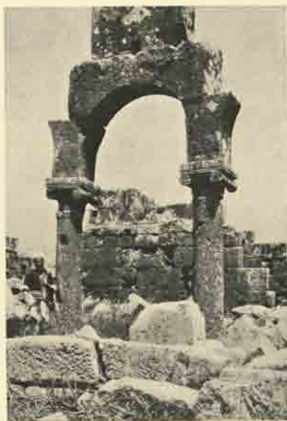
A development of the arcuated lintel, at Bāb il-Hawā.
