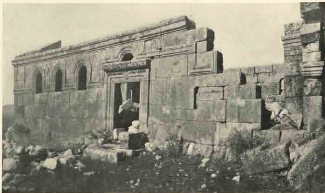
South wall of church at Khirbit Tēzin.
