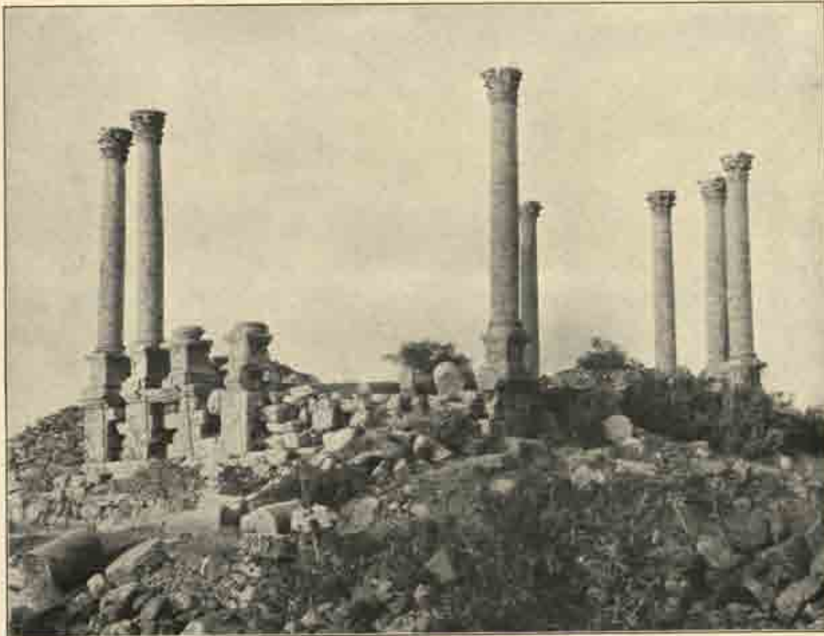
Peripteral temple at Kanawāt, from the southwest.
