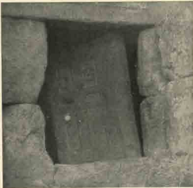
Door of basalt in ground story of tower at Djerâdeh.
