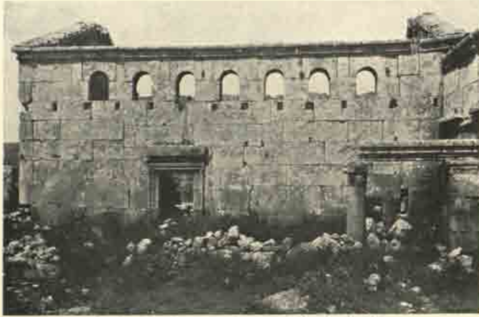
South wall and remains of portico of the chapel at Srir.
