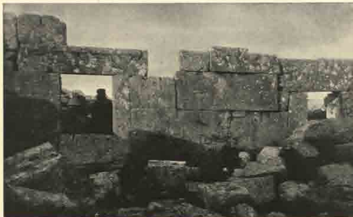
Exterior of south wall, North Church at Bānḳūṣā.
