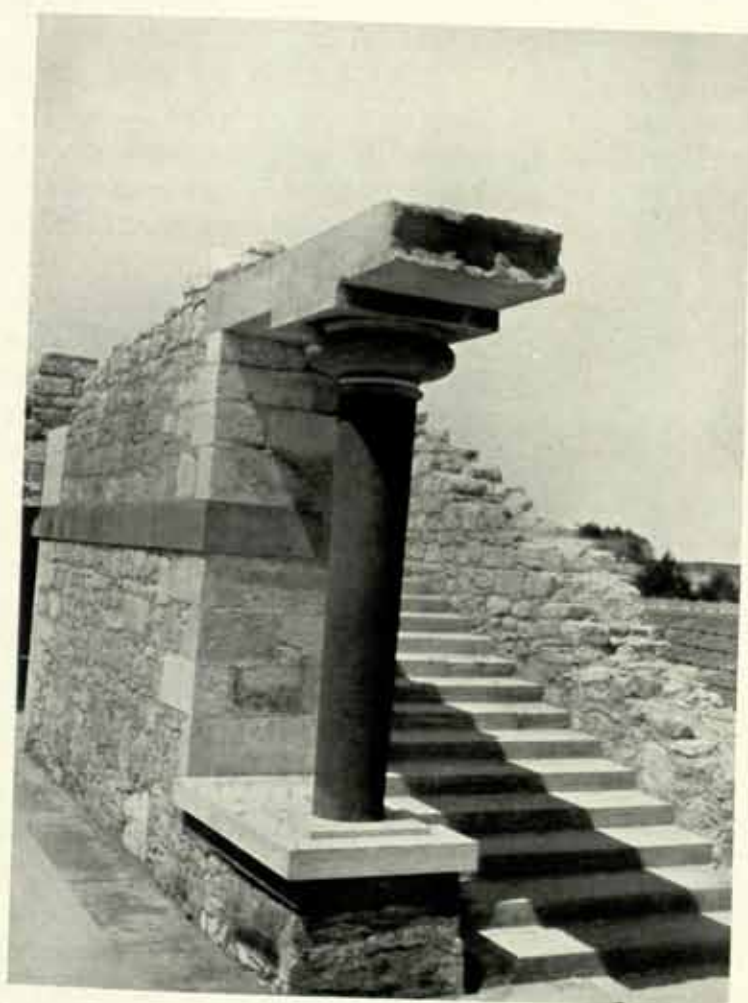
FIG. 535. STAIR BLOCK IN POSITION WITH MARKS OF ASCENDING STEPS, AND WITH RESTORED COLUMN AND FIRST FLIGHT OF CENTRAL STAIRCASE.
