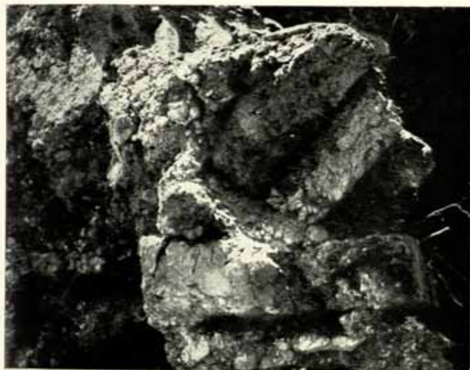
FIG. 320. SUN-DRIED BRICKS: FROM UPPER STORY, 'LITTLE PALACE'.
