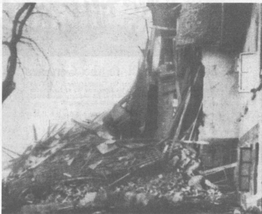
Unanswerable comment on Germany's claim to have taken Norway under her "protection" is afforded by this radio photograph, the first to reach this country, of the damage done in Oslo by Nazi bombers. The ruin is that of one of the houses in the suburbs bombed on April 9, 1940.
