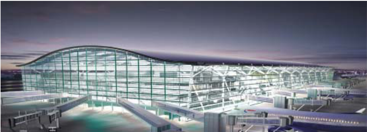
Heathrow Terminal 5 (under construction)
