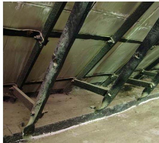
Figure 10: Base detail showing wall plate (Heres 2012)
