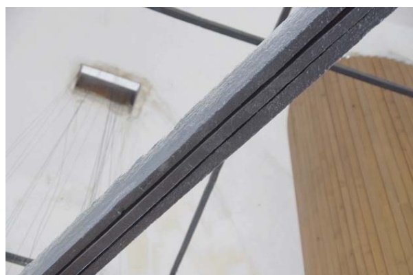
Figure 7: Tie rod showing forging (Lorenz 2012)
