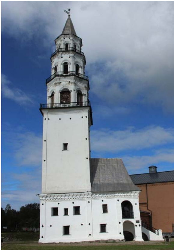
Figure 1: Tower and porch (Lorenz 2013)
