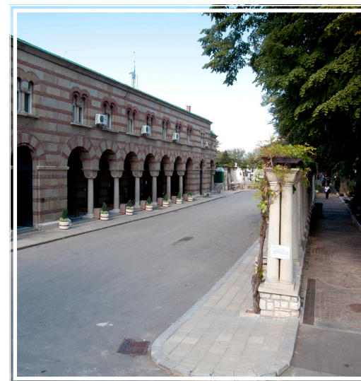
Farewell Chapels and access plateau with the colonnade designed by arch. Rajko Tomic
