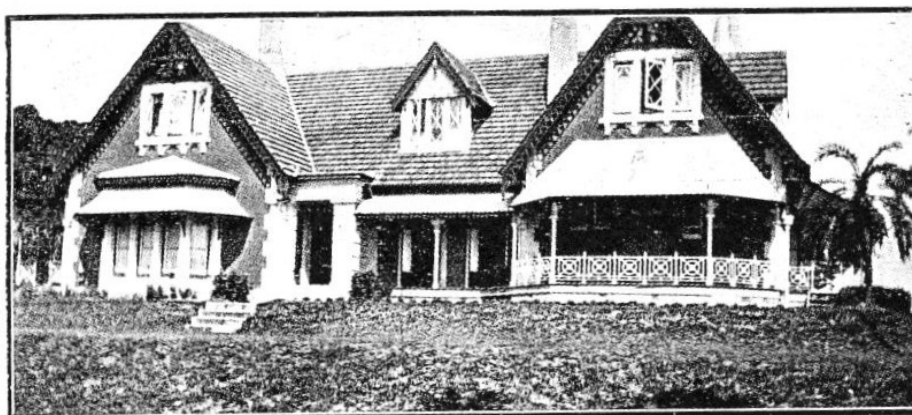
FRONT VIEW OF SHAFSTON HOUSE, FROM THE RIVER SIDE. This building was erected by the late Mr. C. M. Foster on the site of the original Shafston House, which was the home, in turn, of several of Brisbane's prominent citizens of the last century.—See page 7
