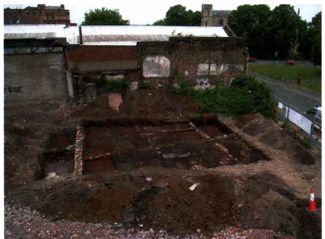
Plate 5 Area 3 looking south-west towards Trinity Church. To the right is Trinity Street.
