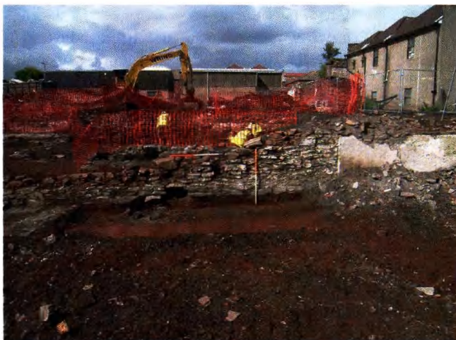
Plate 4 Area 2 showing east facing elevation of wall 2039, the former eastern exterior wall of Fears' Building. Scales 2m.
