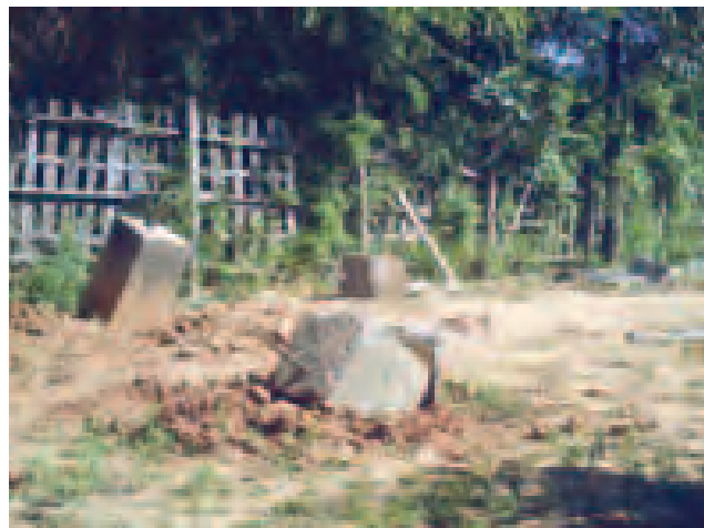
Church foundation destroyed, Kalaymyo township
