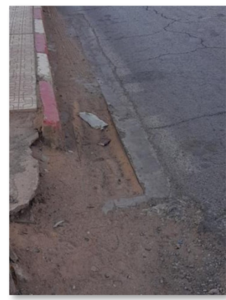
Drains filled with sand. This is what happens in regions where there is more sandstorm than rain.
