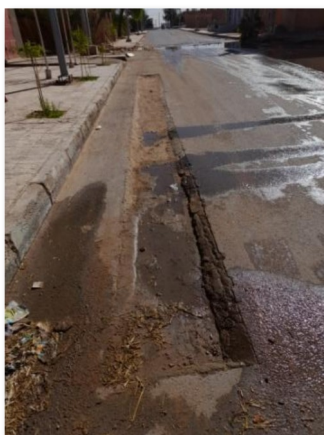
Drains filled with sand. This is what happens in regions where there is more sandstorm than rain.
