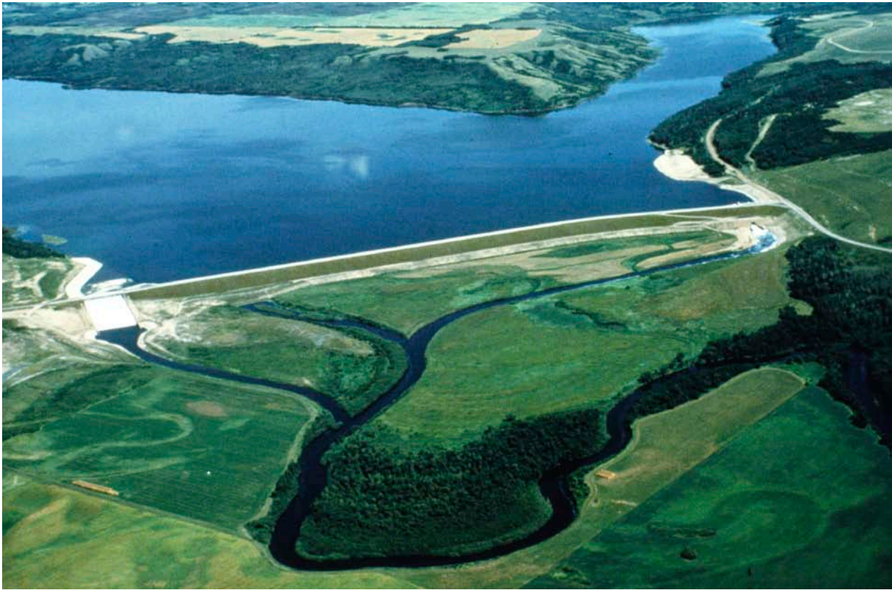
Figure 26: An aerial view of the Shellmouth Dam looking upstream. The outlet for the conduit is on the right hand side of the photo and the spillway is on the left hand side of the photo.
