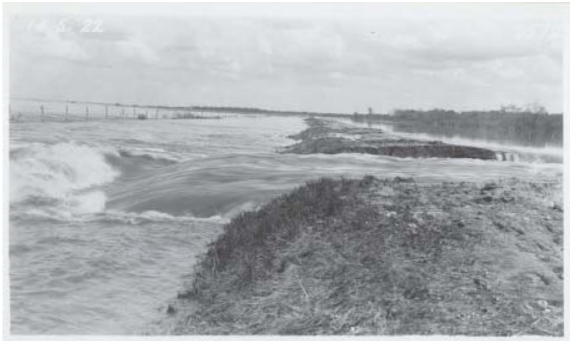
Figure 16: Photograph from 1922. A hole was blasted in the Winnipeg-Portage highway two miles east of Poplar Point to pass waters north and prevent destruction of the entire road (Attwood, 1923).
