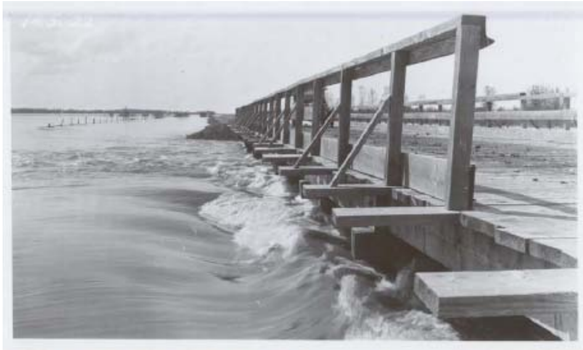
Figure 18: Photograph from 1922 showing water flowing north under a bridge on the Winnipeg-Portage highway that was reported to be normally dry (Attwood, 1923).
