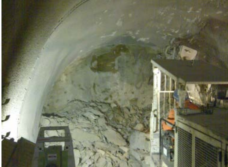
Face position after mucking Adv 29 & 30
