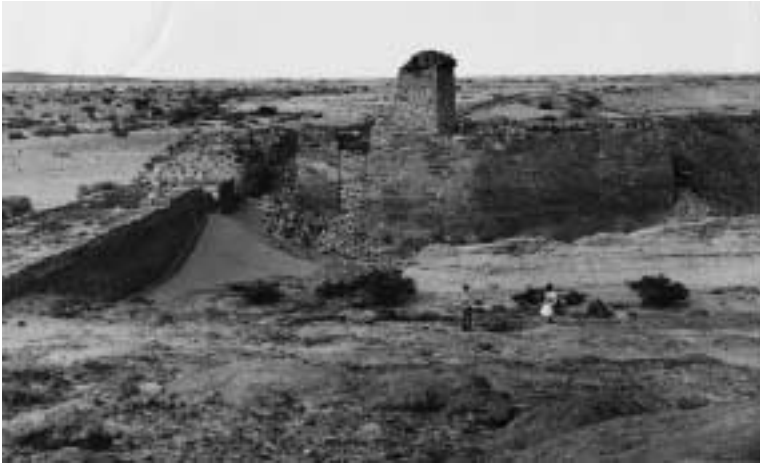
Plate 14 Marib dam, ancient ruins of northern sluice system (AFSM).
