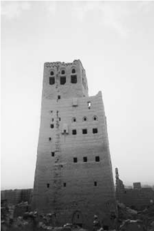
Plate 23 Mud-brick house in old Marib (author).
