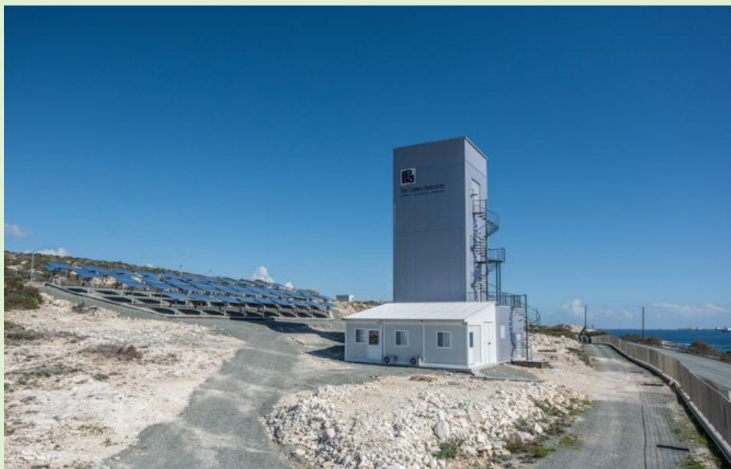
Our solar thermal field spreads out over half an acre in Cyprus, overlooking the Mediterranean Sea.
