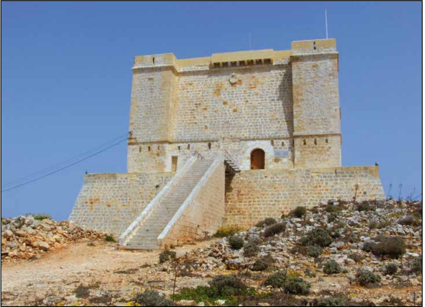
Comino Tower stairs
