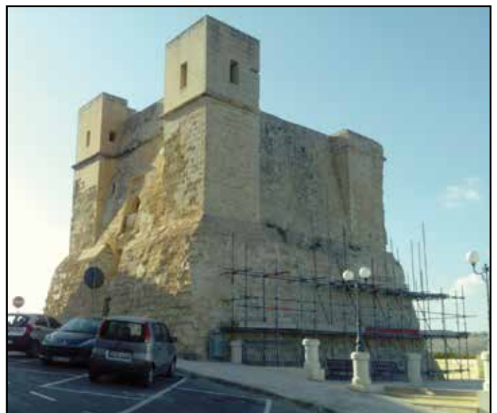
Wignacourt tower being enclosed by scaffolding
