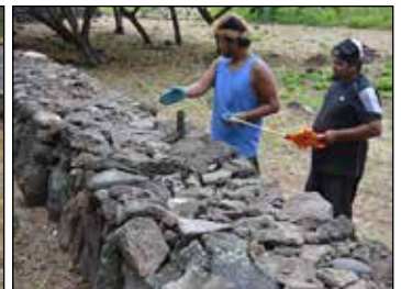
Rock wall restoration in Nāpali, Kauaʻi.
