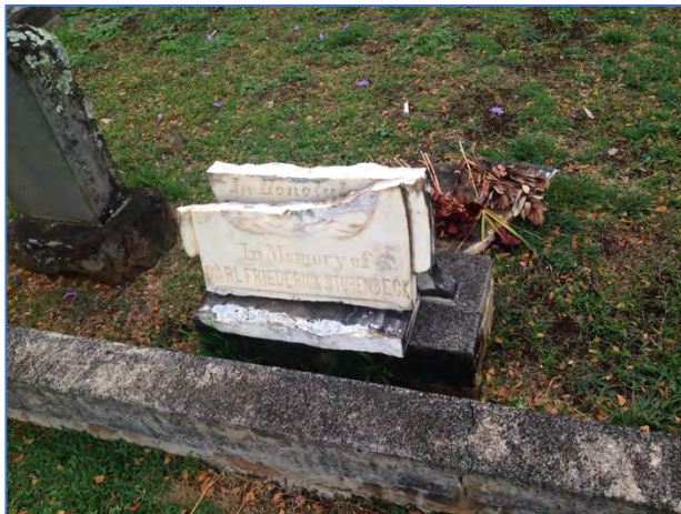
Left and right: Kawaiha'ō flawed stones that cracked as a result of weathering and moisture seeping into those flaws. These stones have slotted pedestals.
