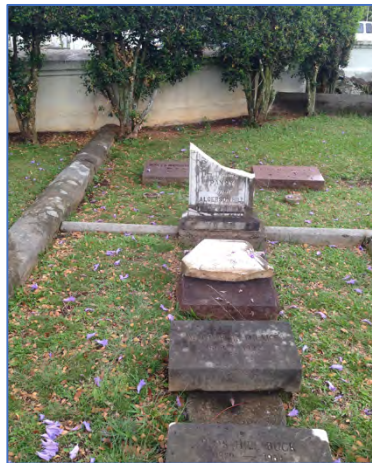
Left and right: Kawaiha'ō flawed stones that cracked as a result of weathering and moisture seeping into those flaws. These stones have slotted pedestals.
