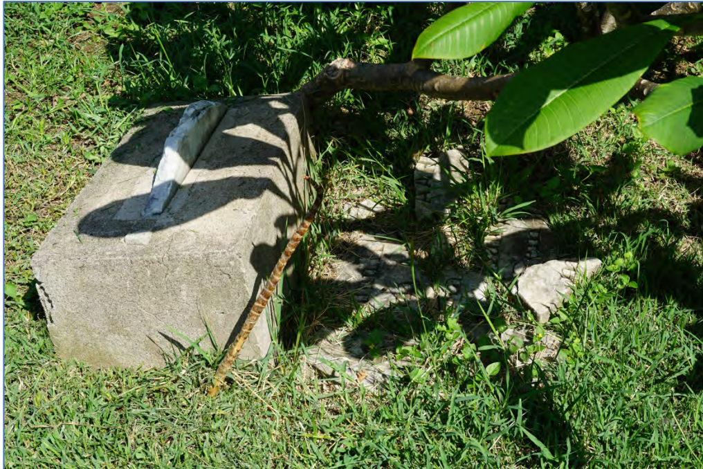
A Makiki Cemetery slotted pedestal formerly holding a very thin marble headstone (The broken pieces of the headstone are to the right in the grass below.)
