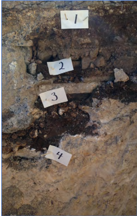
Soil strata in the excavation pit: 1—fill prior to forming the 1963 concrete cap; 2—coarser rubble fill prior to forming the concrete cap; 3—the pavement stratum; and 4—karst.
