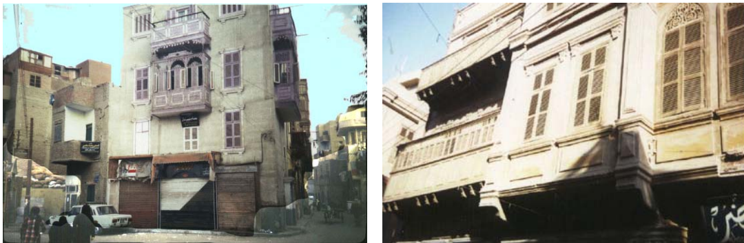
Figure 3-24 The building materials used are burned clay bricks, stonemasonry, and wood.
