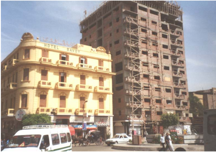
Figure 3-32 Illustration highlights the effect of massive redevelopment with an abrupt change of scale, isolating the remaining building without any possible means of integration.
