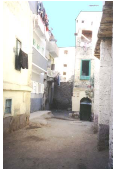
Figure 3-22 Streets are not receiving adequate maintenance, resulting in concentrations of mud in times of rain and heavy dust during the dry season.
