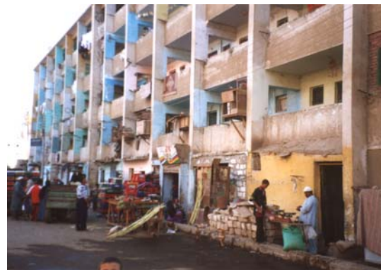
Figure 3-77 Users occupying ground floor flats usually modified this space and transformed it for private use.
