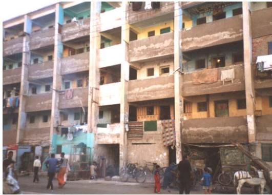
Figure 3-75 To cut costs of the low-cost housing, poor finishing materials were used. The result was a fast deterioration of these buildings
