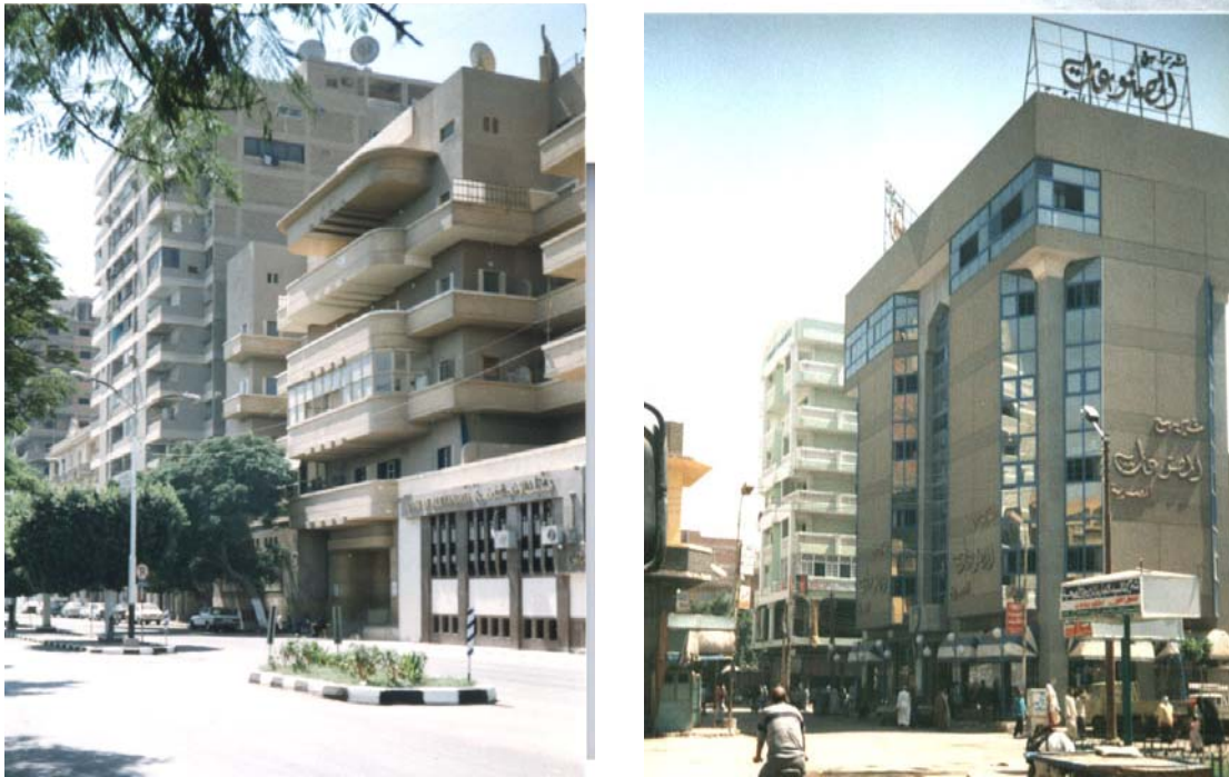
Figure 3-41 The desire for multi-storey building to have a distinct identity can lead to difficulties and a break with the context. In these examples, not only the bulk, but also the general form and use of materials combine to create an overpowering impression. It has destroyed the richness and coherence of this once notable street.
