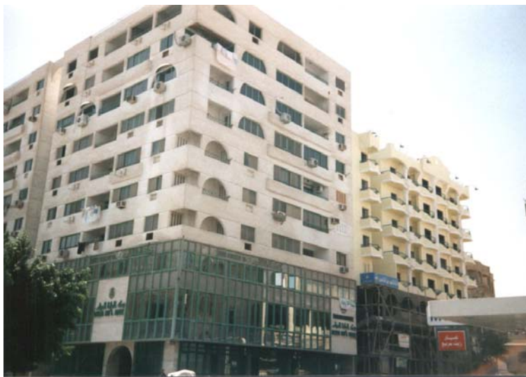
Figure 3-40 An attempt has been made here, with the new building, to lessen the disparity of height with its illustrious neighbour, by lining through with the ground floor level.
