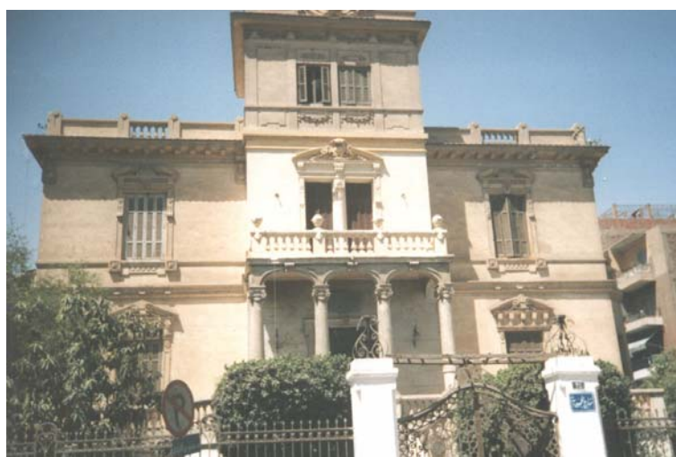
Figure 3-42 Facades have considerably less glazed areas. The mouldings, pilasters, cornices and other projections also provide partial solar protection to the openings and to the facade in general, especially for high angle summer sun around midday.
