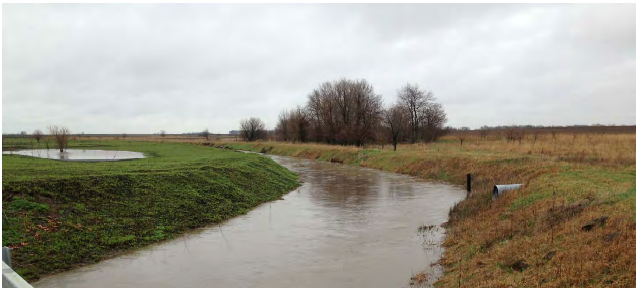
Fig. 10 - This photo from the CR 700E Bridge shows the only small wetland that was easily visible from a road. It is on the far right above the culvert in Big Ditch.
