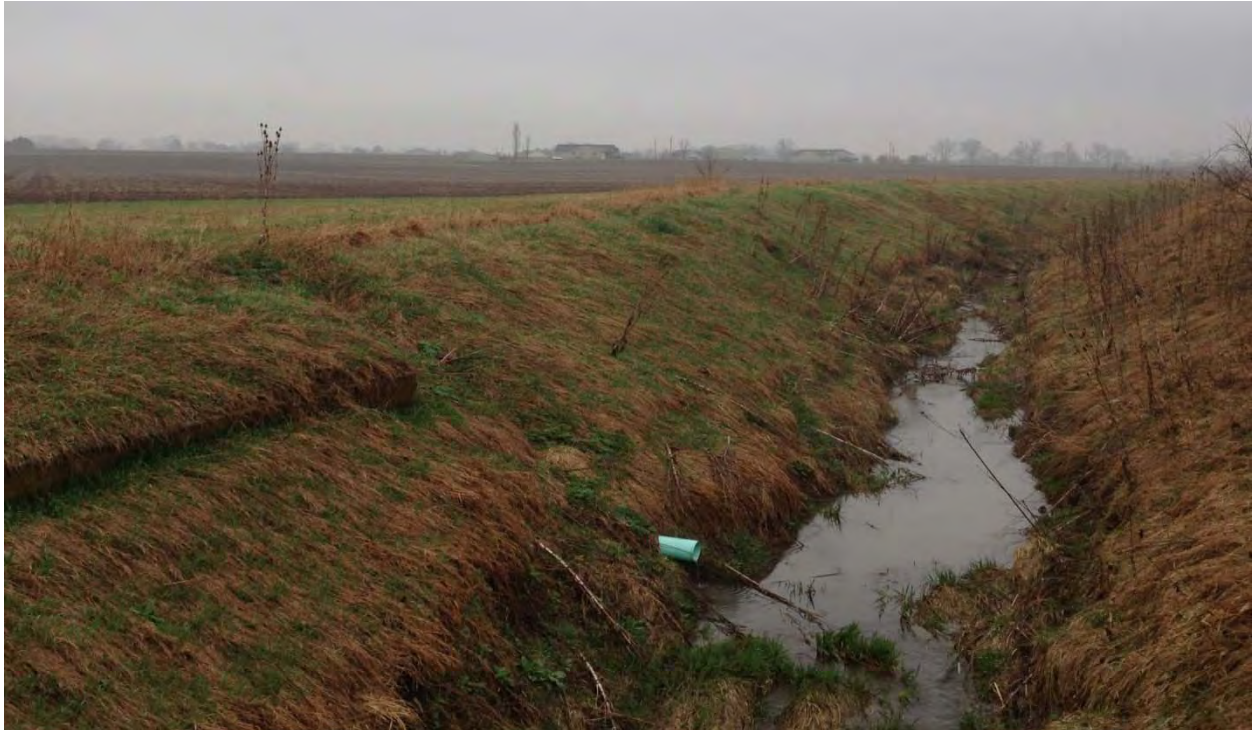
Fig. 14 - Subsurface drainage outlet on a tributary of Big Ditch
