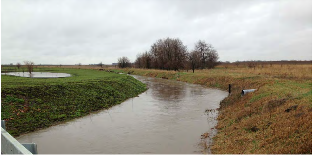
Fig. 7 - Big Ditch and floodplain from the CR 700E Bridge. Note the filter strip conservation practice on both sides of the water body. This was a common sight within the watershed.
