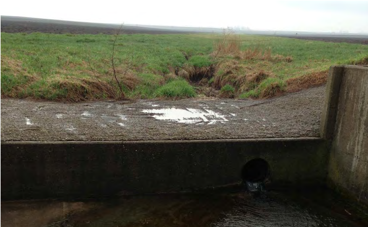
Fig. 24 - Drop notch structure at the base of a grassed waterway
