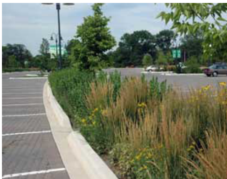
Permeable Paver Parking Lot with Depressed Islands
