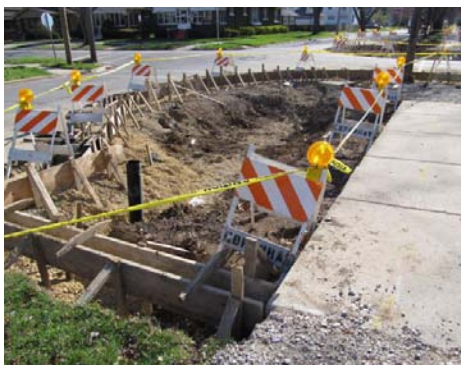
Rain Garden Bumpout Under Construction
