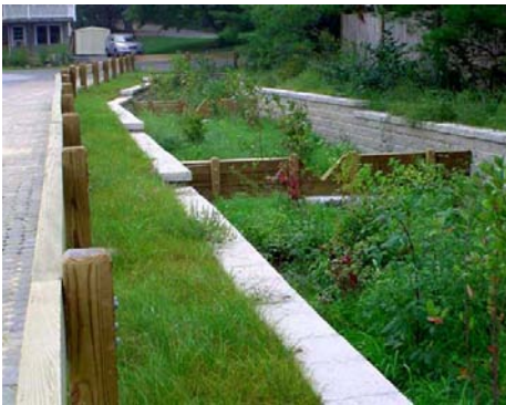
Terraced Vegetated Swale
