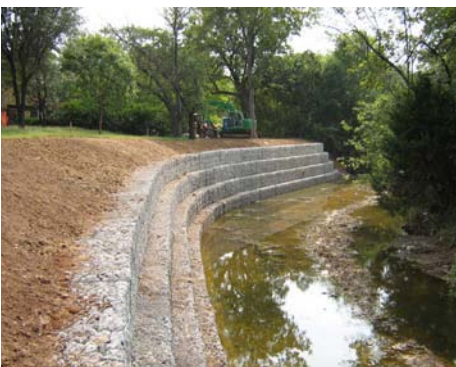
Gabion Bank Stabilization
