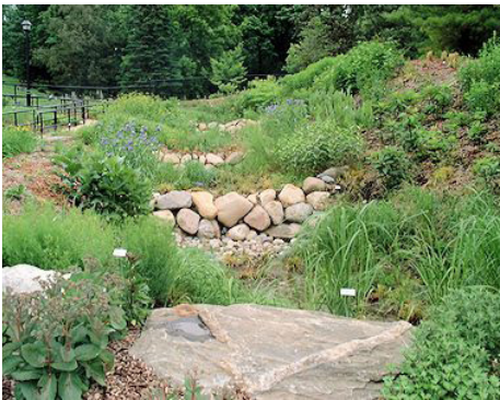
Terraced Vegetated Swale
