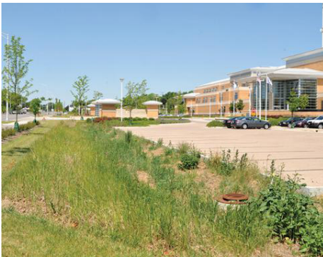
Bioinfiltration Collecting Runoff from a Parking Lot
