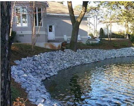
Rip-Rap Bank Stabilization
