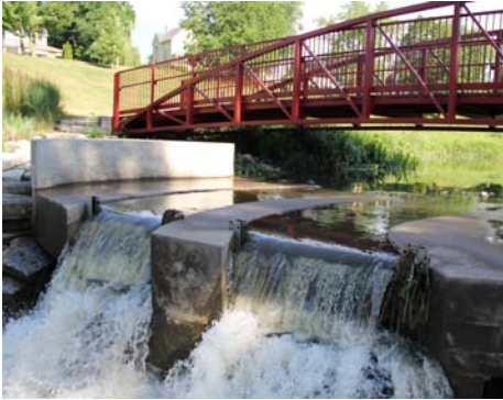
Water Control Structure
