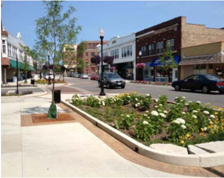
Urban Streetscape Rain Garden
