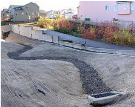
Bioswale Under Construction
