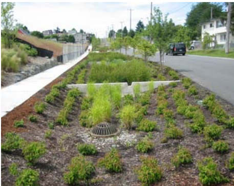
Terraced Bioswale
