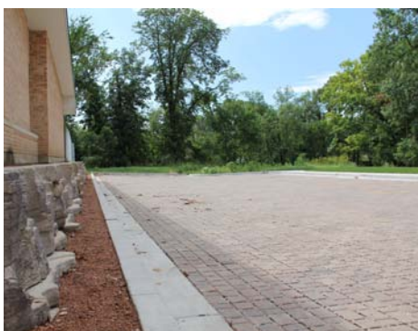
Permeable Paver Parking Lot
