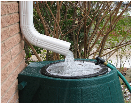
Rain Barrel Inlet Filter
