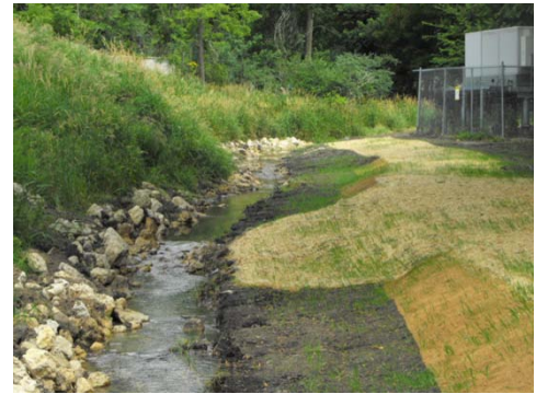
Figure 4-16. Carpenter Creek Stream Stabilization
