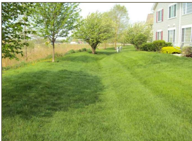
Figure 4-13. The existing 500-foot long swale between the two basins could be retrofitted by installing native plants and/or constructing an aggregate underdrain storage system. This would absorb and infiltrate polluted runoff from adjacent rooftops and side yards. (Source: Village of Carpentersville report prepared by AES)
