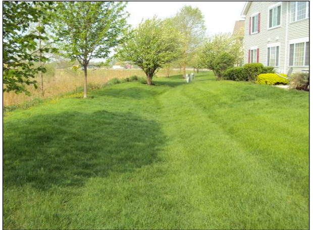
Photo 2: Swale between detention areas
