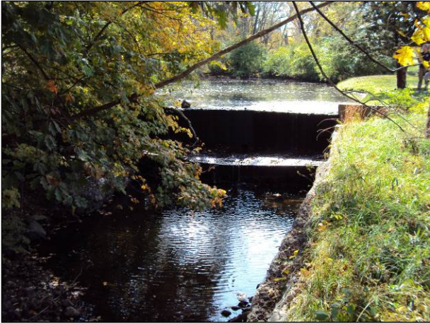
Photo 5: Dam at Fields Property
