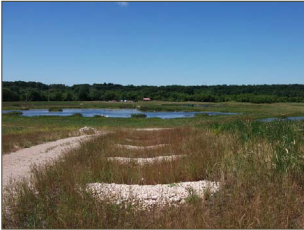
Figure 4-8. An example of rock checks previously installed elsewhere at the Jelke Bird Sanctuary along with a vegetated swale stabilized by native plantings. This approach could be used to stabilize eroding gullies and hillslopes in other portions of the project site.
