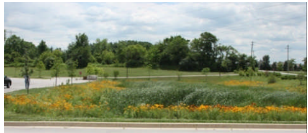
Figure 3-10. Wetland Detention Basin
