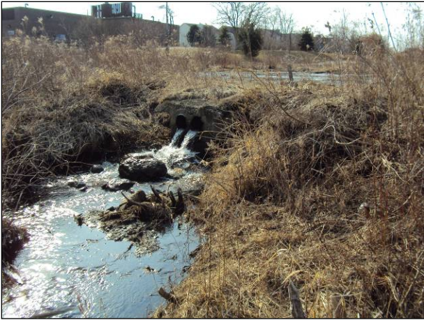
Photo 3: Old dam in Reach 2
