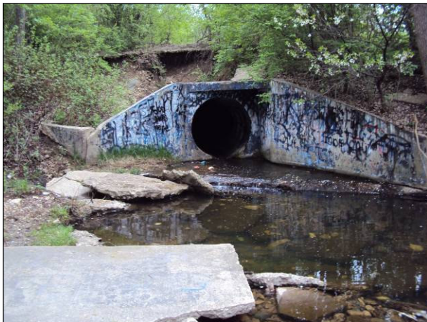
Photo 1: Culvert to Keith Andres Park
