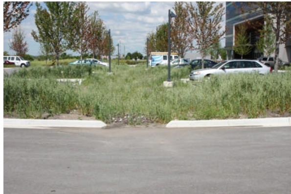
Figure 3-9. Bioretention in Office Parking Lot
