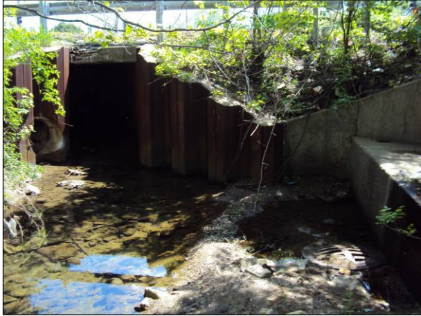
Photo 1: Culvert under N. Kennedy Dr.
