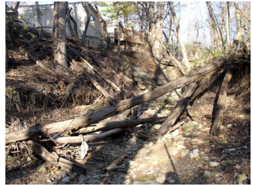
Figure 3-12. In-Channel Debris Accumulation
