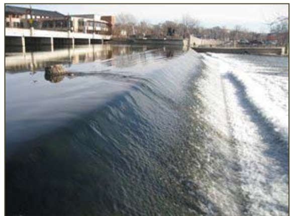
Figure 4-14. Elgin Dam across the Fox River.
