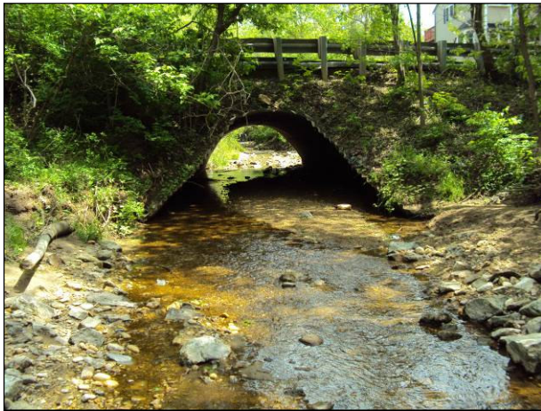
Photo 1: Culvert under Williams Rd.
