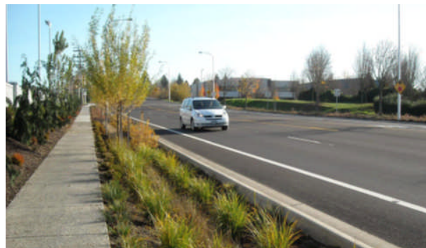
Figure 3-13. Arterial Roadway with Vegetated Swale and Porous Pavement Sidewalk ( Source: San Mateo County Sustainable Green Streets and Parking Lots Design Guidebook)
