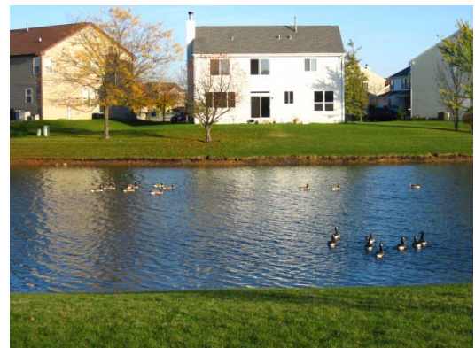
Figure 4-9. Traditional Wet Detention Basin with Canada Geese and Bank Erosion (Source: David Poweleit)
