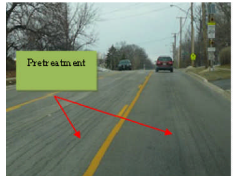
Figure 3-14. Pretreatment on Roadway
