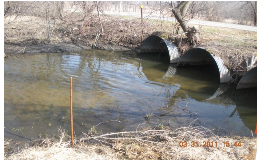
Figure 66. Culverts under Ames Road
