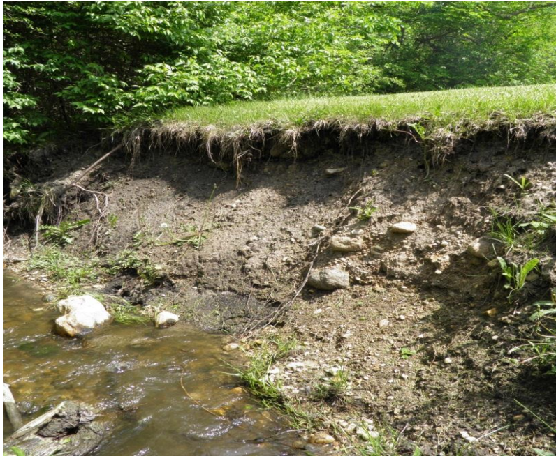
Figure 25. An area of high streambank erosion along the southwest branch of Sleepy Hollow Creek
