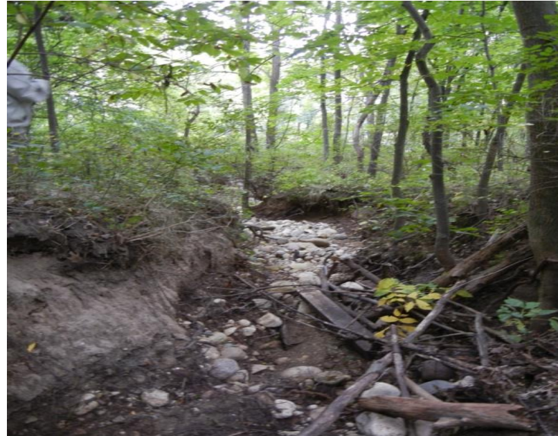
Figure 68. Erosion at the Oakwood Hills stormwater channel
