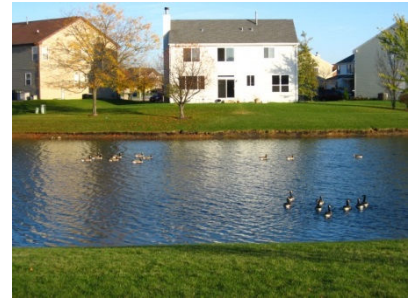
Figure 4.3 Traditional wet detention basin.
