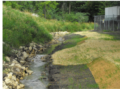
Figure 4.9 Example streambank stabilization project.
