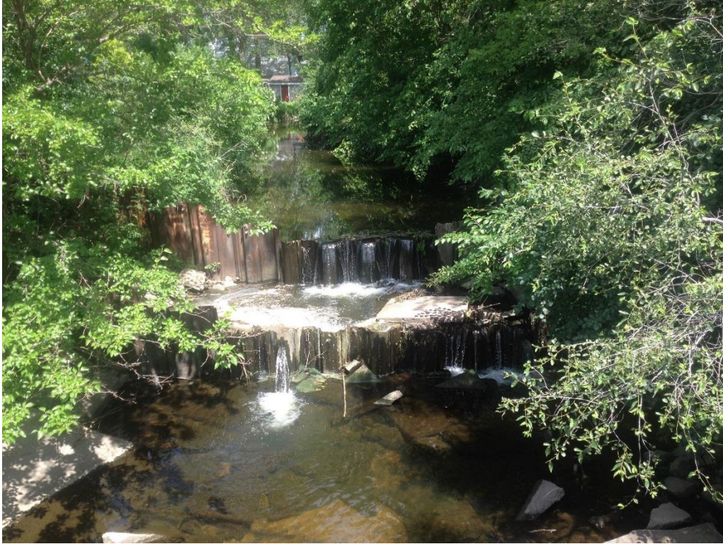
Figure 29 Sheet pile dam east of Belmont St.
