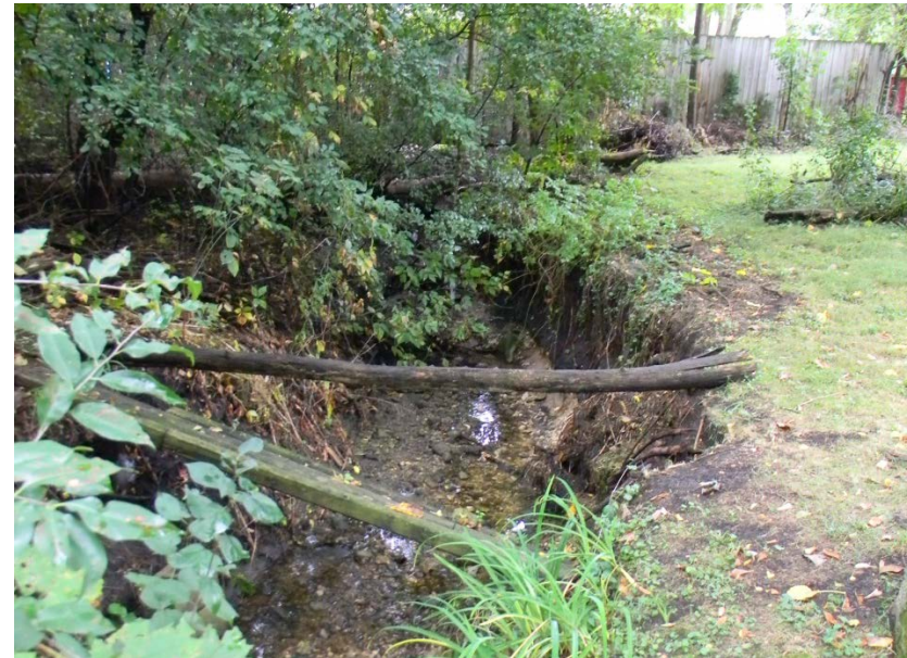
Example of highly eroded streambanks along State Street Creek Reach 3
