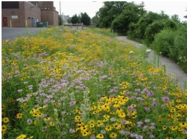
Filter strip along municipal building in Algonquin,
