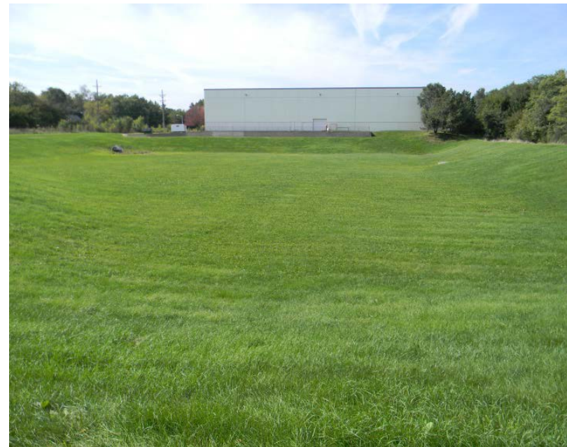
Typical dry bottom turf basin behind Sportsplex in State Street Creek watershed
