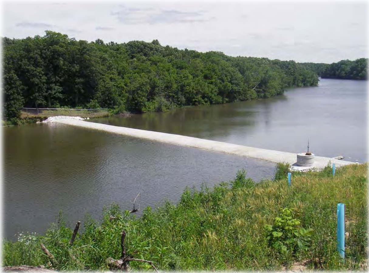
Low-flow/in-lake dam; Otter Lake, Illinois
