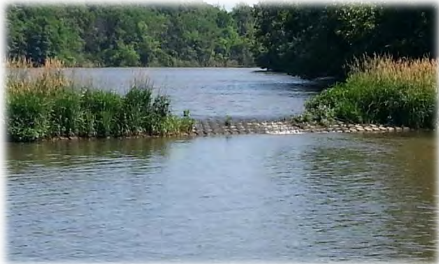
Low-flow/in-lake dam, Otter Lake, Illinois
