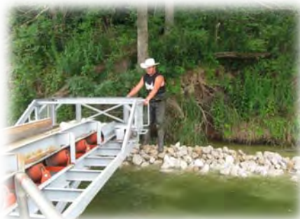
Application of Rock; Shoreline Stabilization
