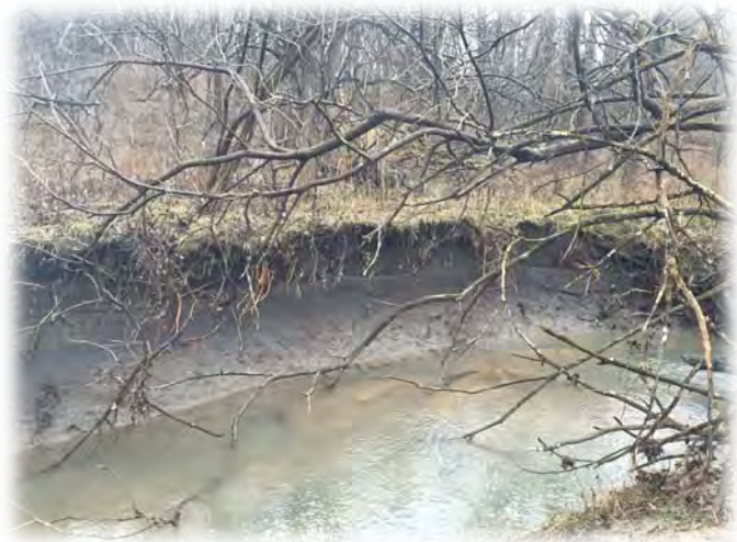
Woods Creek; High Bank Erosion
