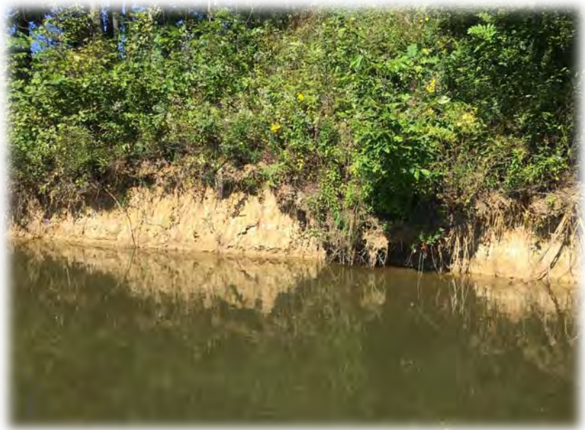
Franklin Lake Shoreline Erosion
