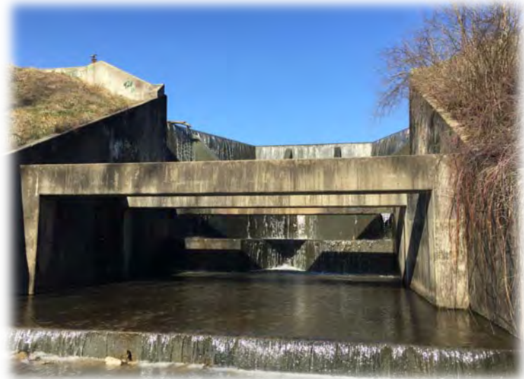
Waverly Lake Spillway
