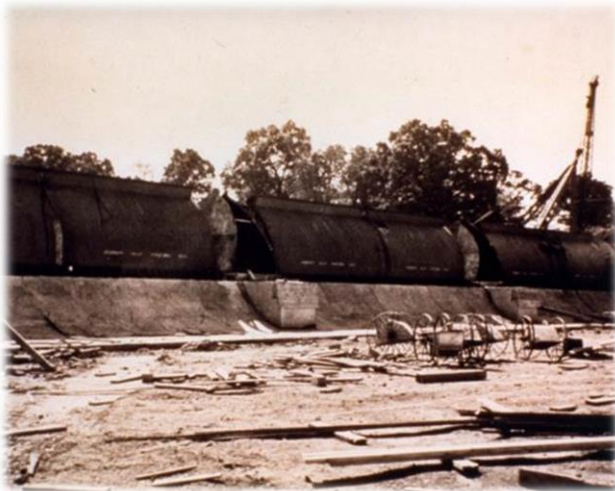
Spaulding Dam under Construction
