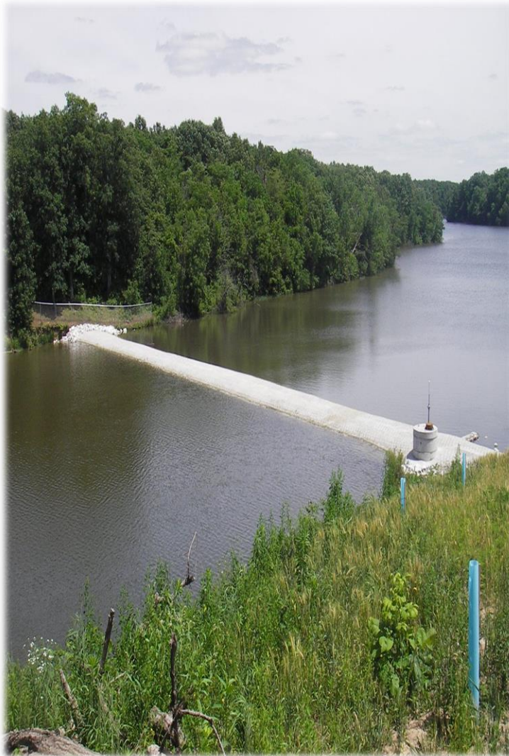
The Otter Lake Low Flow In-lake Dam
