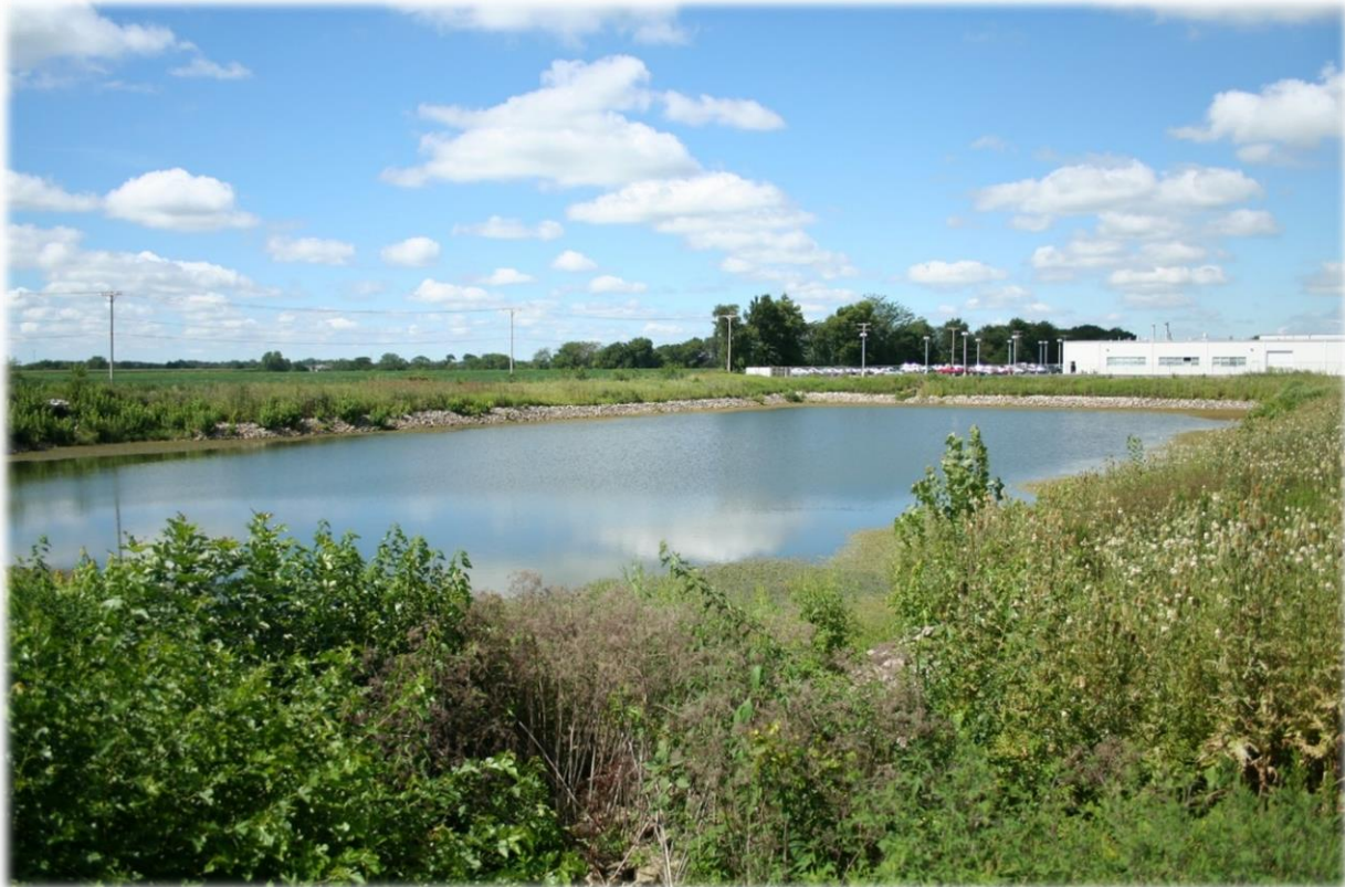
RETENTION POND IN LAKE SPRINGFIELD WATERSHED
