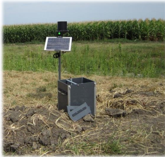
NEWLY INSTALLED DRAIN WATER MANAGEMENT STRUCTURE
