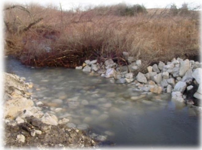
GRADE CONTROL STRUCTURES - ROCK RIFFLES
