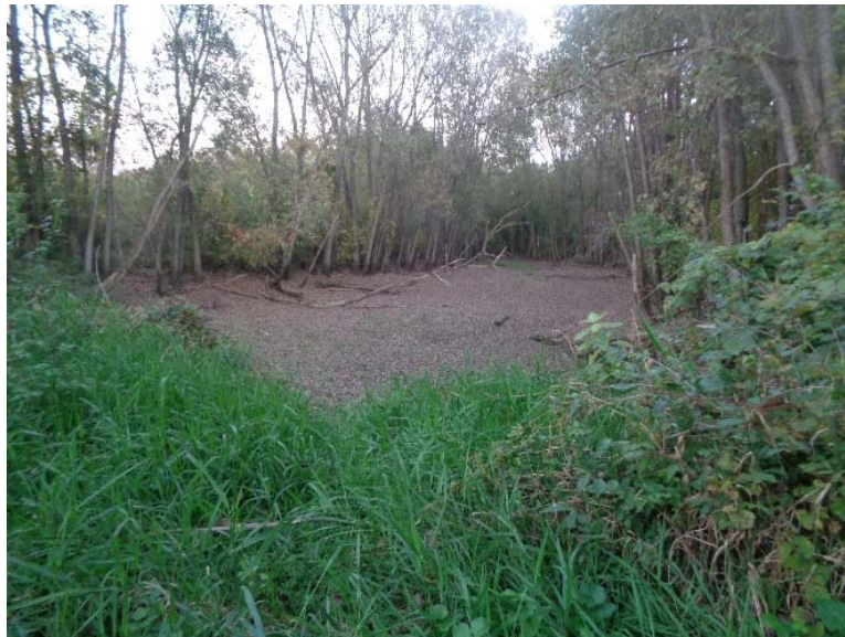
Figure 15 Detention pond upstream of Structure 13.
