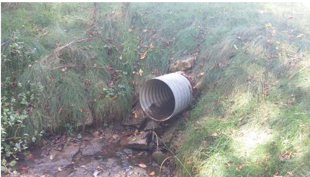
Figure 25 Outlet pipe of Structure 20.
