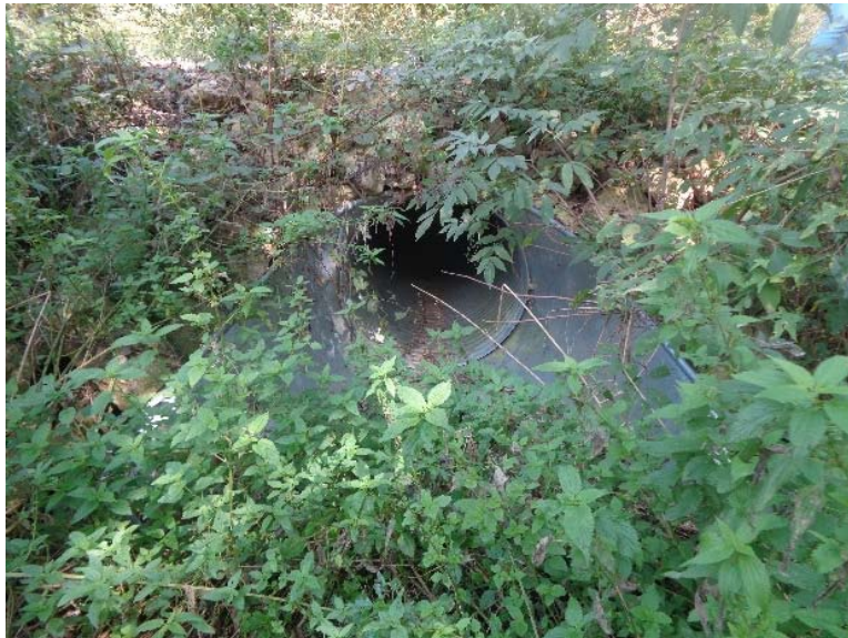
Figure 23 Culvert pipe at Structure 19.
