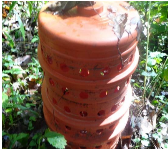
Figure 2 Exposed portion of Hickenbottom riser at Structure 2.
