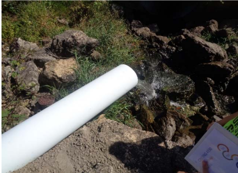
Figure 20 Outlet pipe structure 18.
