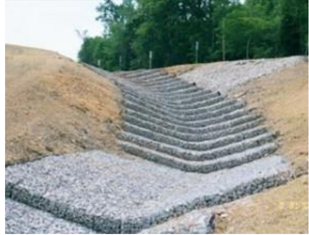
Figure 23. Gabion basket staircase (Quality Gabion Mattress for Slope Stability)
