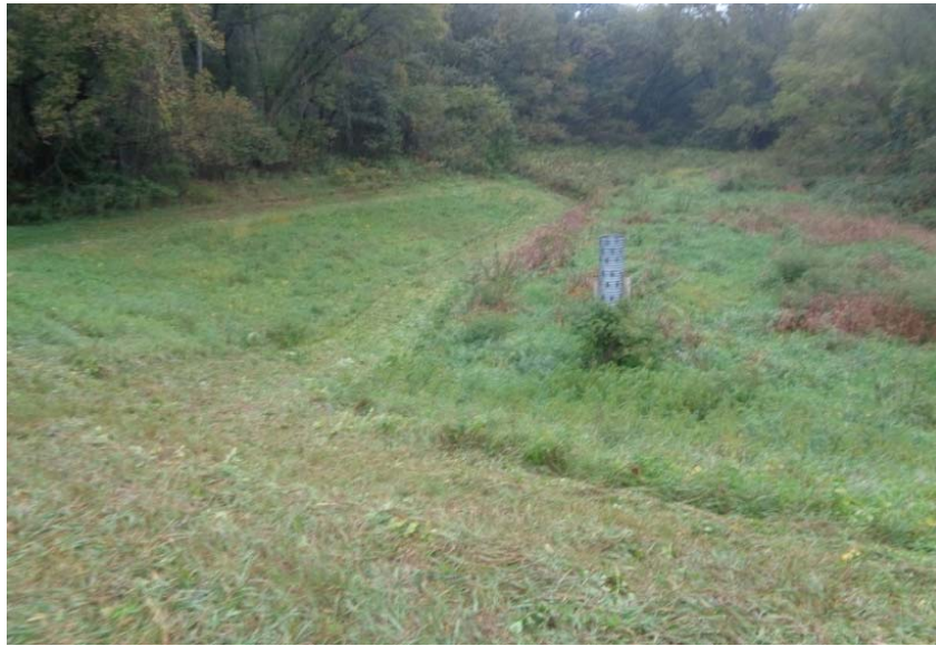
Figure 3 Corrugated riser at Structure 5.
