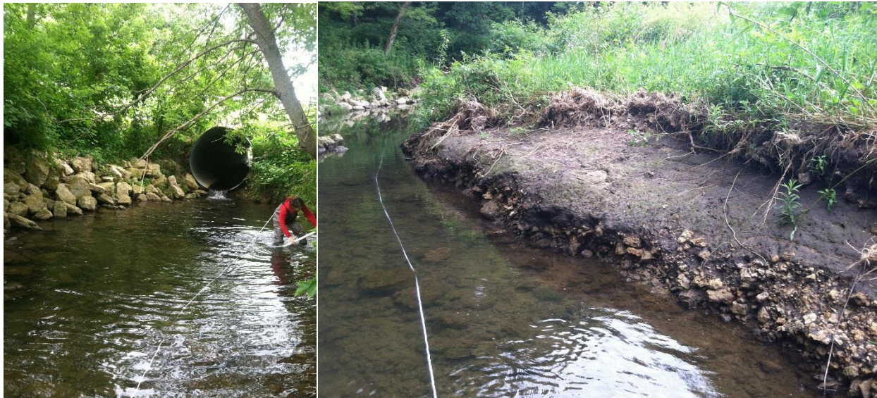
Figure 6-11. Erosion and bank condition in ID 1. Former bank is evident in these photos, however, spot treatment has not remedied larger issues.
