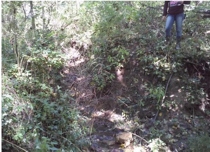
Figure 8. Site 1 bank erosion.
