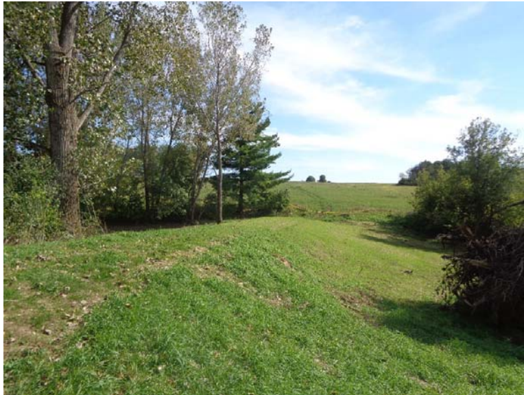
Figure 18 Structure 14 with two trees on left side of photo which may need to be removed.
