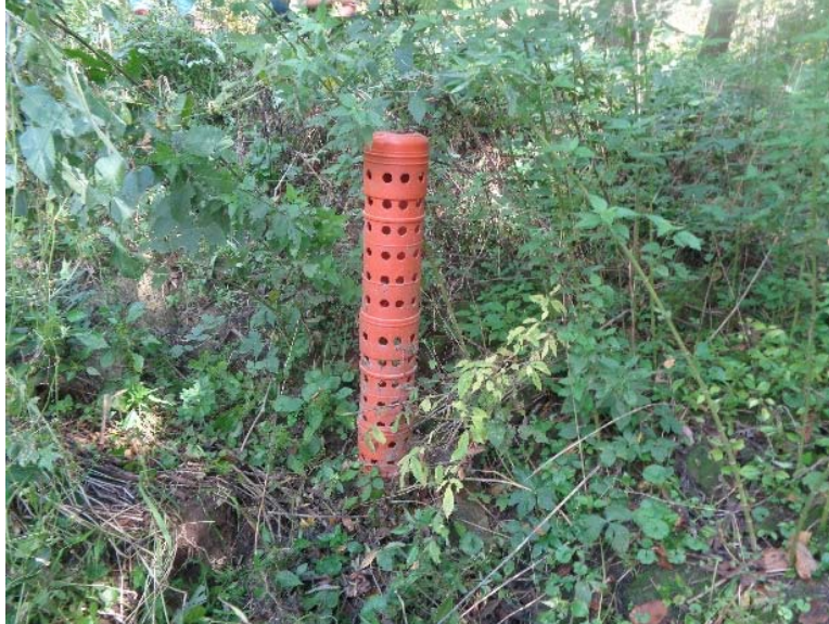
Figure 22 Hickenbottom riser at Structure 19.
