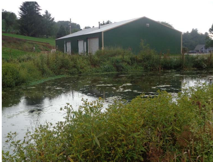
Figure 13 Structure 12 where all water collected flows into.
