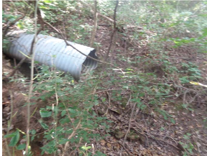
Figure 16 Outlet of culvert at Structure 13.
