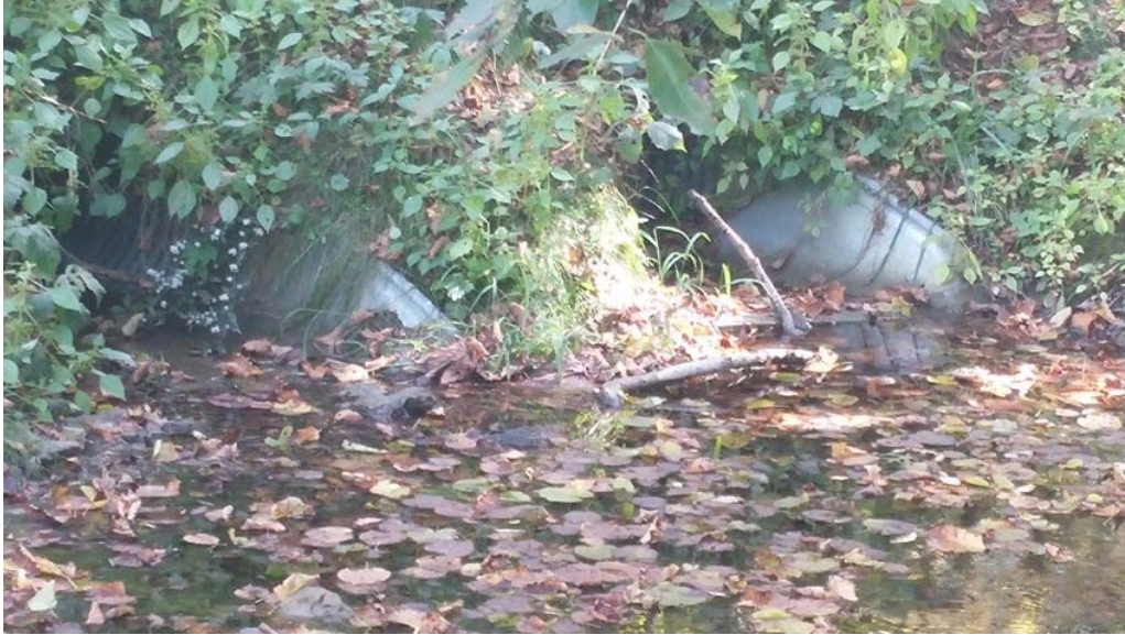
Figure 26 Culverts under the trail at Structure 20.
