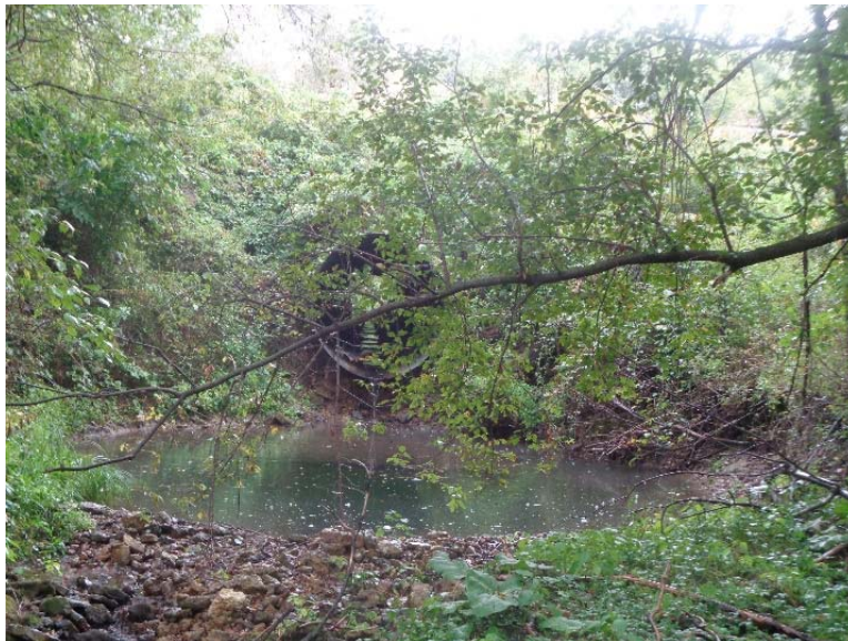
Figure 7 Culvert upstream of culvert 7 (under Lake Road).
