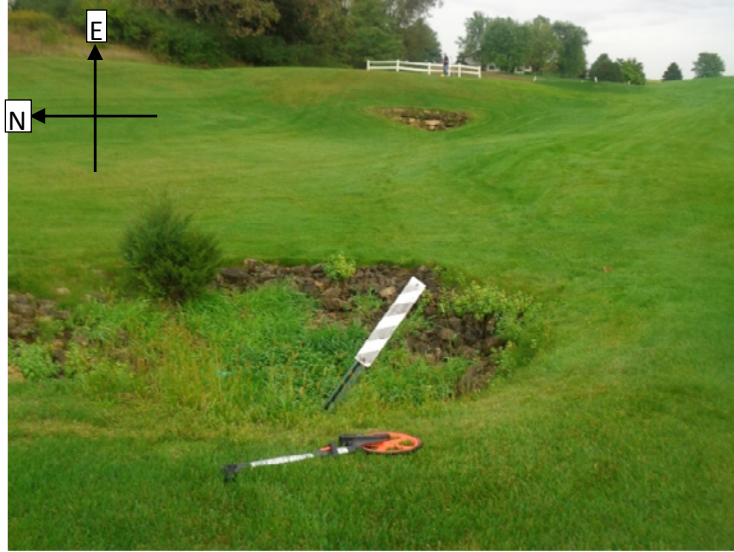
Figure 12 Culvert fed by two dry dams at Structure 12.
