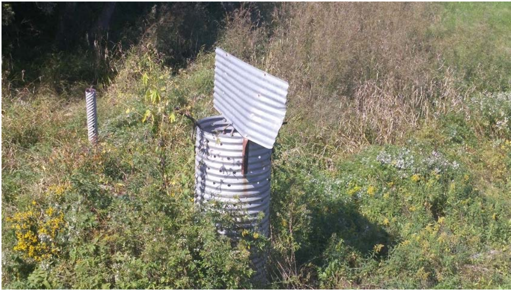
Figure 24 Upstream riser of Structure 20.
