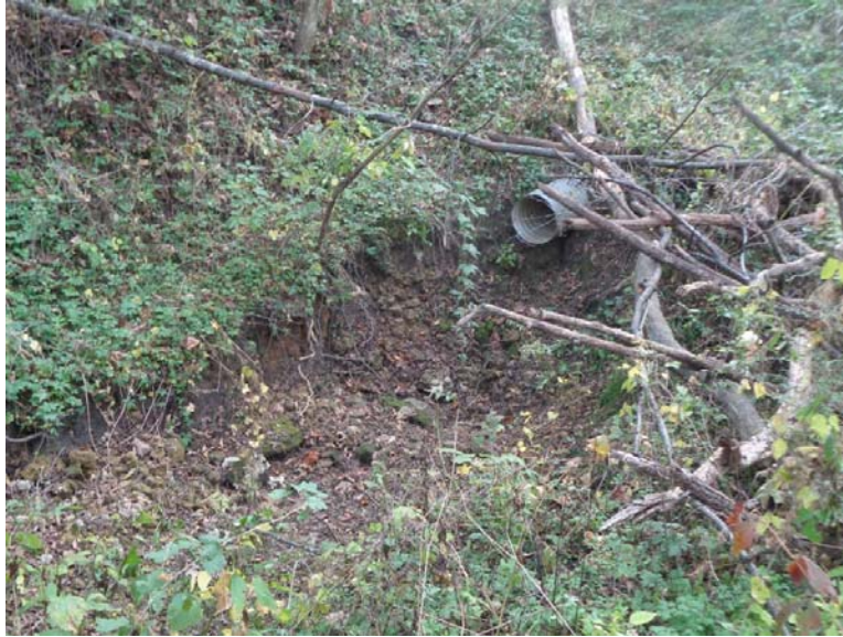
Figure 29 Downstream drop of corrugated pipe for Structure 21.
