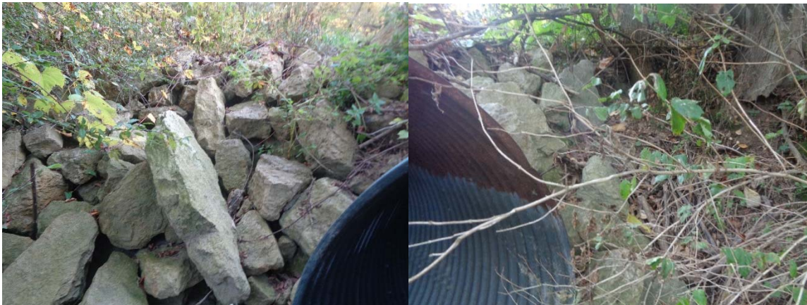
Figure 5 Comparison of riprap placement at culvert inlet in Structure 7.
