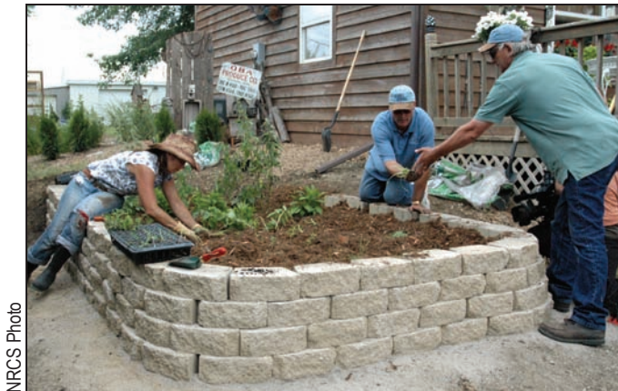
A retaining wall was installed to create a level rain garden on this sloping site in Madison County.
