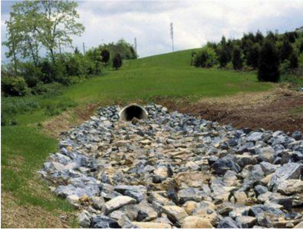
Figure 21. Riprap channel (Level 2).
