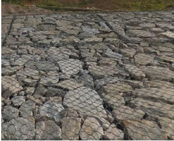
Figure 22. Up close view of gabion basket (Gabions Confine Stone For Erosion Protection and Retaining Soil).
