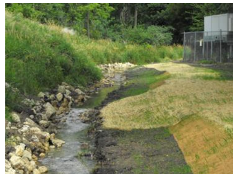
Example streambank stabilization project.
