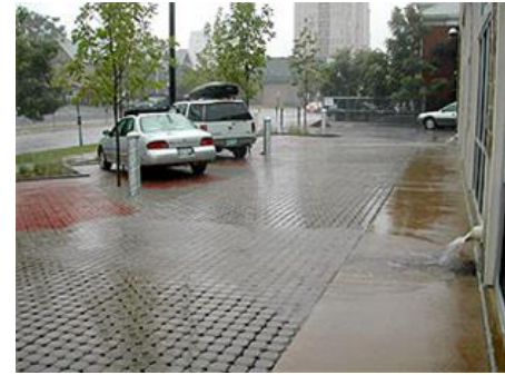
Example permeable pavement.
