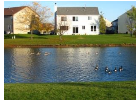
Traditional wet detention basin.
