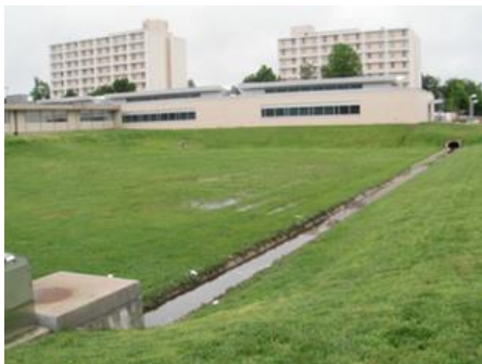
Traditional dry detention basin.
