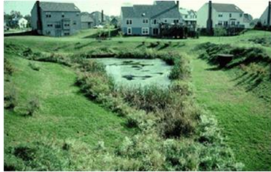
Example detention basin retrofit.
