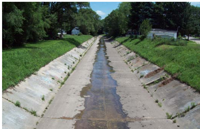
Figure 4: Concrete Drainage Channel
