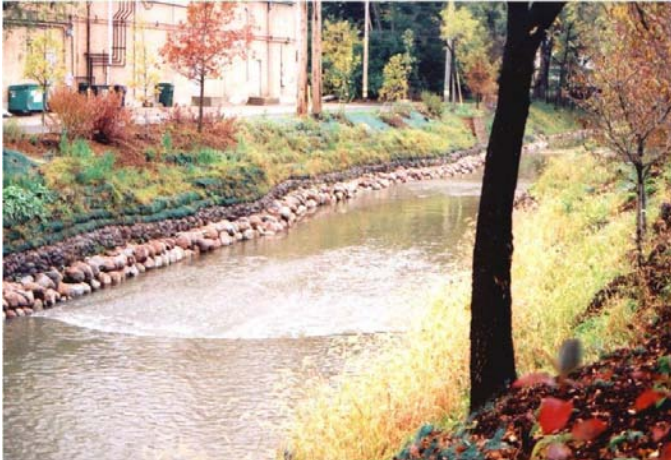
Figure 7: Stream Riffles/Slope Stabilization
