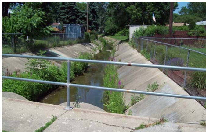
Figure 6: Concrete Drainage Channel
