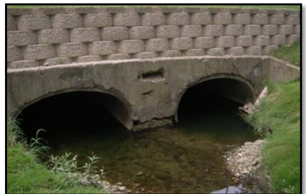
Figure 3-61: Culvert in Buffalo Creek Subwatershed
