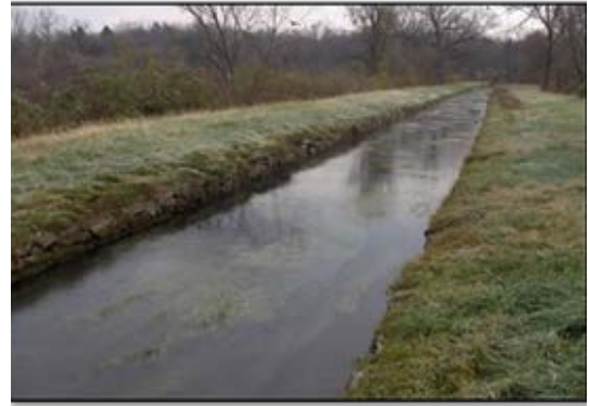
Figure 3-54: Channelization in the Newport Drainage Ditch
