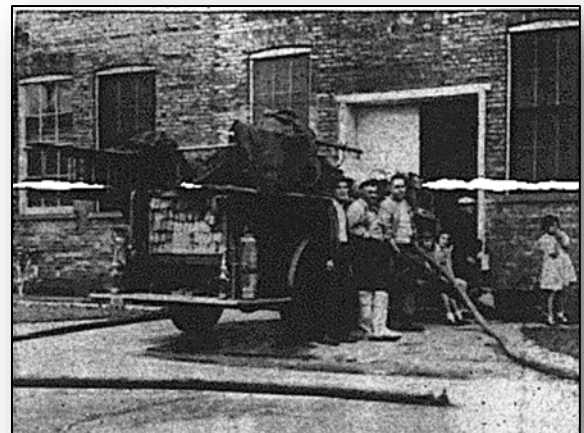
Figure 5-1: Libertyville Fire Department draining the Fould's Milling Co.
