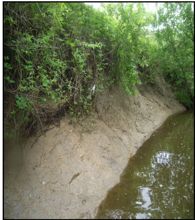
Figure 3-57: Streambank Erosion in North Mill Creek Subwatershed
