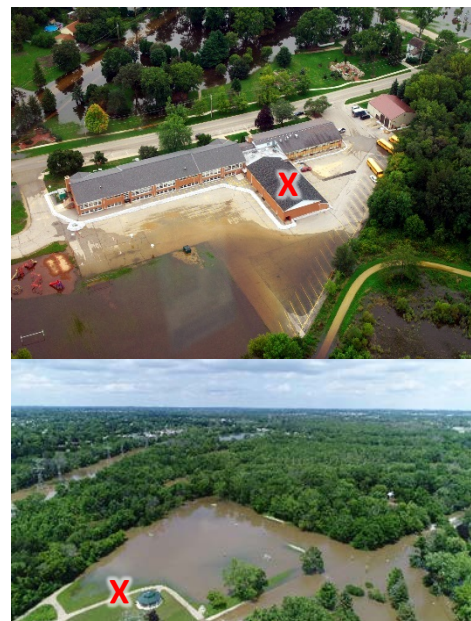
Figure 5-15: 2013 Gurnee Grade School flood mitigation site during flood events Before buyout looking south (top); after buyout and school removed looking north (bottom) "X" is the same spot on the site location
