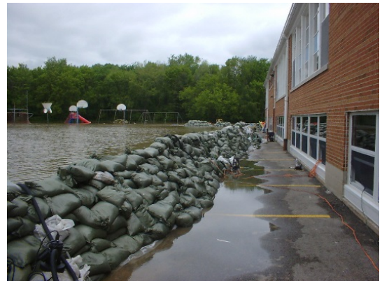
Figure 2-3: Sandbagging efforts to reduce flooding
