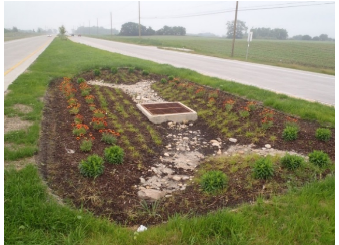
Figure 3-41: Roadway Reconstruction of Peterson Road from Route 83 west through Atkinson Road
