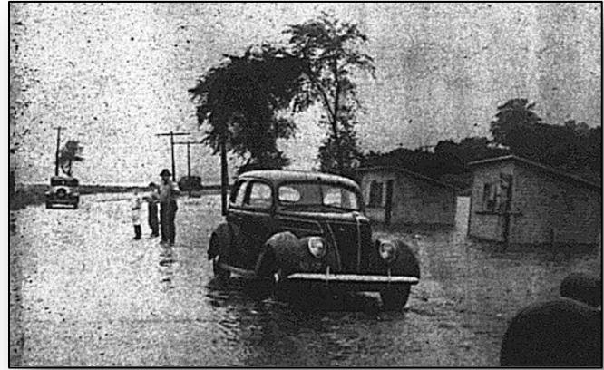
Figure 5-2: Butler Lake flooding of Lake Street
