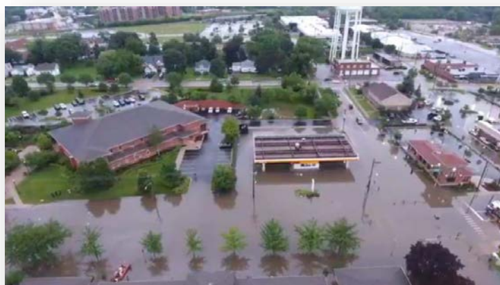
Figure 5-6: Flooding in downtown Mundelein
