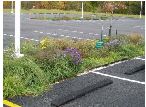
Figure 2-2: Parking lot bioswale with native vegetation
