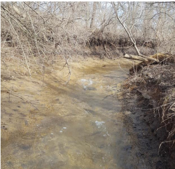
Photo 19: Headcut on Trib. 1 behind I-72 Rest Area
