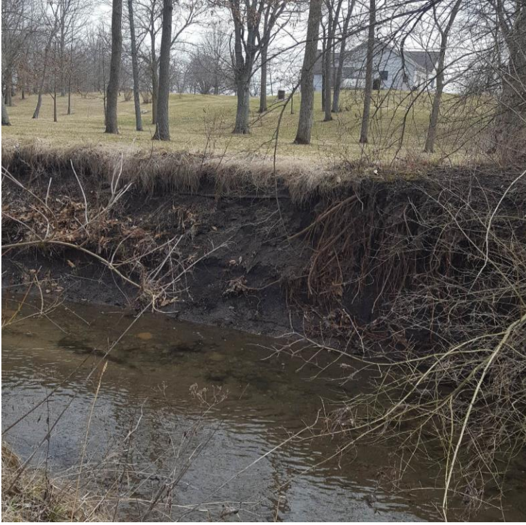
Photo 20: Severely eroding bank on Trib. 1 above Newburg Road
