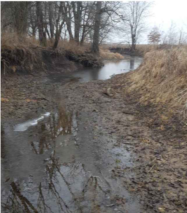
Phot 12: Friends Creek Ditch above Friends Creek Park. Stable bed but eroding banks are common. (Reach 002)
