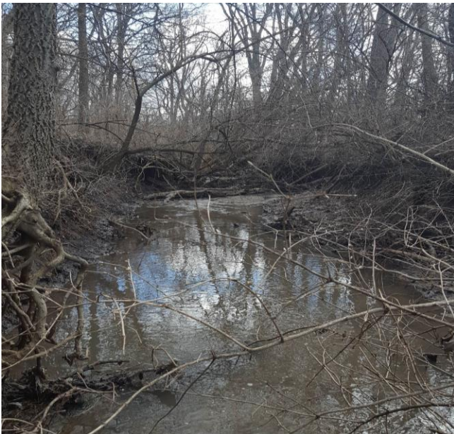
Photo 22: Both banks eroding severely on Trib. 2
