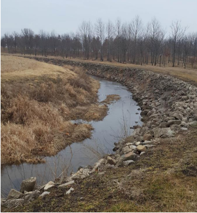
Photo 13: Friends Creek Ditch with 1600 ft. of riprap on the bank. (Reach 003)
