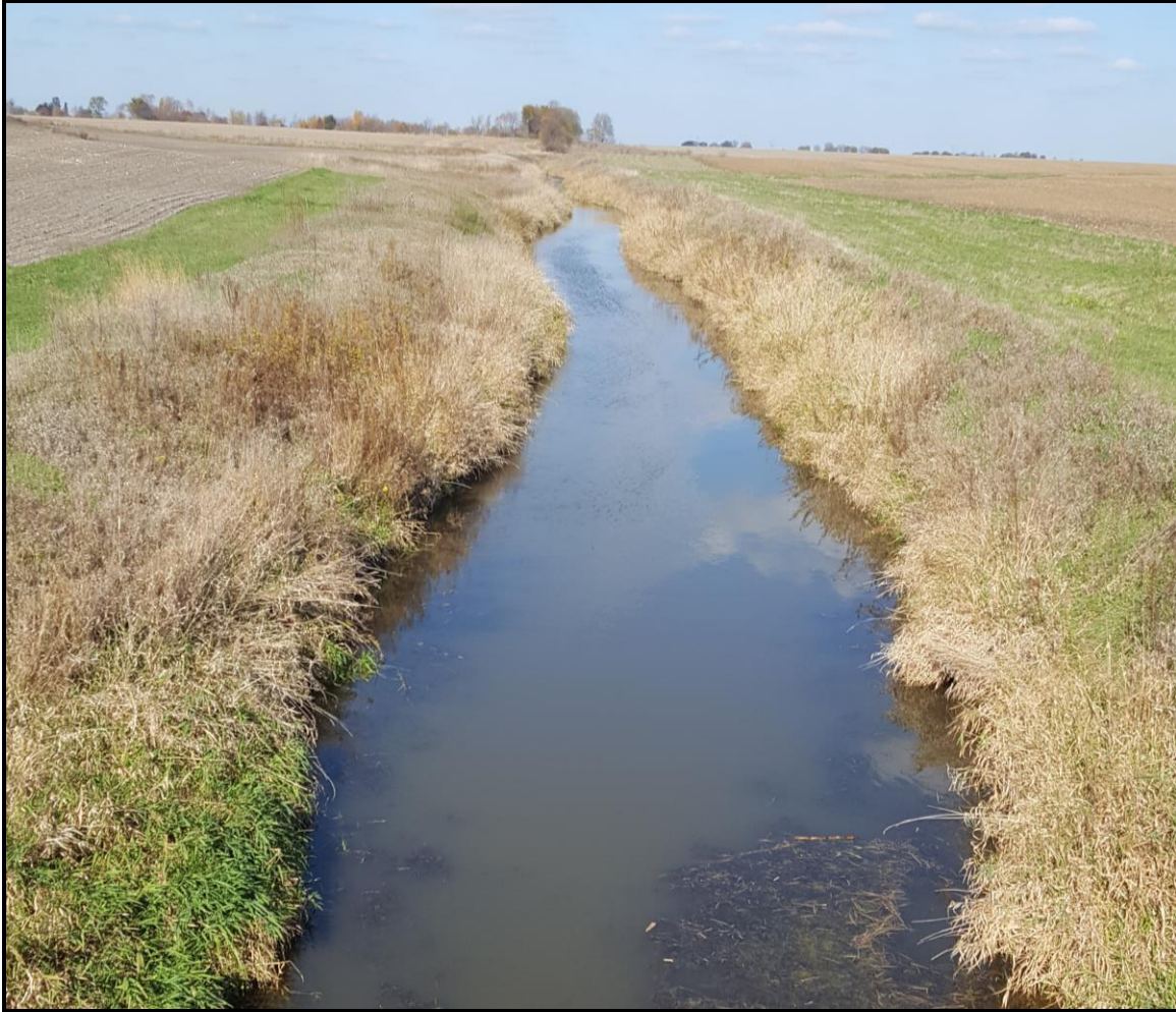
Exhibit 1---Slight Erosion: Typical of drainage ditch with vegetated banks. Little erosion, but good sediment transport of silt entering from outside the channel
