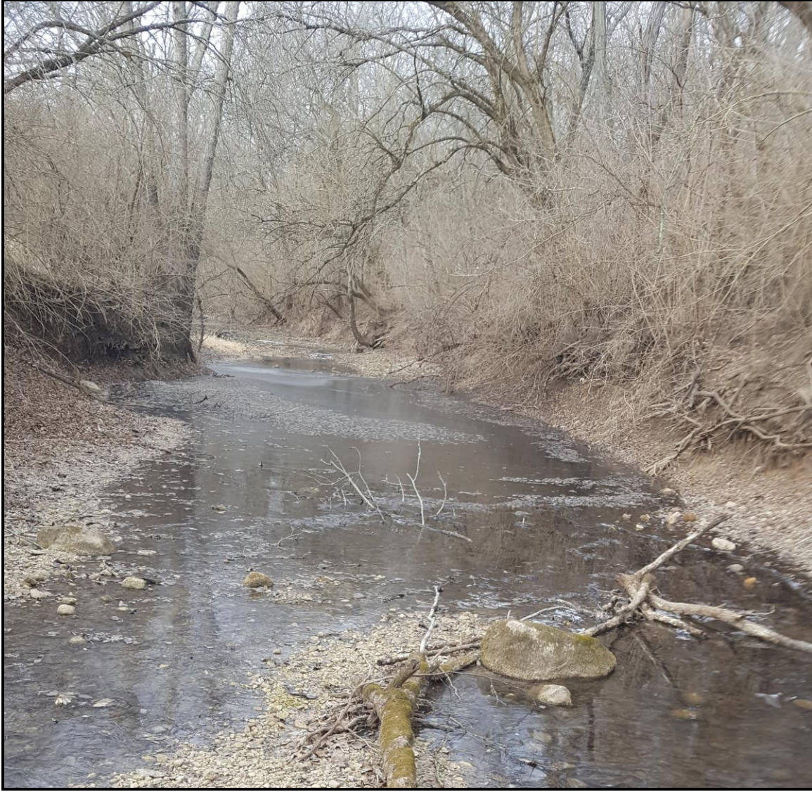
Exhibit 3----Moderate Erosion: Exposed tree roots, some bank overhang and trees leaning into channel
