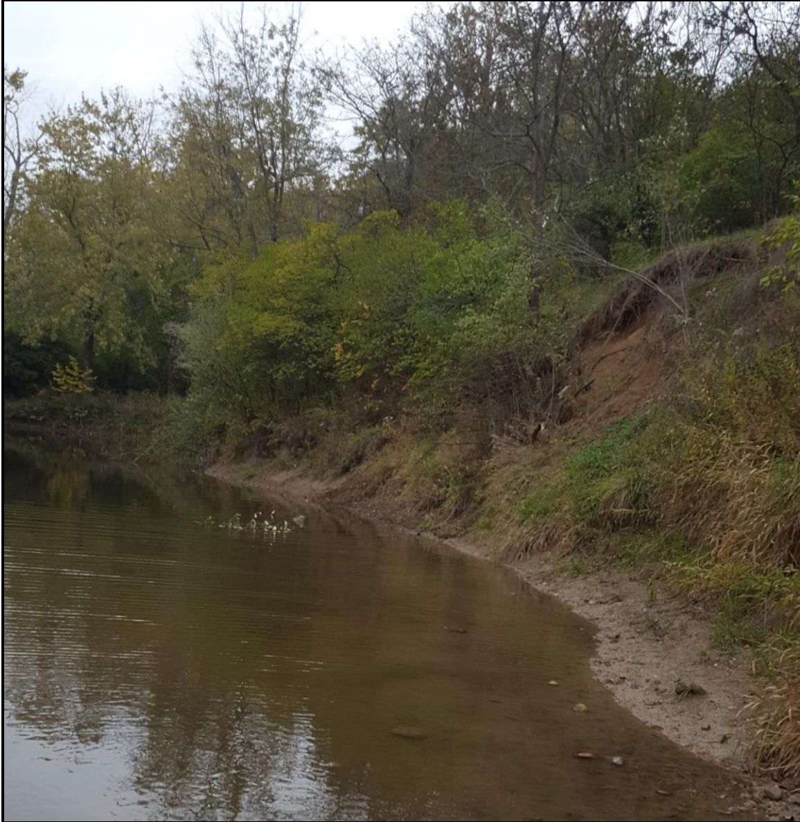
Exhibit 5----Very Severe Erosion: In channel cutoff below I-72. Bank slumping with material at base of nearly vertical slope
