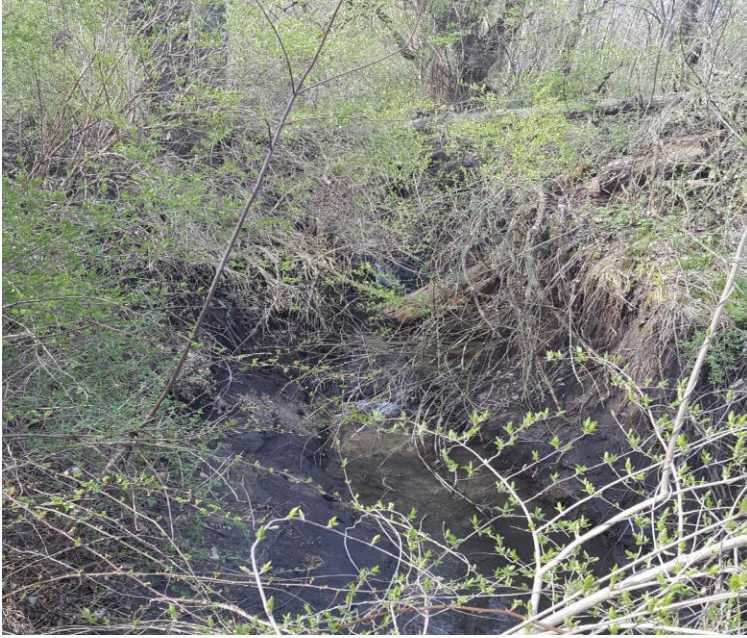
Photo 25: 3 ft. (+ or -) headcut midway up Trib. 3. Channel is 10 ft. deep and severely eroding.
