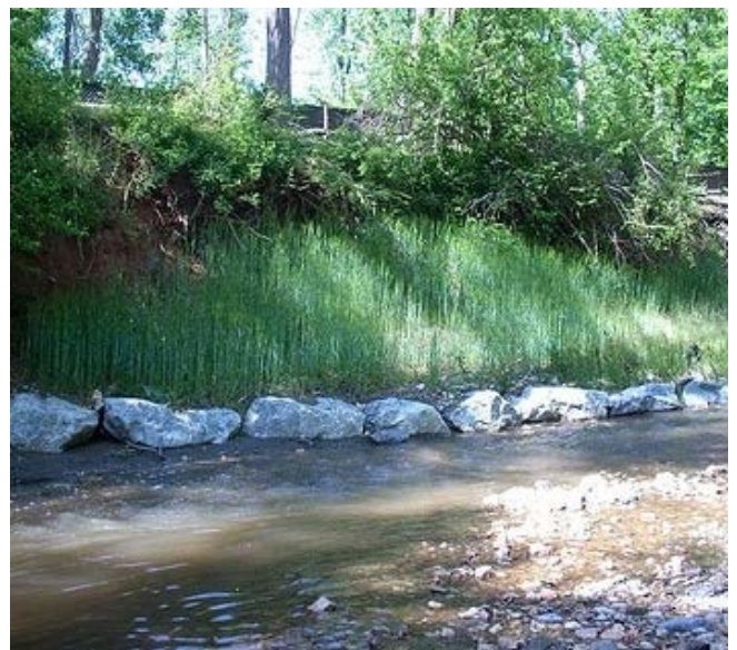
Stone toe protection, which prevents streambank erosion and shoreline erosion. Photo: Montgomery County, Maryland.
