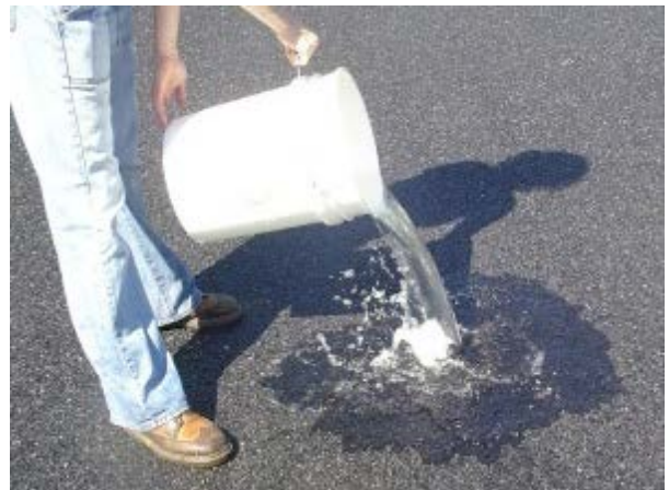
Pervious pavement. Photo: Philadelphia Water.
