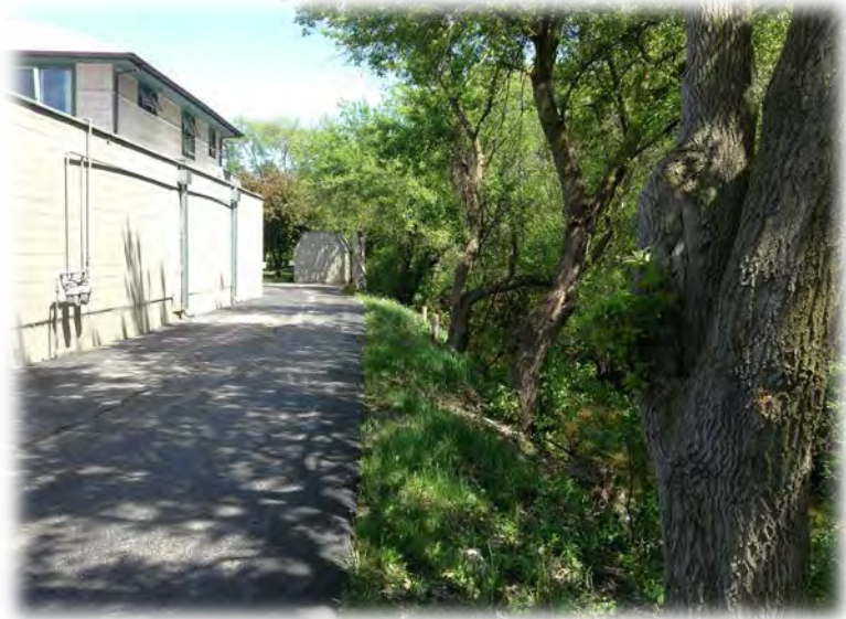
Photo 7-2: BMP SS38, Rain Garden/Gutter Control
