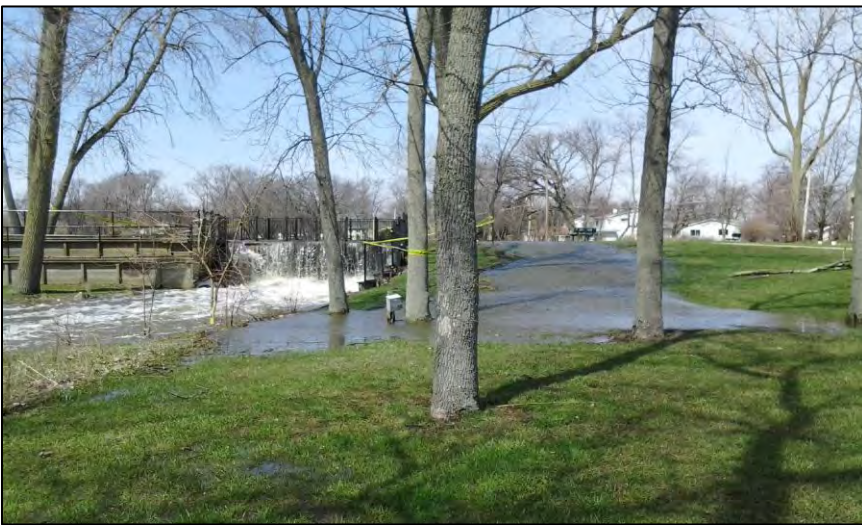
Photo 5-1: Grandwood Park dam overflowing from the March 20, 2013 rain event.
