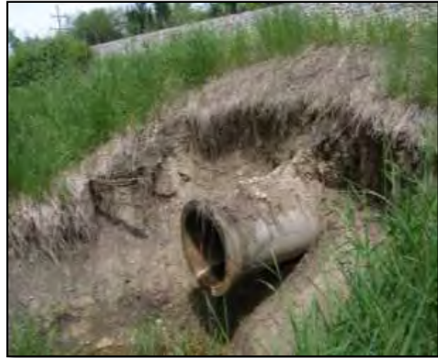
Discharge point in the Avon-Fremont Drainage Ditch
