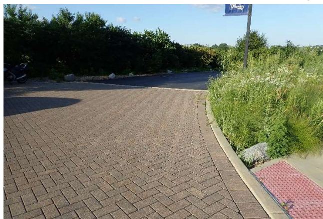
Permeable pavers at the St. Charles Park District's Hickory Knolls Discovery Center driveway and parking lot.
