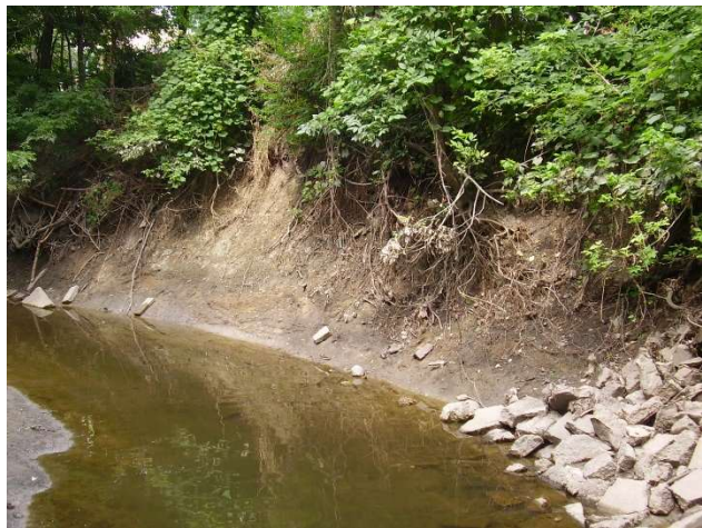
Photos 68 and 69: Severe channel erosion downstream of 5 th Avenue. Right Photo: Storm Sewer outfalls deliver runoff directly into Silver Creek, contributing to pollutant loading and scouring.
