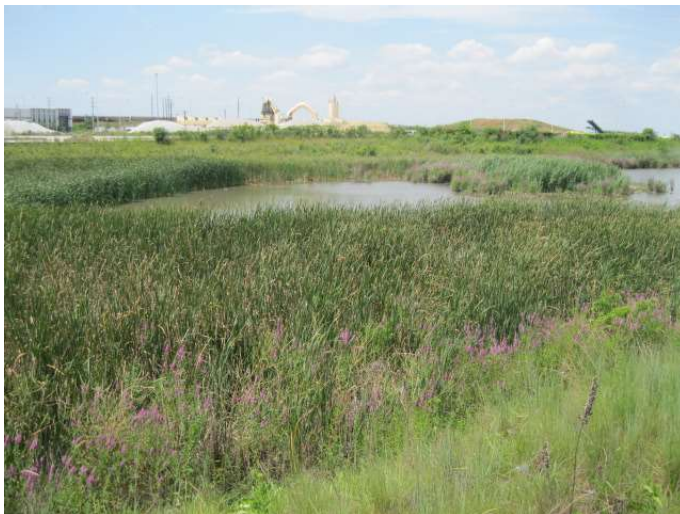
Photos 89 and 90: The O'Hare Airport (left photo) online detention areas previously described (see also Photos 16 and 17) has emergent wetland shoreline vegetation. This along with the open water area provides areas for settling and removal of nutrients and solids from upstream areas. On the negative side, online basins directly on the creek can reduce dissolved oxygen levels and increase water temperatures in the creek. Right Photo: A separate meandering "off-line" creek channel separate from a runoff storage basin during normal baseflow conditions can be constructed to improve water quality. During flood events, the creek overflows into the storage basin for a comprehensive BMP (Source: Living Waters Consultants, Inc.)
