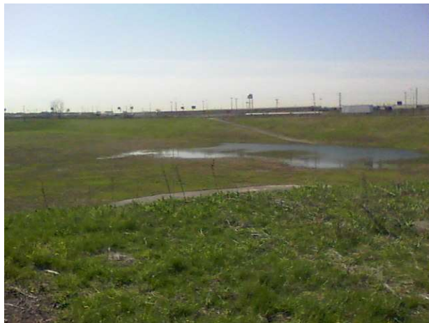
Photos 18 and 19: The MWRD Basin (left photo) contains some surface water storage at the bottom of the facility. The facility is overall managed to be pumped relatively dry. Mowed turf grass is dominant along the tall side slopes of the 36-acre facility. Silver Creek (right photo) flows below ground and does not interface with the MWRD Basin except during extreme flood events. Both facility modifications and operational modifications would be needed in order for the existing basin configuration to be allowed to provide improved water quality benefits along Silver Creek.
