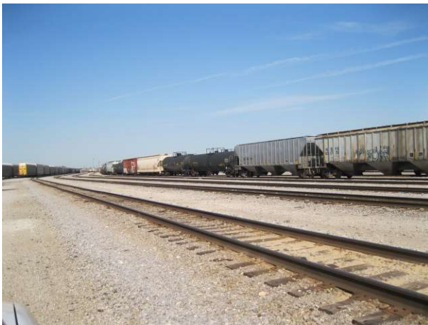
Photos 24 and 25: The Canadian Pacific railroad yard reach contains extensive gravel areas (left photo). The gravel materials improve potential runoff infiltration, provides at least limited filtering of oil, grease, or other materials, and reduces potential runoff volume into Silver Creek. The south parcel of the railroad yard contains office building, parking, and other impervious surfaces. Perhaps the most significant concern (and opportunity for water quality improvement) is the ditch approximately 4,500 LF in length along Franklin Avenue. This non-vegetated ditch contains significant bank erosion, rills, and gullies. During the site visit, vegetated along the ditch was being herbicided (we are uncertain if rock improvement is being proposed along the ditch.) Sediment deposits in the channel bottom are extensive. This ditch is periodically dredged to remove sediment deposits.
