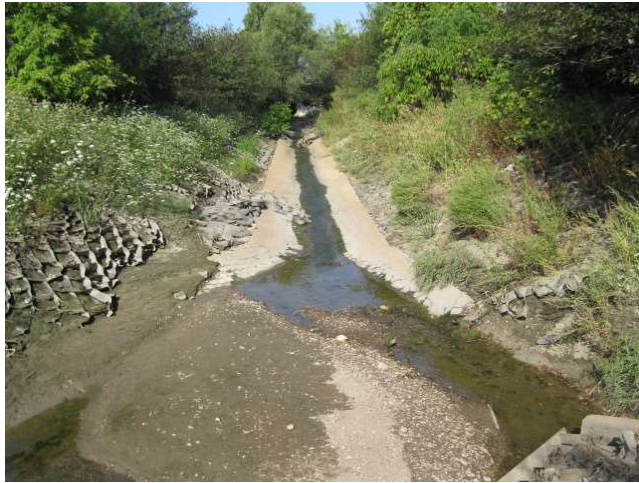
Photos 22 and 23: The small runoff collection basin receives storm pipe inflow from the railroad yard. During major flood events, flood waters are not detained long, but are pumped out with large capacity overhead pumps (right photo) into Silver Creek when the flood stage recedes.
