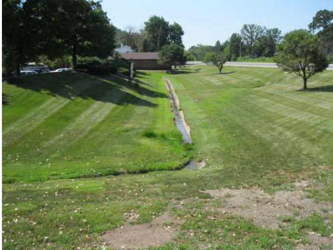
Photo 88: This mowed turf detention area (Basin 2.A) in a multi-family residential development has a low-flow concrete channel in the bottom of the basin. Impervious surfaces such as concrete increase the rate and velocity of discharge of runoff from the basin, and prevents the infiltration of runoff into the ground. This site receives some runoff from Rt. 83 during flood events.
