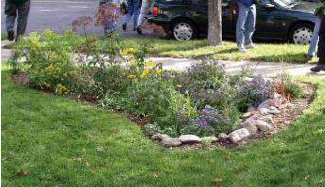
Photo 118: Residential areas can also contain rain gardens to filter runoff before discharging into storm sewer systems at the streetside area.
