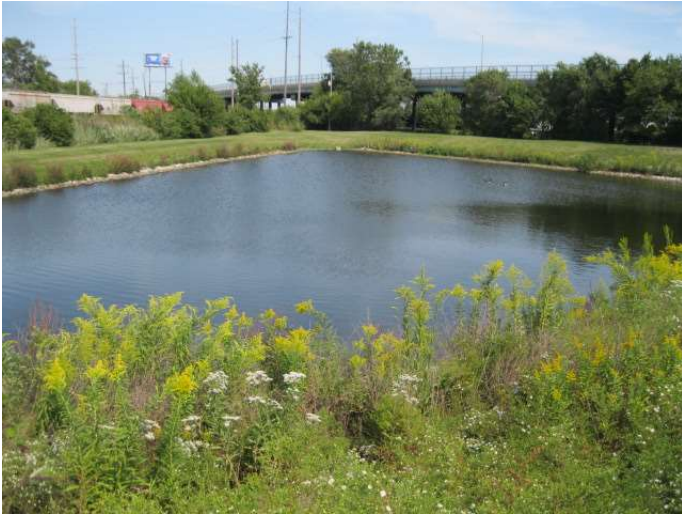
Photo 95: Industrial detention areas vary widely in condition. Some have no shoreline vegetation. Some are located immediately adjacent to large parking lots or other paved surfaces. Basin # 16.A. depicted contains a mixture of mowed turf grass and taller native plantings (foreground).
