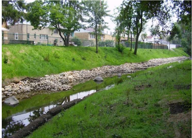
Photos 64 and 65: Before and After Construction of the Phase 2 Silver Creek Stabilization Project completed in 2008 by the Village of Melrose Park, near 5 th Avenue. Rock toe, rock points, and re-shaped slopes with native plantings are depicted. Mature willow trees that had been falling into the channel were selectively removed. Native plantings are maintained annually, which is an important ingredient for their establishment and longevity.
