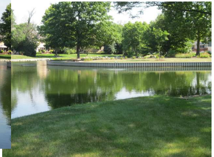
Photos 83 and 84: An unnamed lake (Basin 1-B) with residential areas along the shoreline contains extensive turf grasses at the shoreline with a variety of shoreline stabilization treatments ranging from retaining wall, to rip-rap, to re-shaped turf slopes. It is likely that turf grass pollutant runoff contributed to algae blooms that appear to be present.
