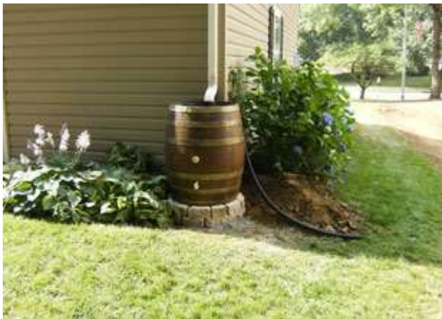
Photo 117: Residential areas can be equipped with rain barrels to reduce runoff volume.
