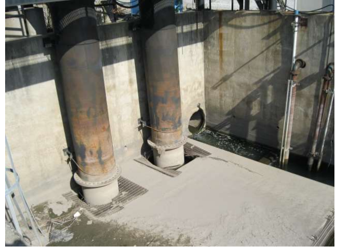
Photos 22 and 23: The small runoff collection basin receives storm pipe inflow from the railroad yard. During major flood events, flood waters are not detained long, but are pumped out with large capacity overhead pumps (right photo) into Silver Creek when the flood stage recedes.
