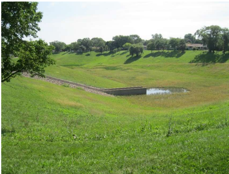
Photo 94: Water levels in the reservoir are pumped out to provide flood storage capacity. This basin could be modified to improve water quality by installing native plant side slopes. (Note: Some communities such as Franklin Park have ordinance restrictions on plant heights.) Other improvements could include constructing a wet detention basin, a meandering low-flow creek corridor, and/or wetland habitat within the basin. Unfortunately, at present Silver Creek flows are not routed through this basin, except during flood flows. Therefore, no consistent water quality improvement occurs at this time. This is significant in part because the Silver Creek corridor adjacent includes some of the most degraded reaches in the entire watershed (See Photos 35 through 39).
