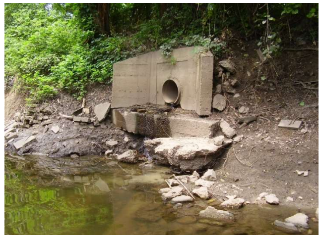
Photos 68 and 69: Severe channel erosion downstream of 5 th Avenue. Right Photo: Storm Sewer outfalls deliver runoff directly into Silver Creek, contributing to pollutant loading and scouring.
