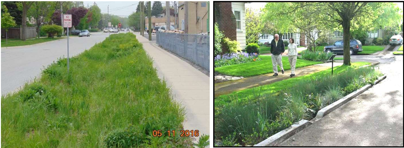
Photos 100 and 101: Urban bioswales can be retrofitted along street rights-of-way to significantly reduce runoff volumes and associated pollutant loading. Signage can help to educate the public.
