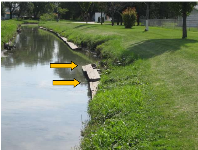
Photos 44 and 45: In some locations, lunker boxes are highly scoured. Turf grasses predominate. Right Photo: Interestingly, a side-channel walking path, the "Silver Creek Trail," allows residents to view the open stream channel condition.
