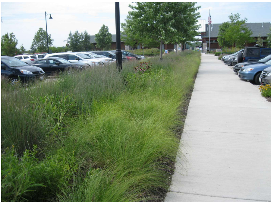
Photo 106: Installation of a linear bioswale with native plants in a setting with expansive parking lots.
