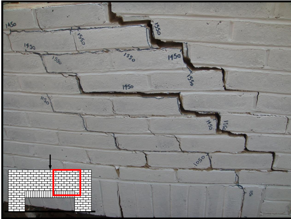
Fig. 14. View of the right hand side of the panel.
