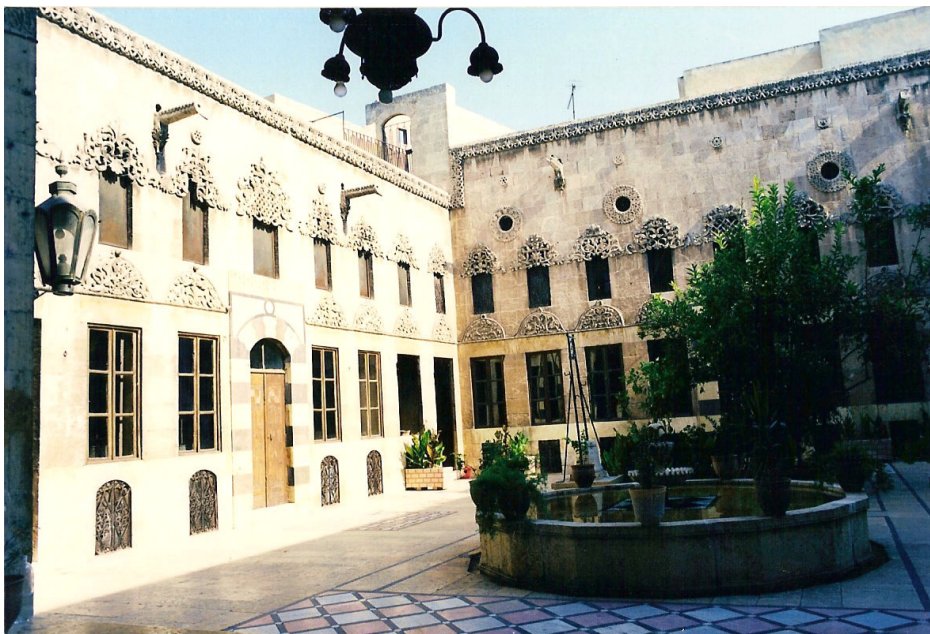
Figure 4.3. The Courtyard house in Jdedieh district as introverted
