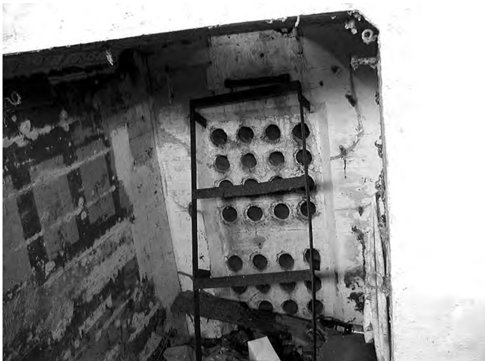
Lower level of the Wilridge (Kirkpatrick) BCS, showing niche for the Mk XX naval computer. Holes in the back wall are conduits for data transmission and power lines. Author, 2002
