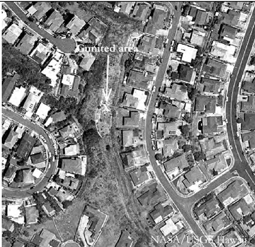
View of the site believed to be the location of Battery Salt Lake (Burgess). Arrow points to large gunned area on the inner aspect of a small crater. USGS
