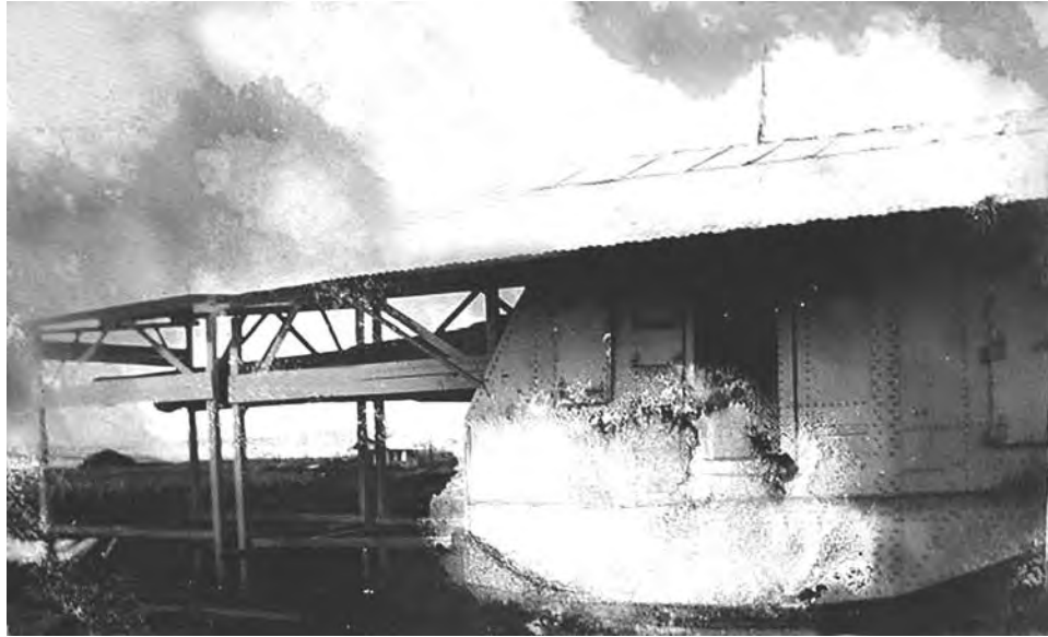
Battery Brodie's No. 1 Turret Mount showing rooftop camouflage structure of corrugated tin and timber that was removed before firing. Photo was damaged during a flood of Monroeton, PA. Varney
