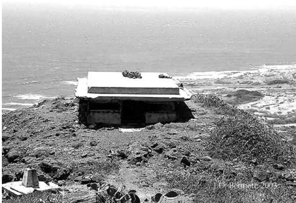
Makapuu Head Fire Control Station "H" (el. 647 feet), a double station built in 1943, served as the B4 of Battery Wilridge. Author, 2001
