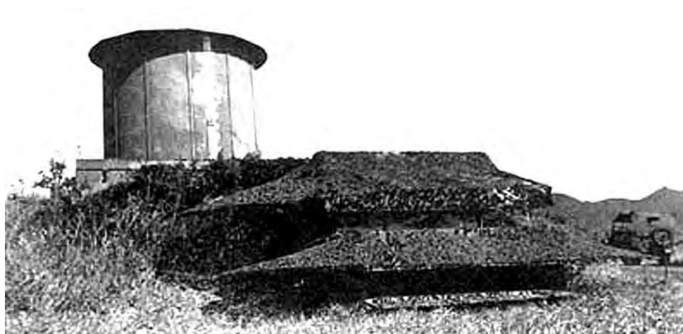
Camouflaged BCS at Battery Wilridge. Note SCR-296A radar antenna disguised to resemble a water tank, and camouflage netting that resembled house rooftops. NARA
