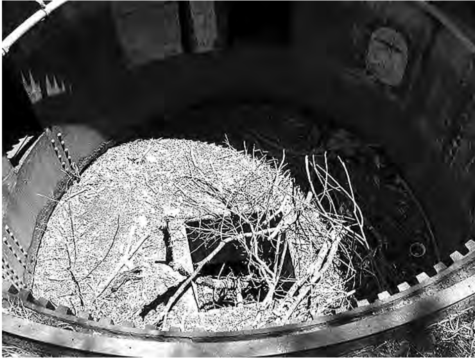
Opening in the floor of Battery Wilridge (Kirkpatrick) Turret No. 1's barbette for electrical, data transmission, and compressed air lines that were routed to the turret mount. Author, 2002
