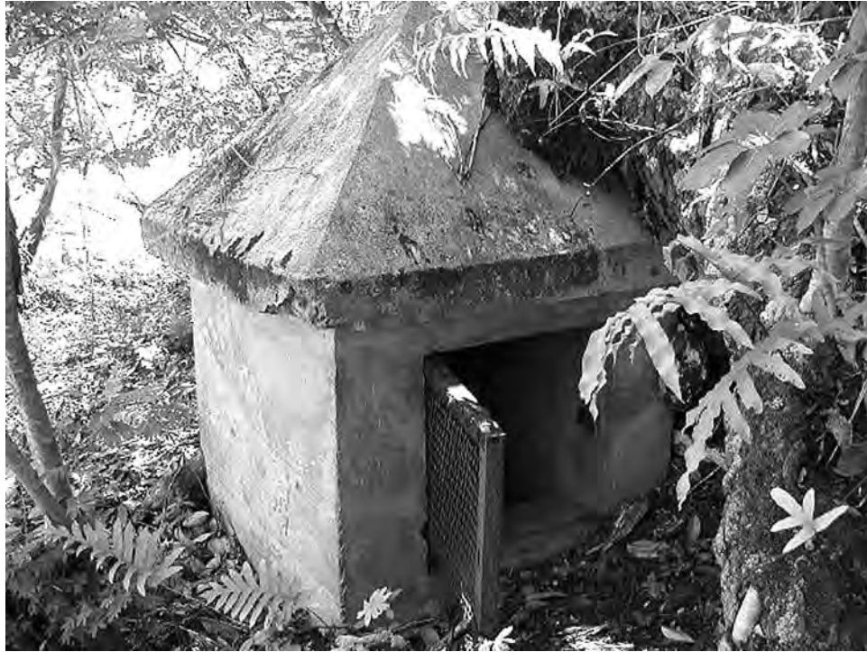
Typical escape housings found atop 8-inch NT battery plotting rooms. This example is at Battery Opaeula (Riggs). Author, 2002
