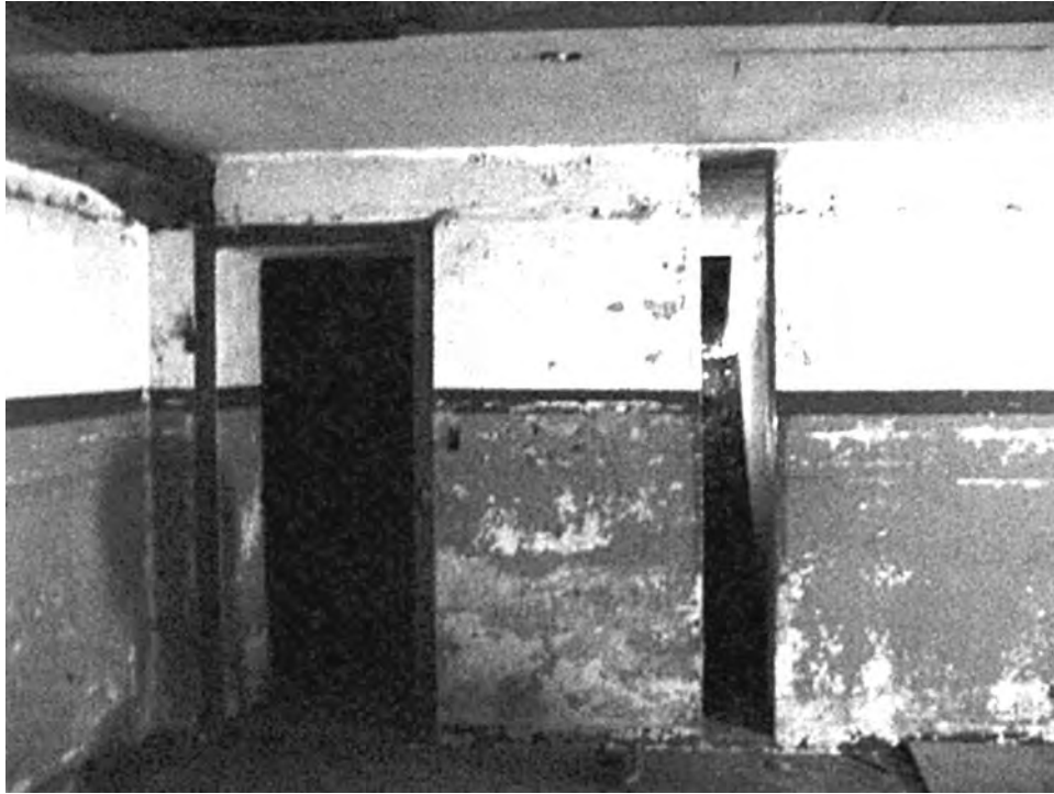
Interior of Plotting Room No. 1 at Battery Opaoula (Riggs). Author, 2002
