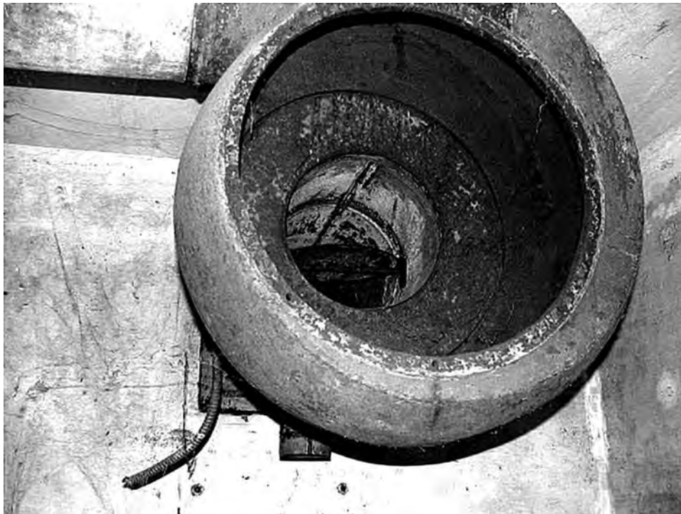
Part of the CWS equipment on the interior wall of Plotting Room No. 1 at Battery Opaoula (Riggs). Author, 2002
