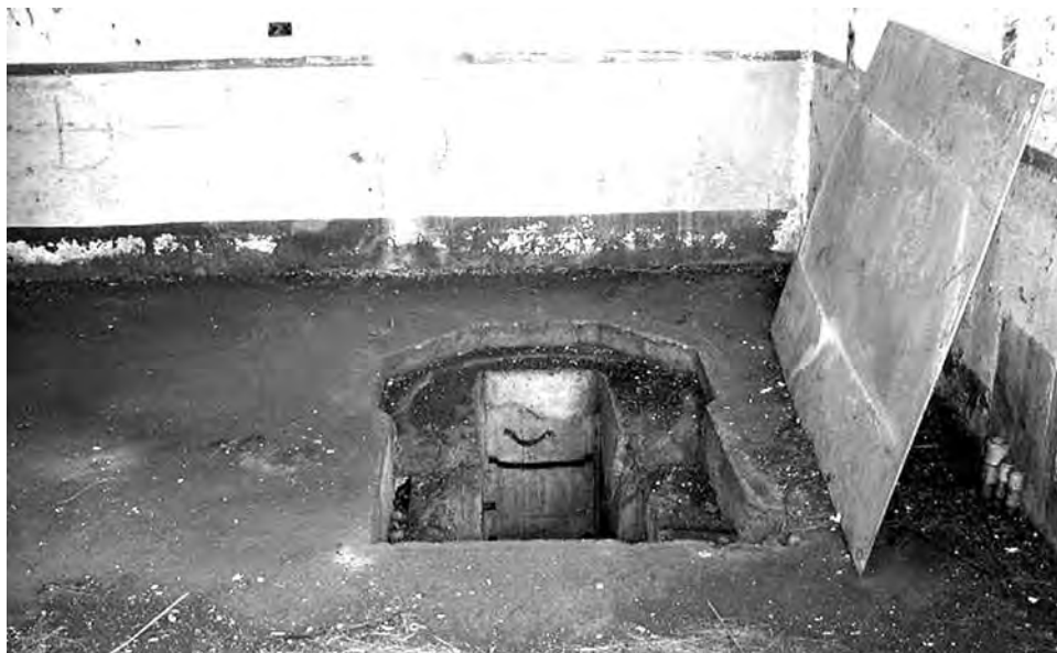
Floor of Brodie's BCS showing manhole to a passageway leading to Mk XX naval computer room. Author, 2002
