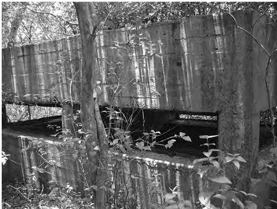
Concrete vent housing, Battery Wilridge (Kirkpatrick) power room. Author, 2002
