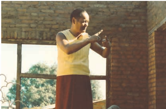
Lama Yeshe supervises building of Kopan Gomba extension, 1976
