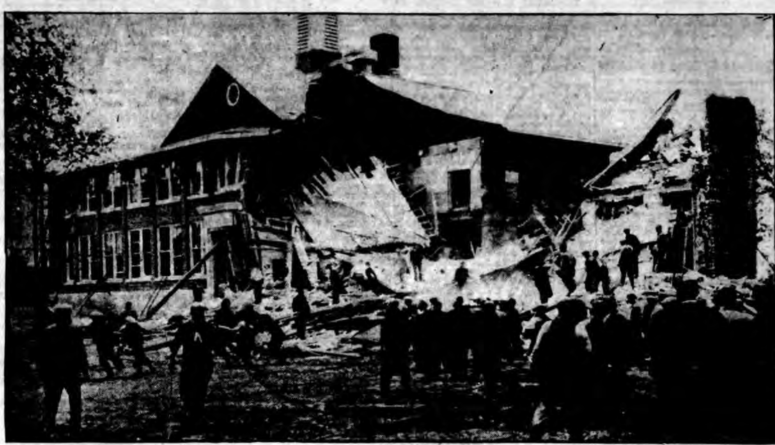
Andrew Kehoe, revenge-maddened farmer, blew up this school at Bath, Mich., killing 36 pupils and five adults. Kehoe planted a large quantity of dynamite in the school basement and by means of an ingenious wiring system leading to his automobile set off the blast. He was one of the victims of his deed.
