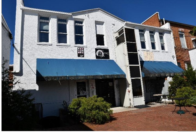
124 Main Street, Rear elevation, looking northwest. (Photo 013).
