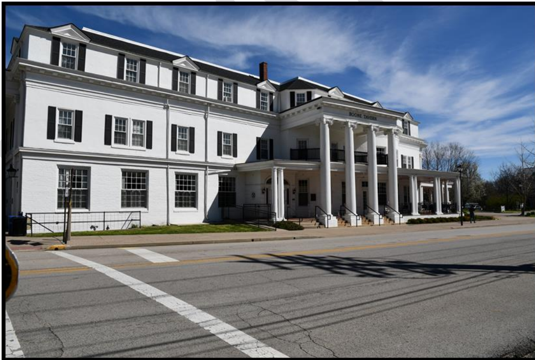
Figure 6. Berea College Square District, Boone Tavern (MAB-12), looking northeast from Prospect Street. (Photo 003).
